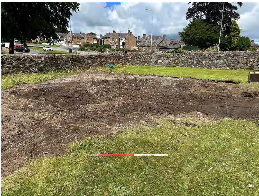
Plate 4: Area monitored after groundworks. View north
