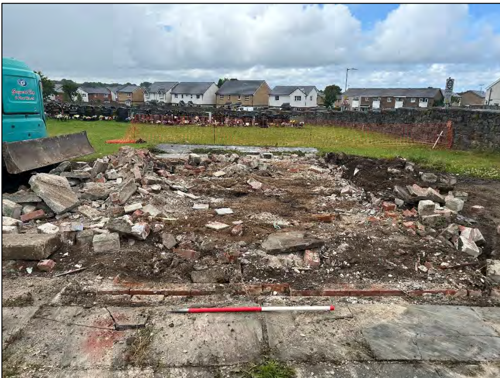
Plate 2: Imprint of building after demolition, view southwest
