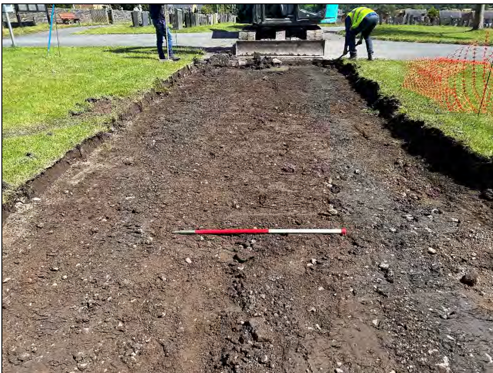
Plate 6: Tarmac Road fully removed. View east south-east
