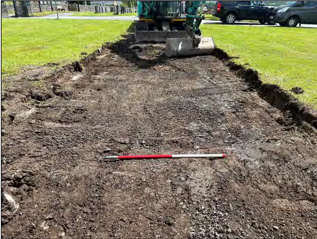
Plate 5: Removal of tarmacked road. View east southeast
