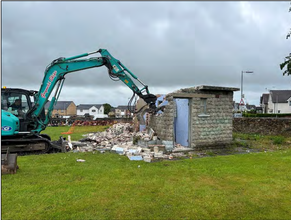
Plate 1: Working shot of public conveniences demolition. View west
