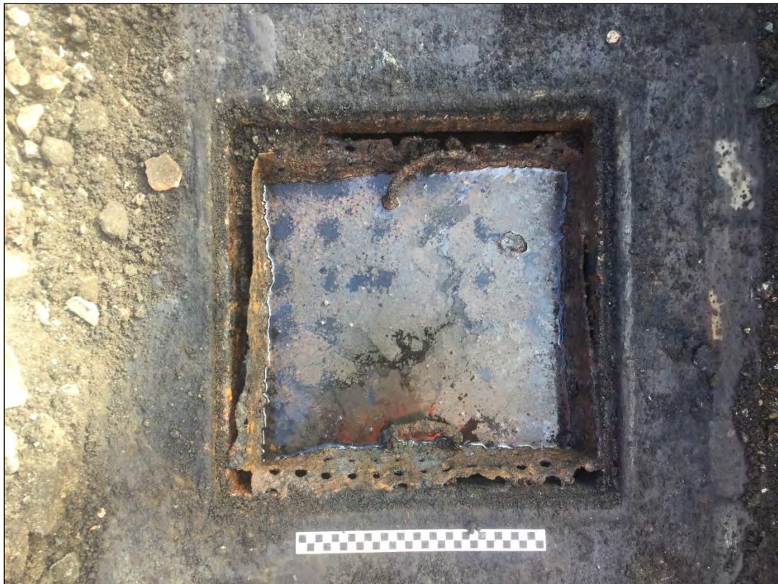
Plate 13. Interior of the sump, with filter still in place.
