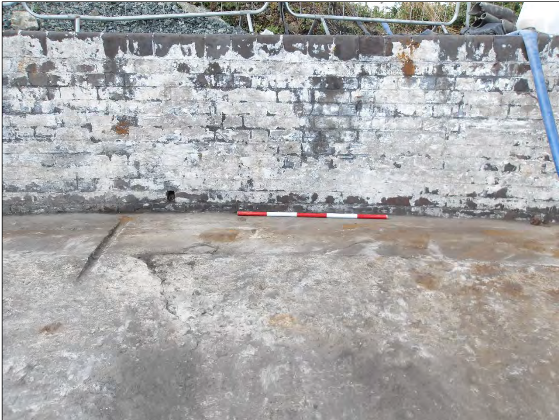
Plate 31. Turntable wall [304], showing white render.
