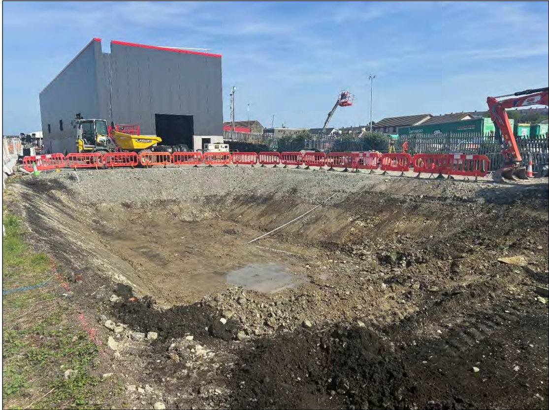
Plate 21. Excavation of the attenuation tank, looking north.
