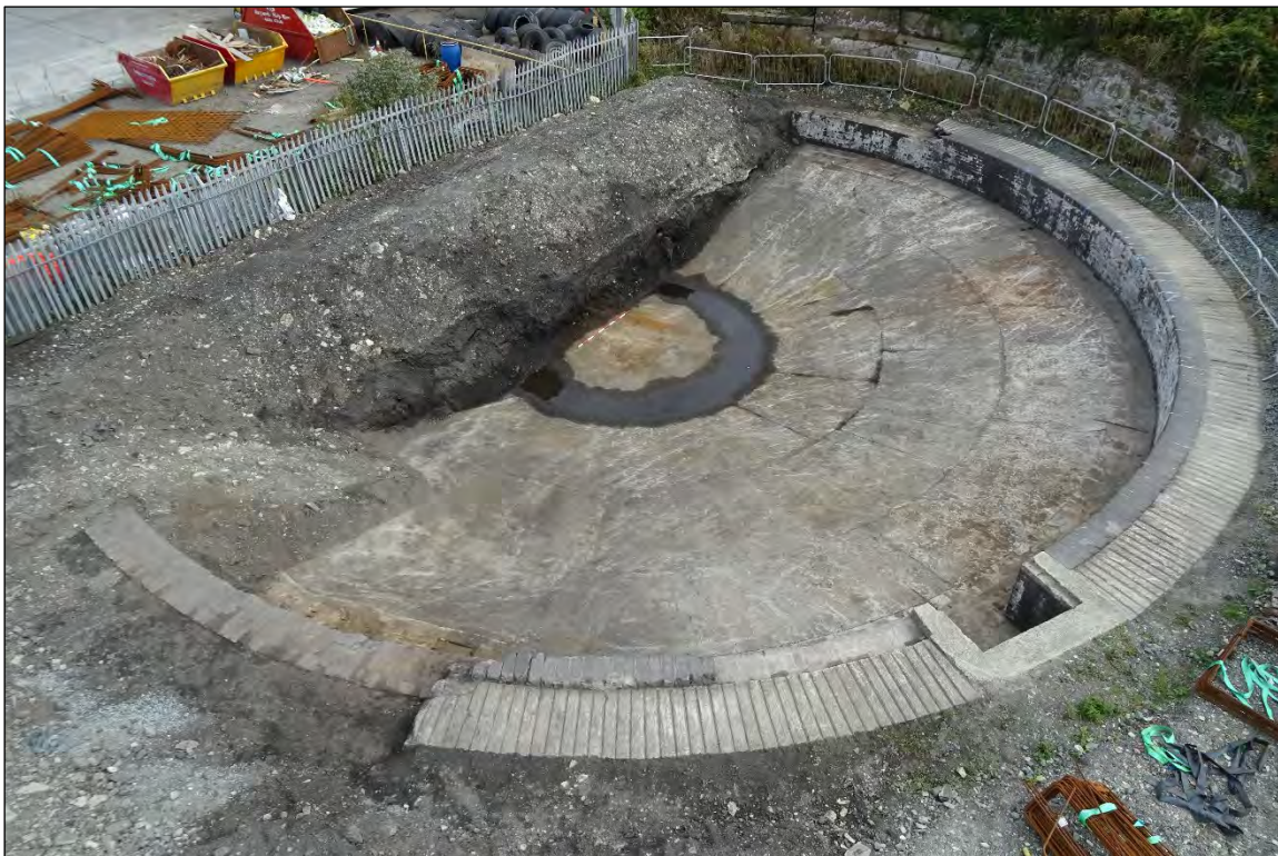
Plate 38. Turntable G3 after removal of the infill.
