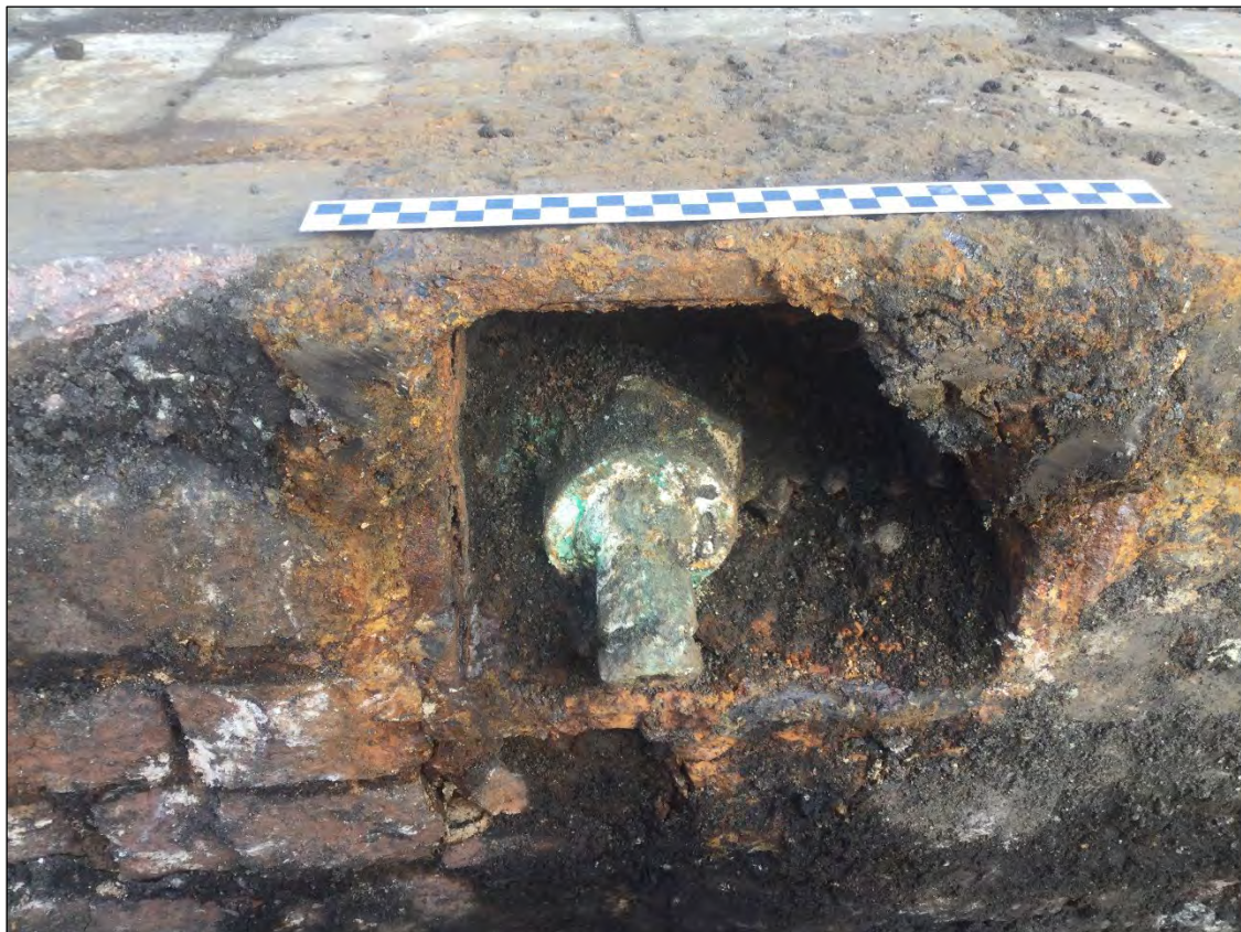
Plate 11. One of the hose fitting set either side of the walls of the inspection pit.
