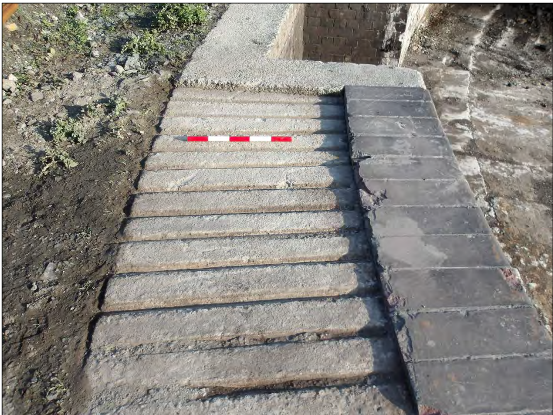
Plate 32. Ribbed walkway around outer edge of the turntable.
