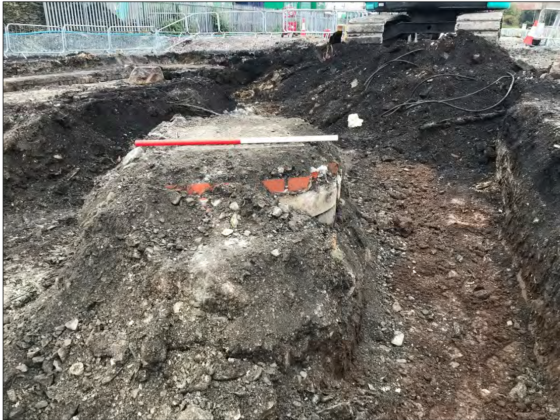
Plate 17. Modern concrete brick manhole at southern end of Area 1.
