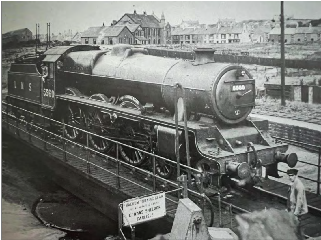
Plate 41. Historic photo of turntable G3 in operation.
