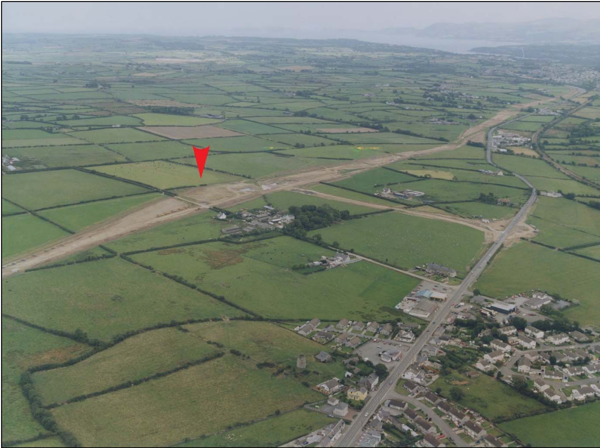
Plate 1: Aerial photo by Gwilym Davies during construction of A55 in 1999, arrow shows proposed development area (WM2540/5/14, Anglesey Archives)
