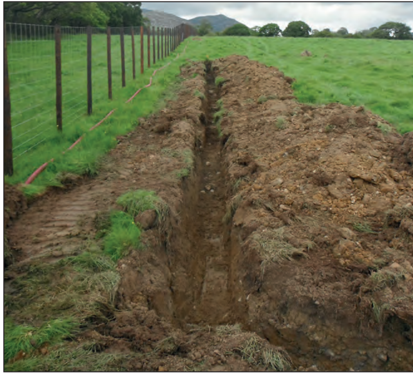
General working shot, cabling trench
