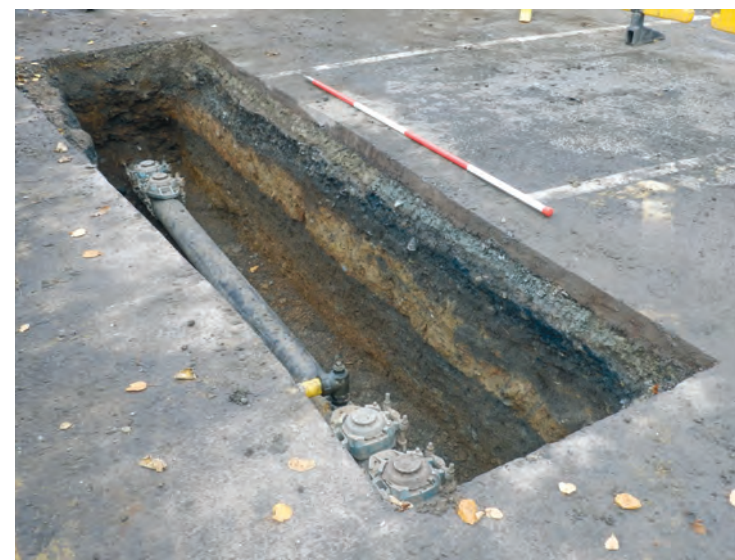
South-west facing section of Trench 4 (scale 2m)
