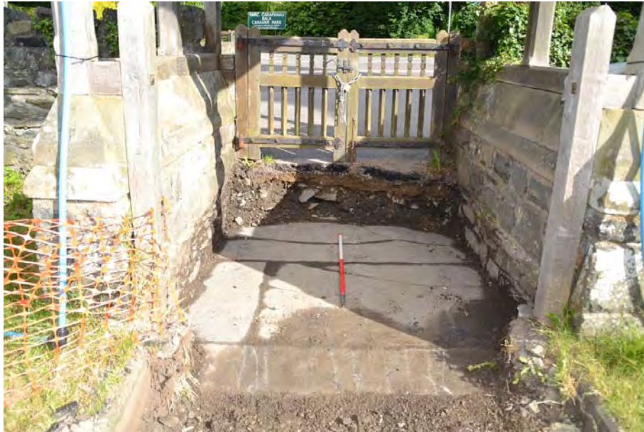
Fig. 20 Slate flag stone and beam footing of cemetery lychgate. Photo CPAT 3881-0005.
