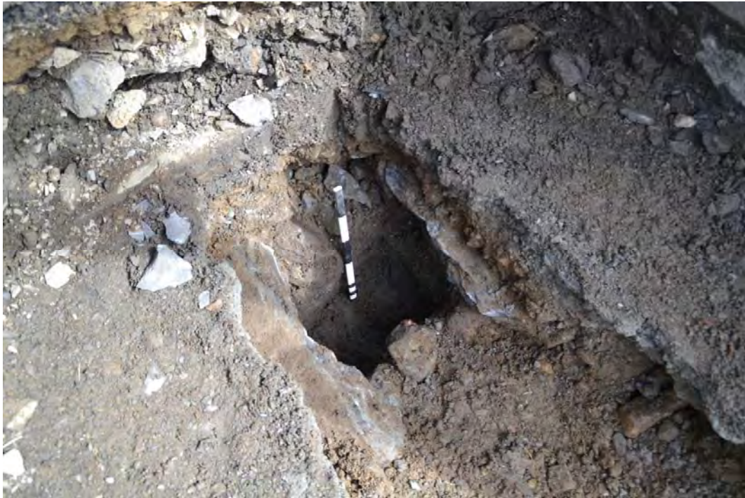
Fig. 26 Lime-bonded stone wall footing (64); the earlier line of the churchyard wall. Photo CPAT 3880-0011.
