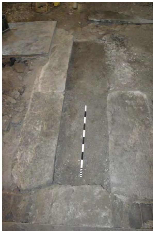
Fig. 7 Stone slab floor foundation at the entrance to the nave with one grave slab removed (and the photo scale introduced) to reveal the rubble make-up, viewed from the north. Photo CPAT 3805-0012
