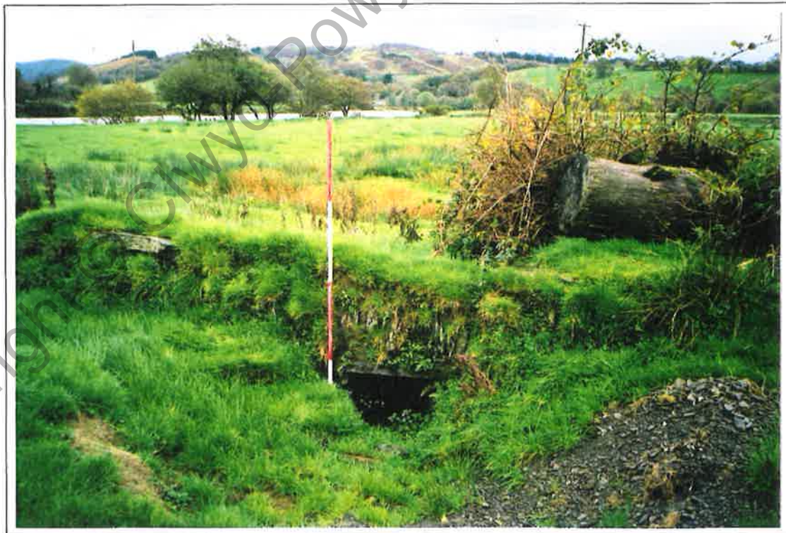
Plate 8 Corris Railway culvert (PRN 36888). Photo CPAT 1113.10
