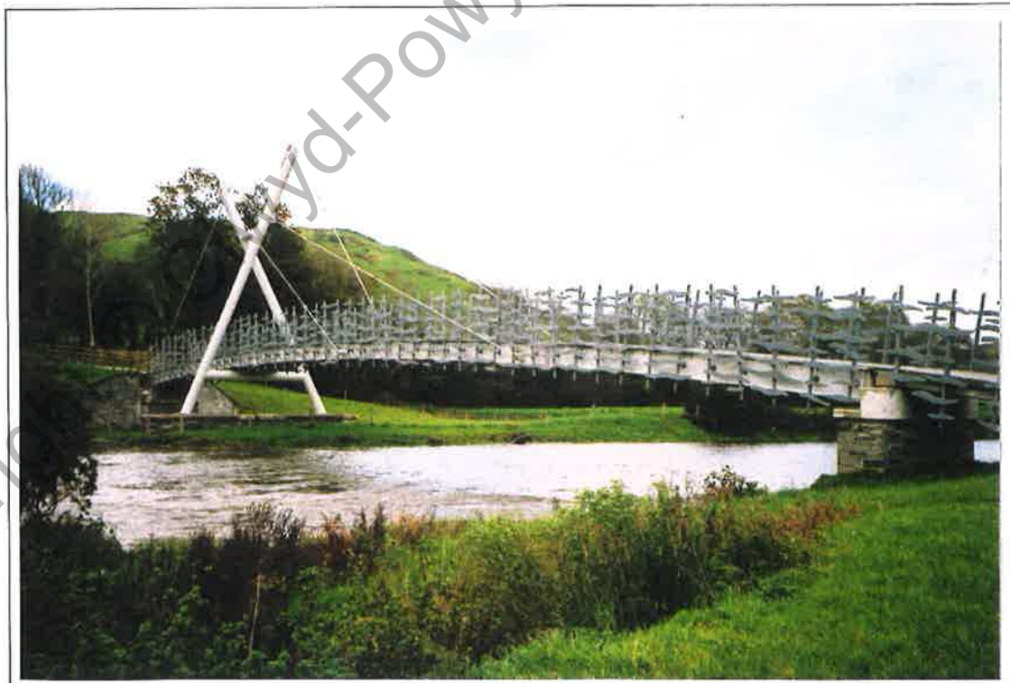
Plate 10 Site of Corris Railway Dyfi Bridge (PRN 36894). Photo CPAT 1113.11
