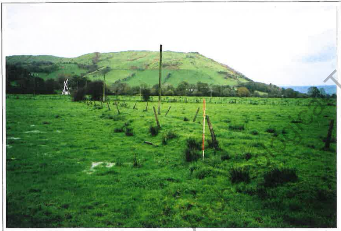
Plate 7 Corris Railway embankment (PRN 36886). Photo CPAT 1113.9
