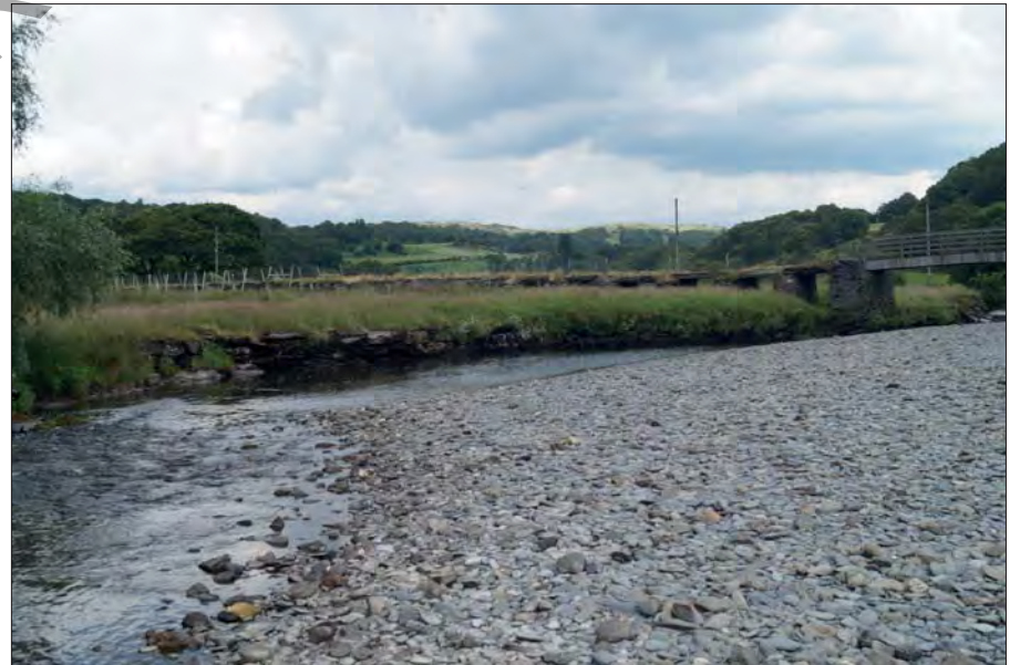
Plate 4. River Revetment Associated with Chwarel-y-Fedw Quarry Bridge and Causeway
