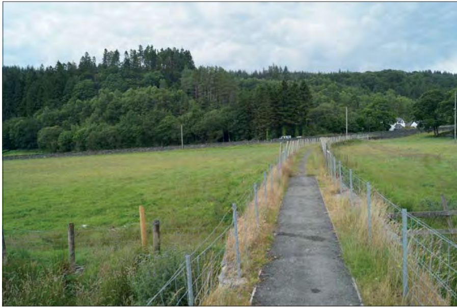
Plate 13. Chwarel-y-Fedw Quarry Bridge and Causeway
