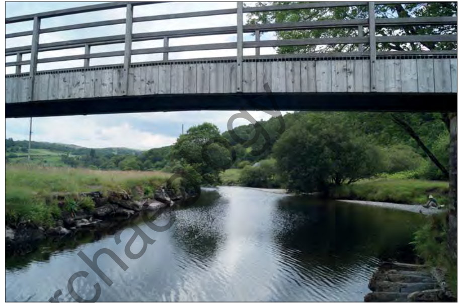
Plate 6. Chwarel-y-Fedw Quarry Bridge
