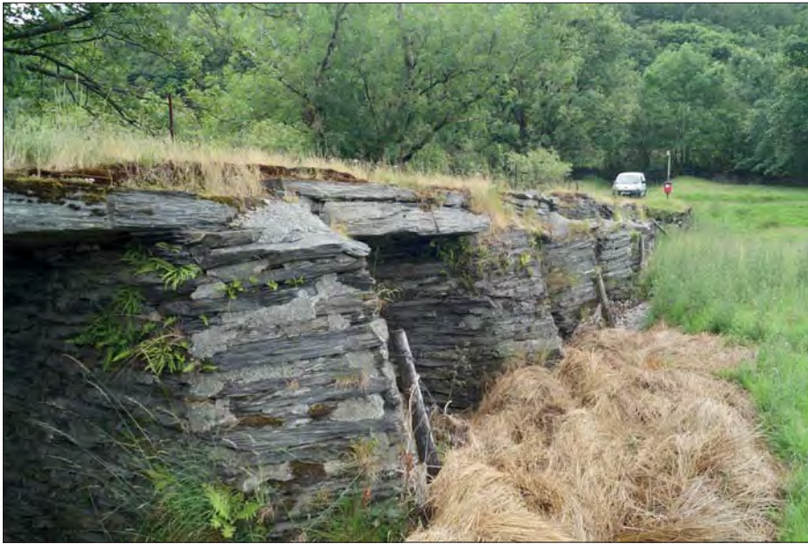
Plate 9. Chwarel-y-Fedw Quarry Bridge Stone Pier
