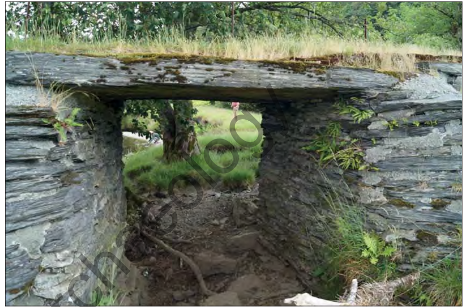
Plate 10. Chwarel-y-Fedw Quarry Bridge Stone Pier and Slab
