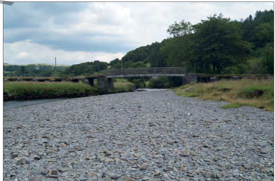
Plate 8. Shingle Bank Adjacent to Chwarel-y-Fedw Quarry Bridge and Causeway
