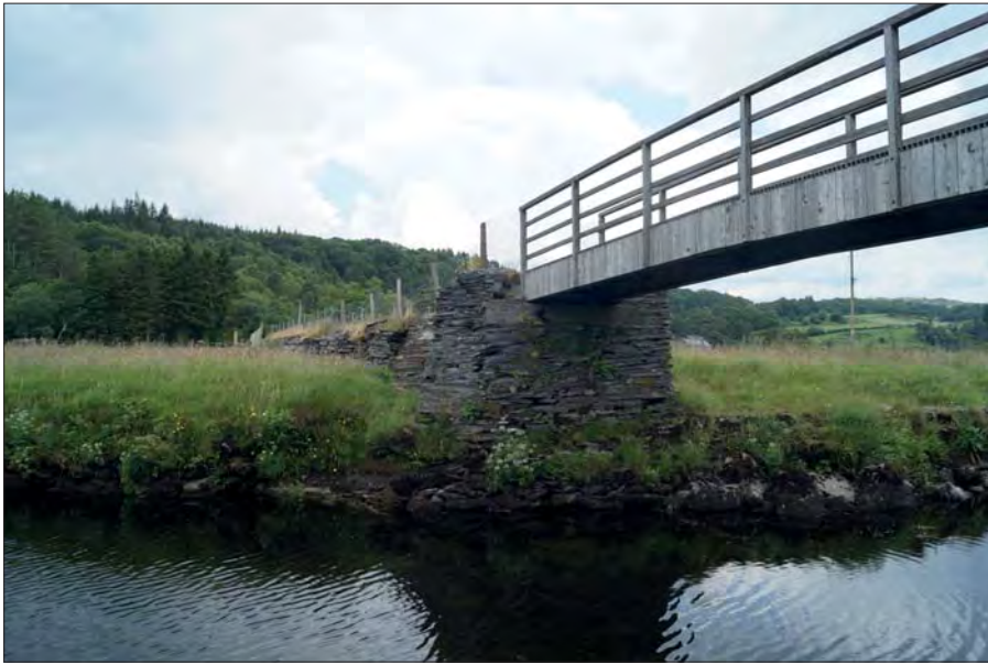
Plate 5. Chwarel-y-Fedw Quarry Bridge
