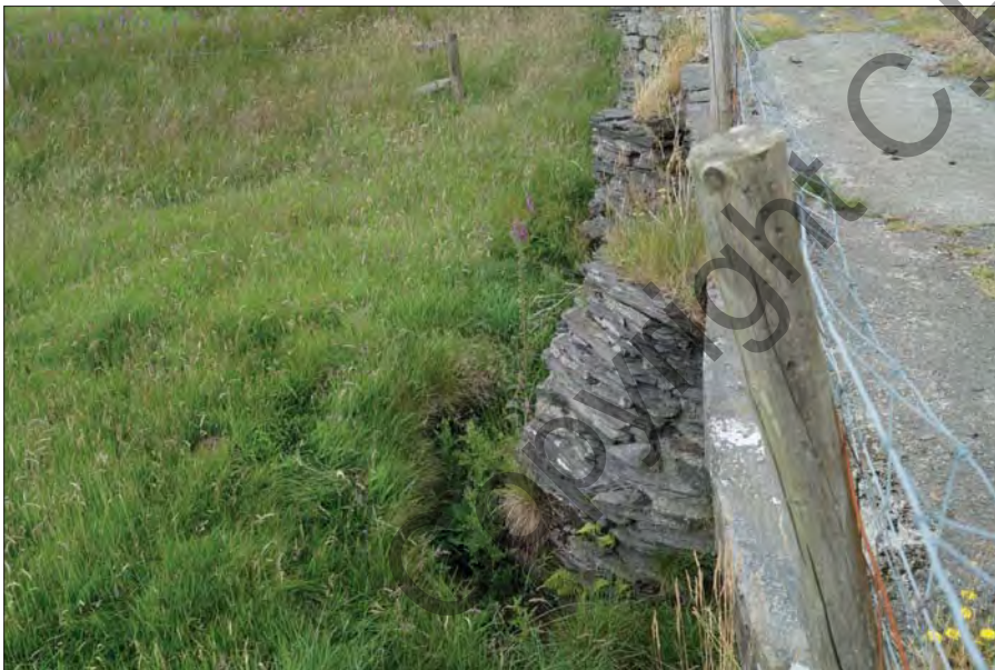
Plate 11. Chwarel-y-Fedw Quarry Bridge and Causeway Stone Pier
