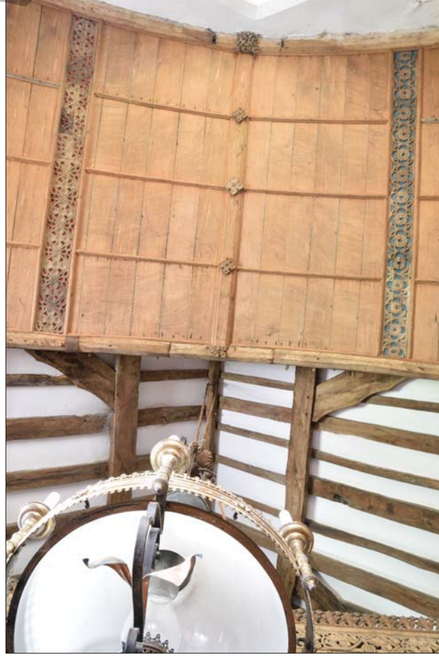
Plate 45. Barrel Vaulted Ceiling in Chancel
