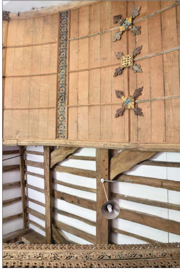
Plate 46. Barrel Vaulted Ceiling in Chancel
