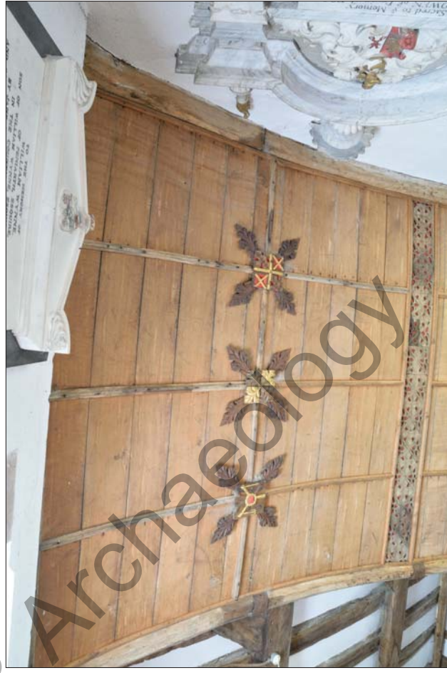
Plate 46. Barrel Vaulted Ceiling in Chancel
