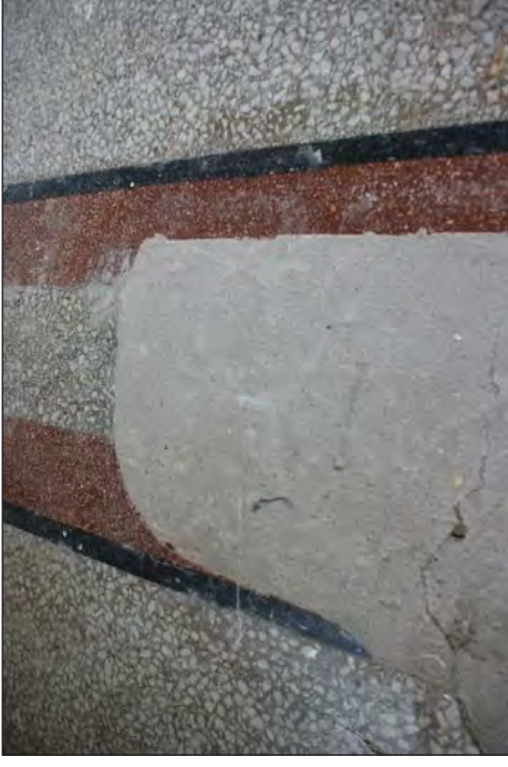
Plate 45. Partial Survival of Original Floor Detailed Shot Showing Concrete Base With Thin Stone Floor Tiles
