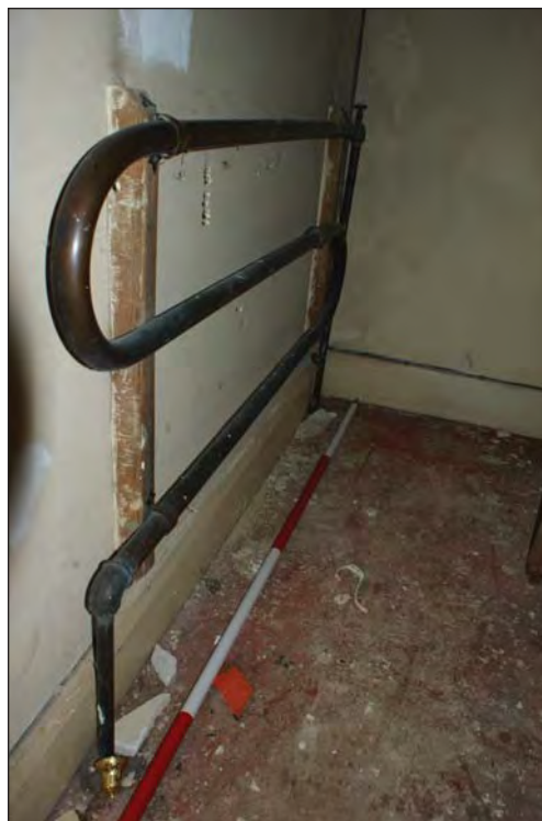
Plate 29. Second Floor Linen Closet With Original Copper Pipe Radiator
