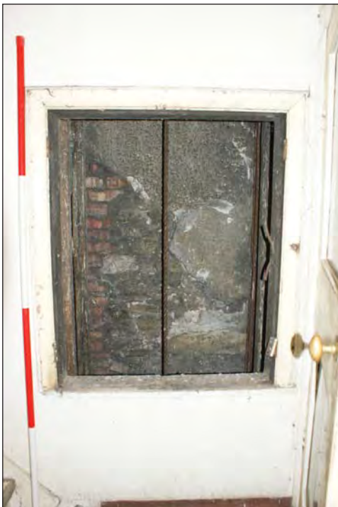
Plate 49. Opening for Dumbwaiter at Ground Floor Level
