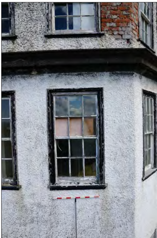
Plate 19. The 1919 Extension Western Elevation Showing Window Details (1m Scale)
