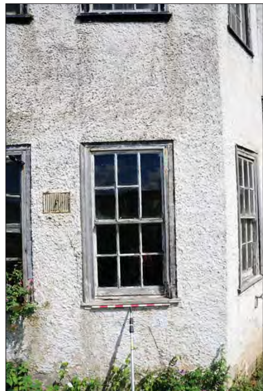
Plate 20. The 1919 Extension Western Elevation Showing Window Details (1m Scale)
