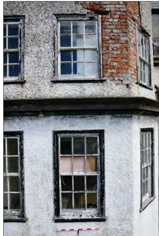
Plate 16. The 1919 Extension Window Detail and Exposed Brickwork In Western Elevation
