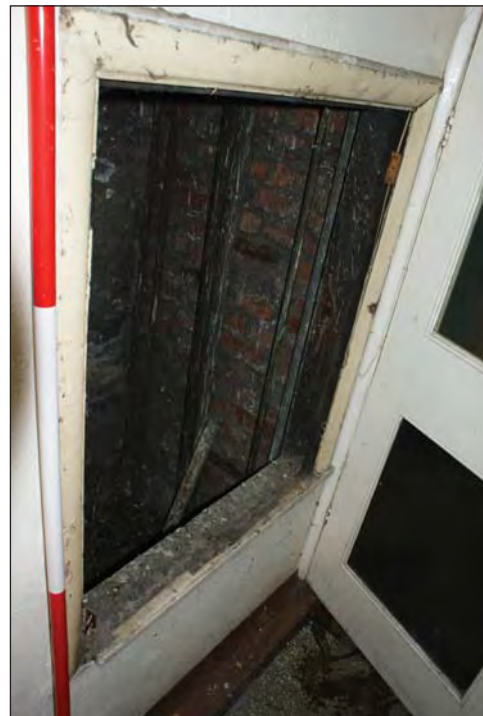
Plate 50. Opening for Dumbwaiter at Ground Floor Level
