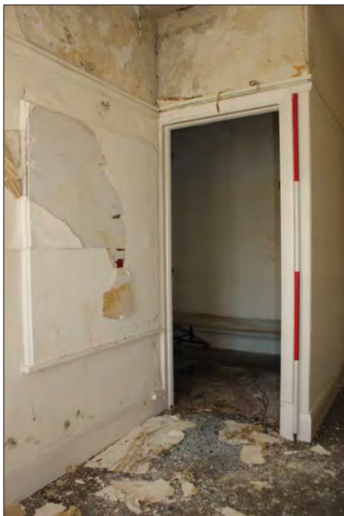
Plate 30. Second Floor Cupboard At Top of Stairway. Blocked Dumb Waiter Can Be Seen to the Left
