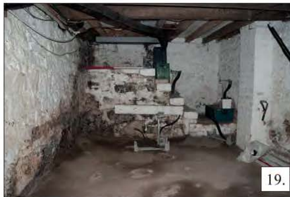
Plate 16. Victorian Entrance Added Between Cellar Rooms 1 & 2. Brick Used Around Entrance - Walls are Stone Built
