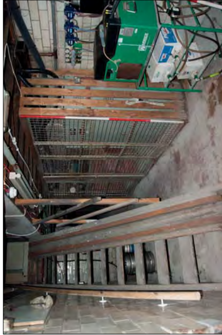
Plate 31. Cellar Room 3 Showing Steps And Barrel Slide.
