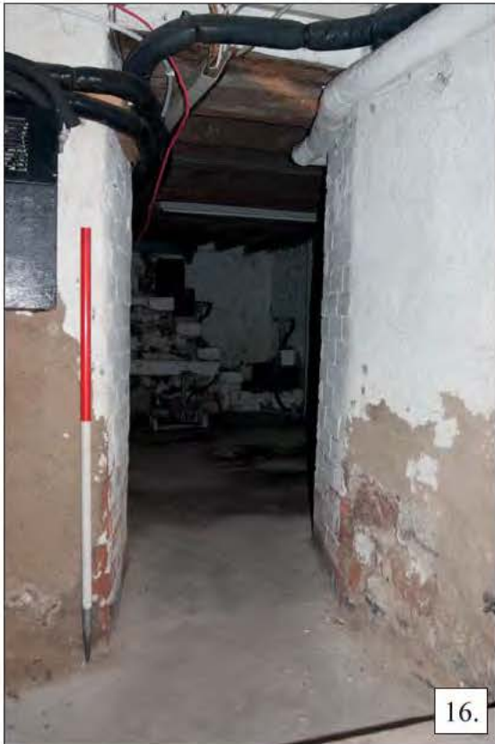
Plate 16. Victorian Entrance Added Between Cellar Rooms 1 & 2. Brick Used Around Entrance - Walls are Stone Built
