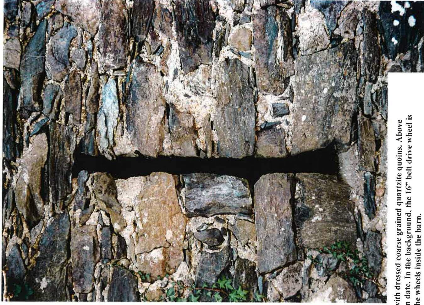
Plate 11 right : Sample ventilation slit in the 1818 barn. Slits measure 0.97m high by 0.44m wide by 0.57m deep
