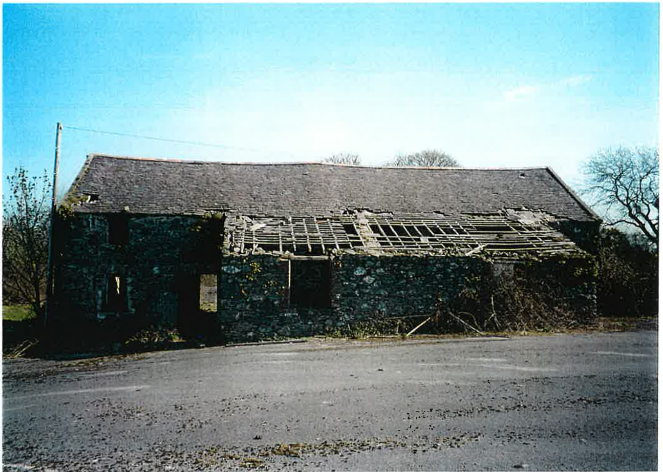
Plate 8 Barn B2, viewed from the southwest across the yard / car parking area. The two-compartment addition to the southwest side was built in 1923 as a root store ( left ) and an engine house ( right ).
