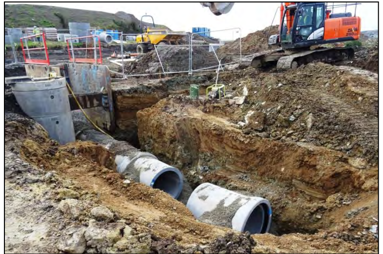
Plates 33 & 34 above: Deep excavations for ain sewer, March 2017
