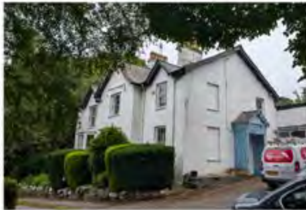
View of the primary elevation and main entrance door to the side
