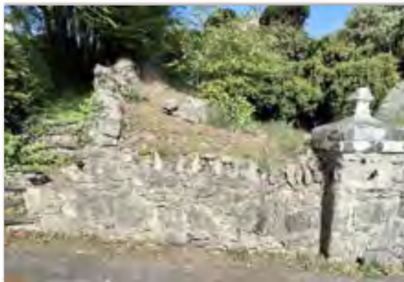
View of the section of retaining wall in question
