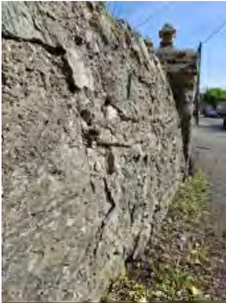
Side-on view of the wall looking East
