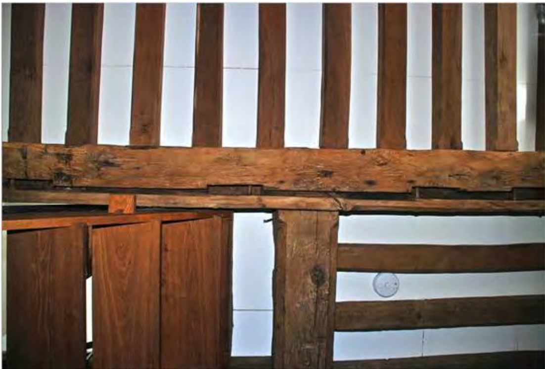
Plate 14: Evidence for the post and plank partition
