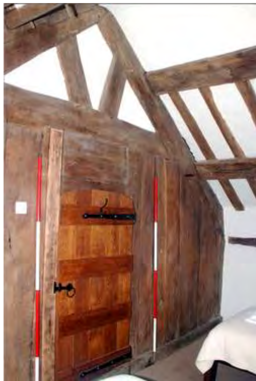
Plate 20: Plank and post partition looking west
