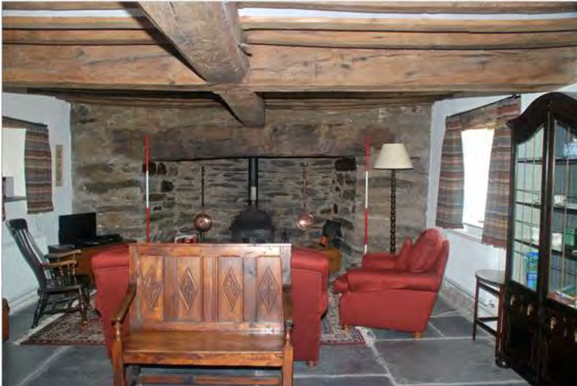
Plate 12: Bressumer and main longitudinal beam
