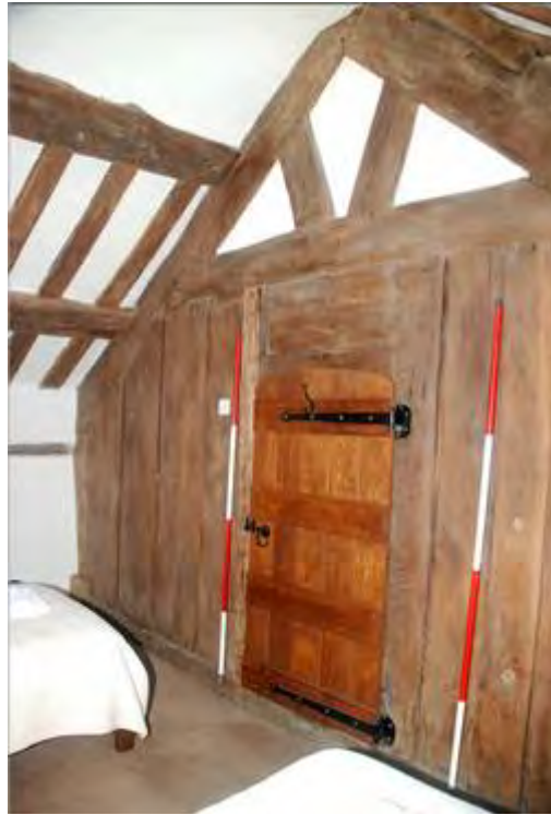
Plate 21: Plank and post partition looking south
