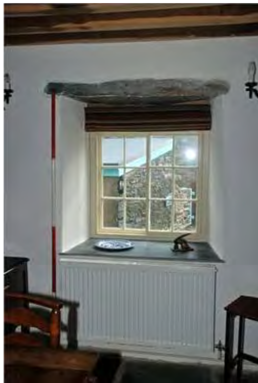
Plate 10: South eastern window showing slate lintel
