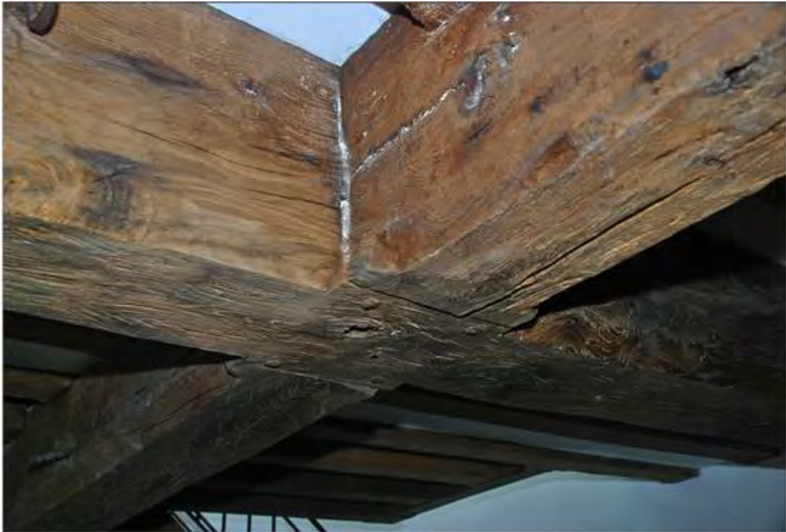
Plate 13: Detail of chamfers and stop at intersection between the longitudinal and lateral beams.
