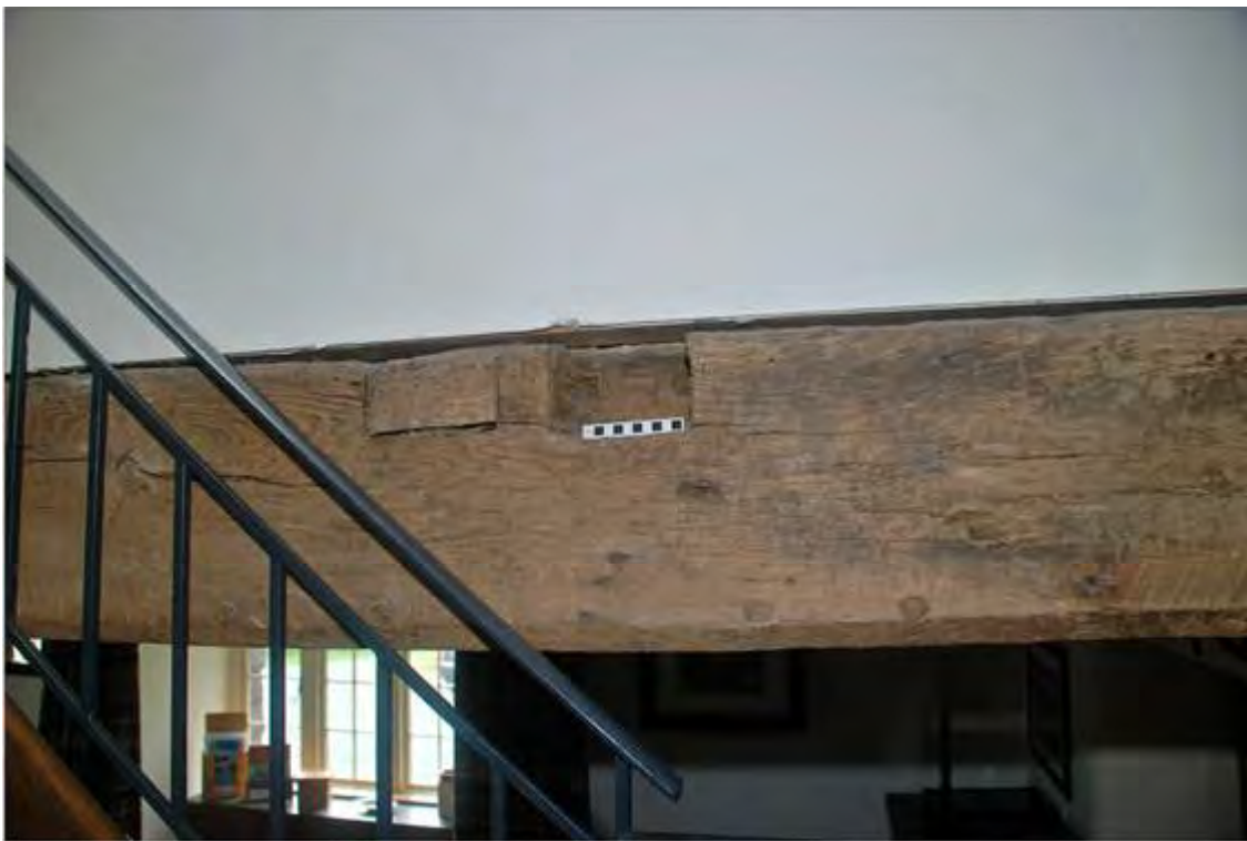
Plate 16: Mortise for an original joist.
