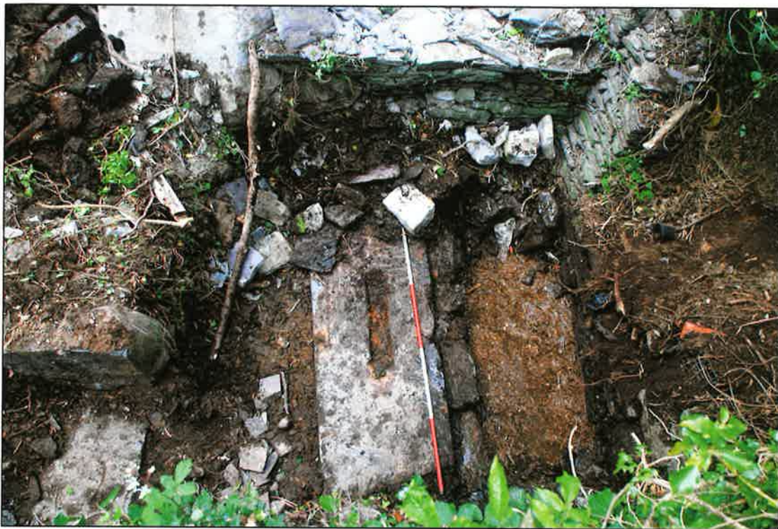
Plate 27: The slate slab for the eastern mounting of the water wheel
