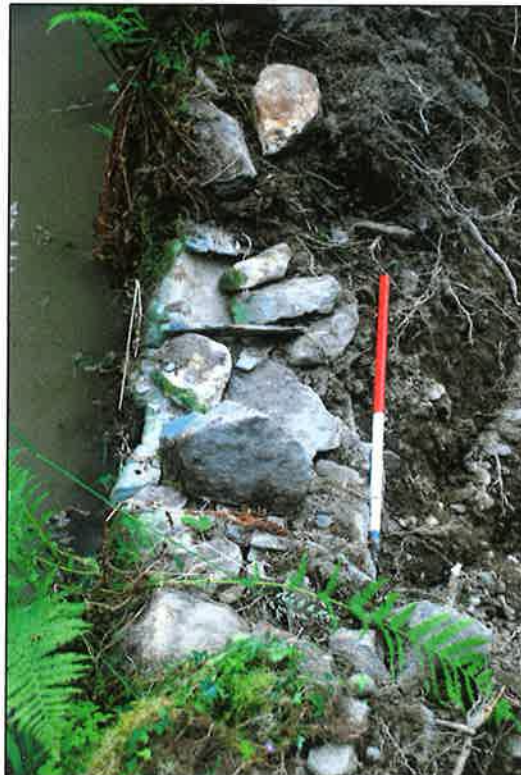
Plate 16: Top of the dam, partly excavated showing the structure of the wall
