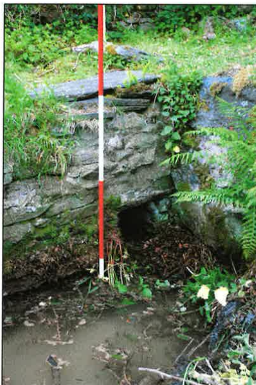
Plate 13: Detail of the leat opening in the south west corner of the mill pond
