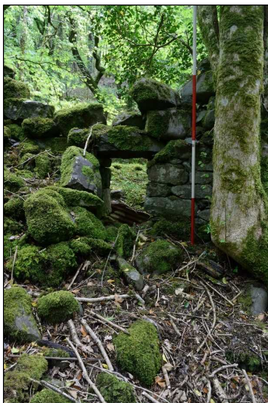
Plate 15: Slot for the drive shaft of the waterwheel, looking south
