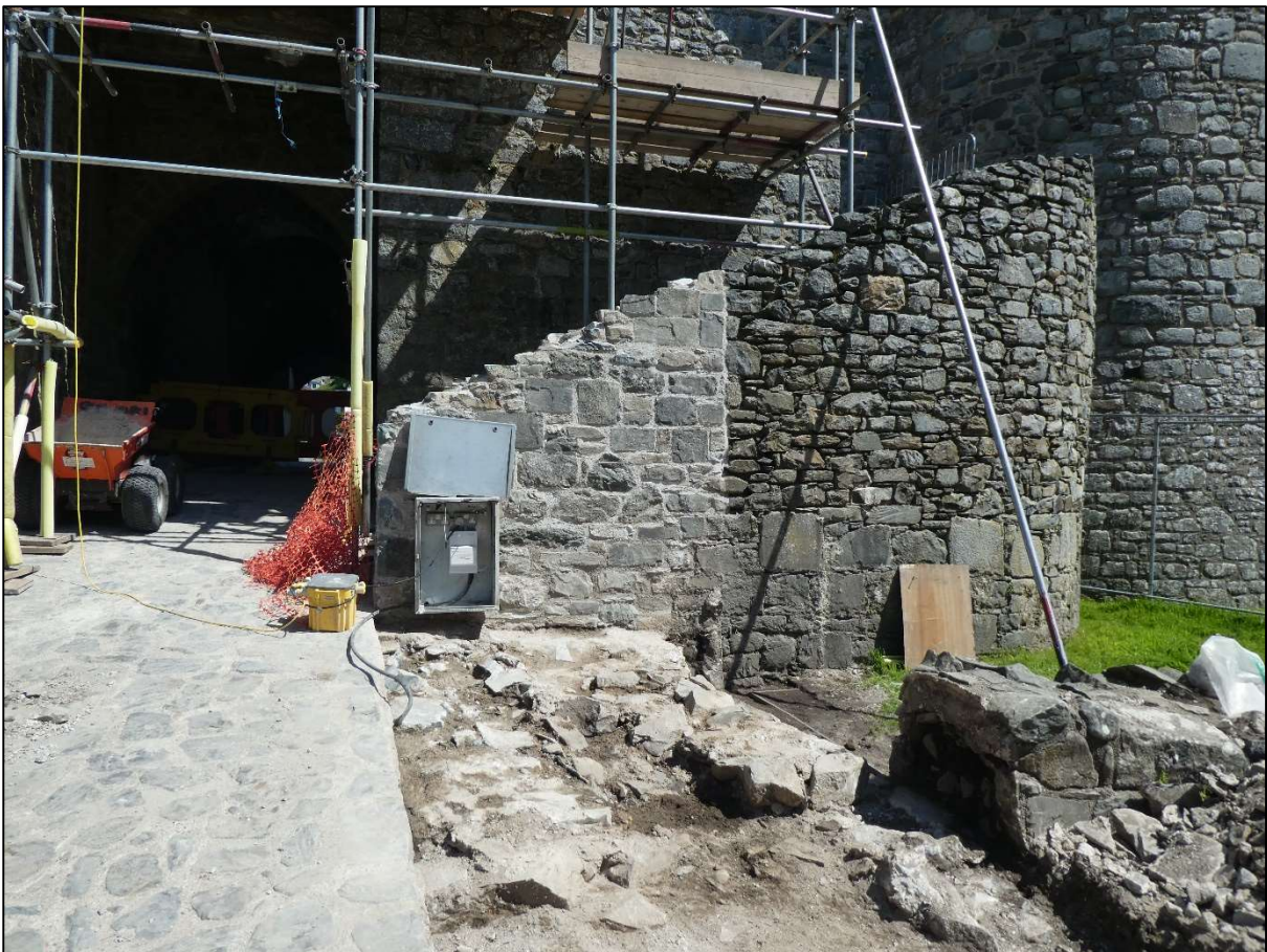
Plate 6: Possible wall below the stairs
