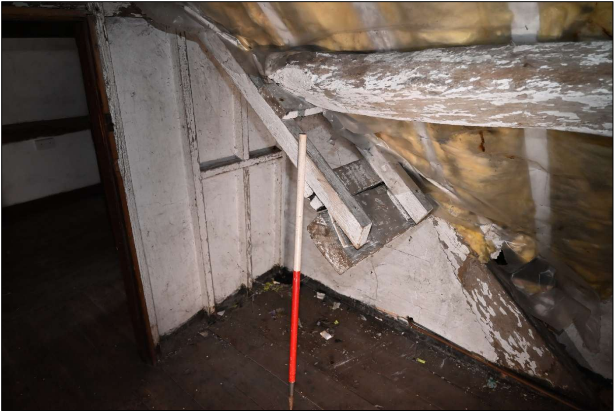
Plate 117: Relationship between the purlin of Attic 4 and the roof structure of Bedroom 4
