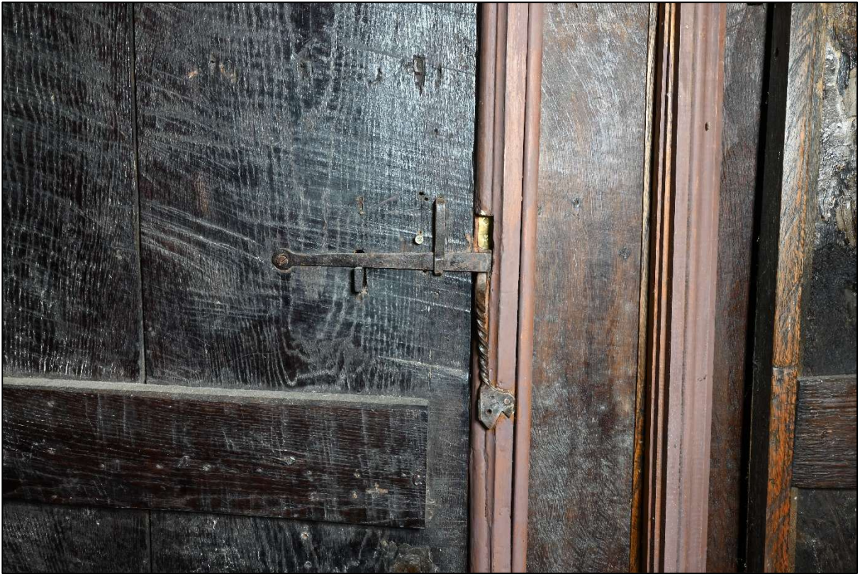
Plate 91: Latch on the eastern door of Bedroom 1
