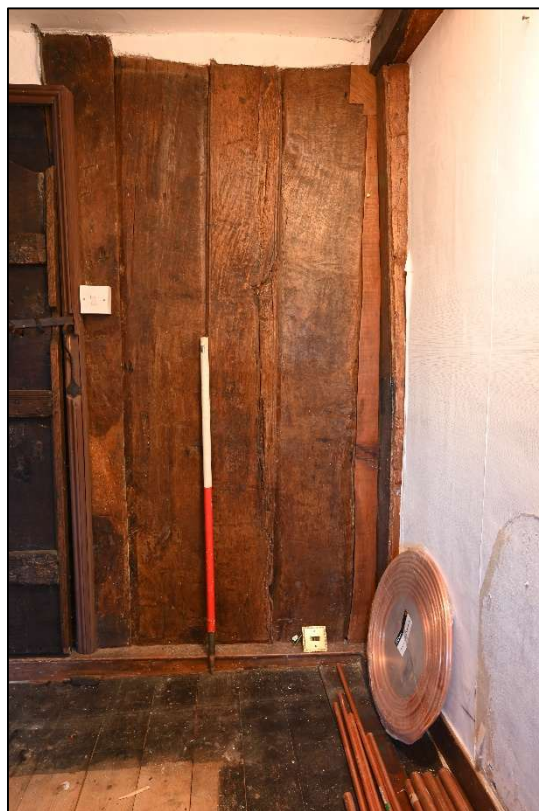
Plate 86: Detail of the plank and muntin partition in Bedroom 1
