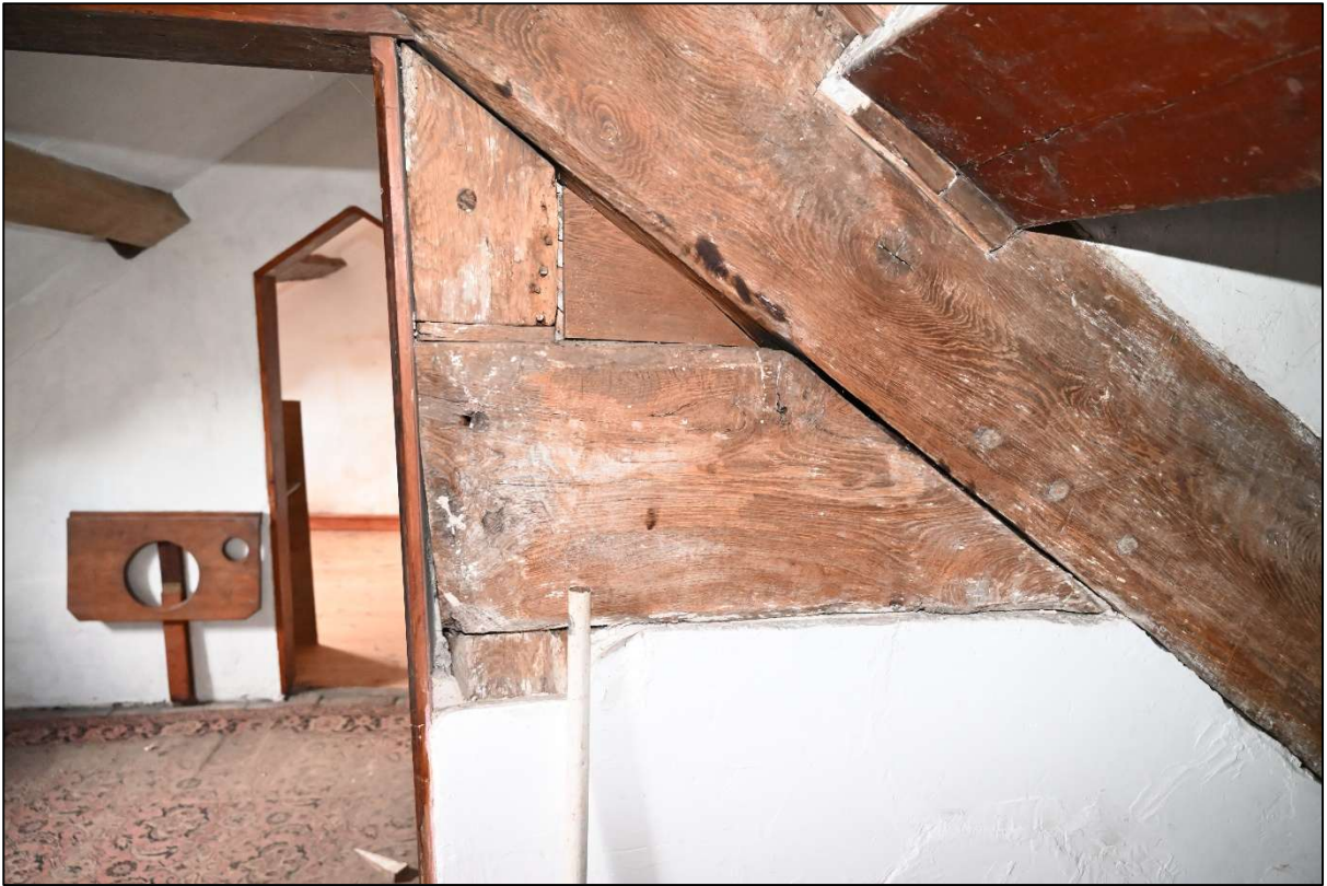
Plate 125: Detail of the truncated collar on Truss 2
