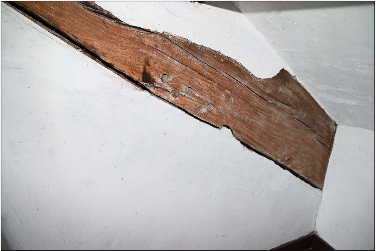
Plate 121: Burn mark on Truss 1
