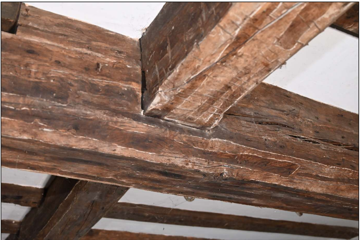
Plate 36: Chamfer and stop on the ceiling beams of the Hall
