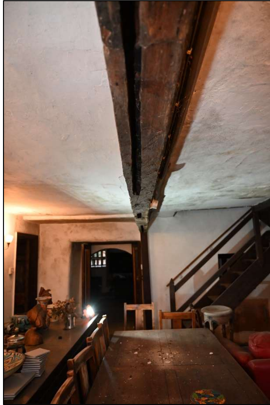
Plate 57: Head rail of the partition in the Dining Room
