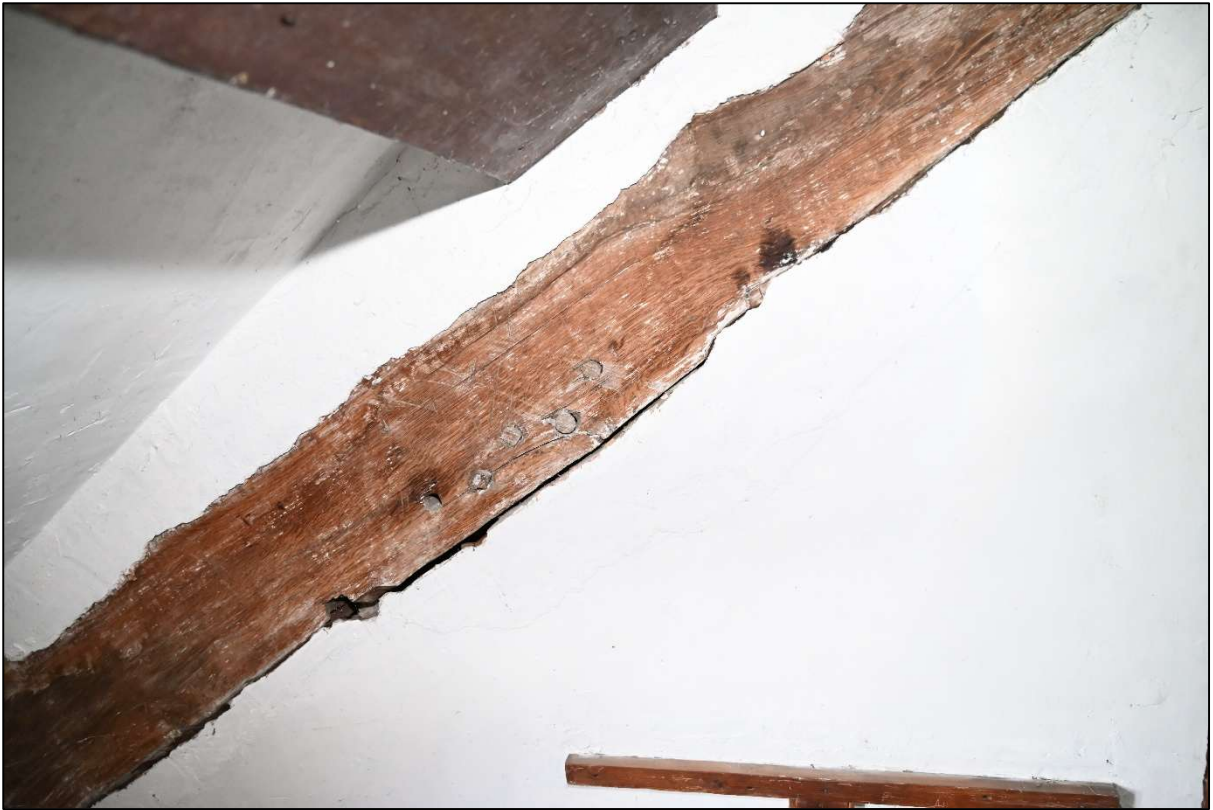
Plate 123: Burn mark on Truss 1
