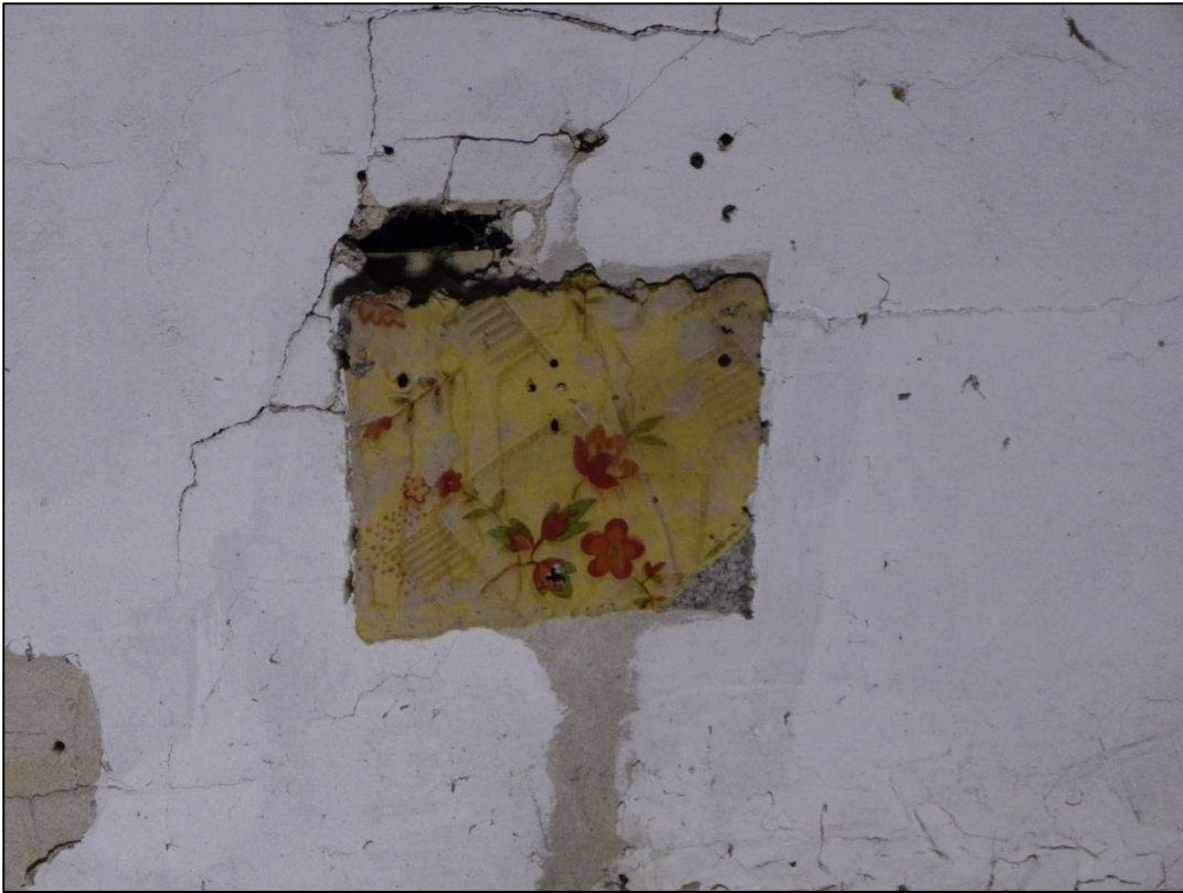
Plate 139: Old wall paper behind an electrical fitting
