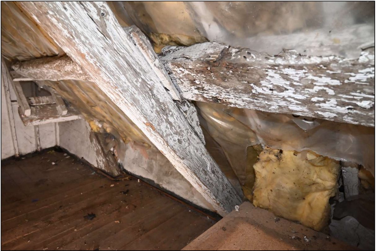
Plate 115: Relationship between the blade of Truss 5 and its purlin
