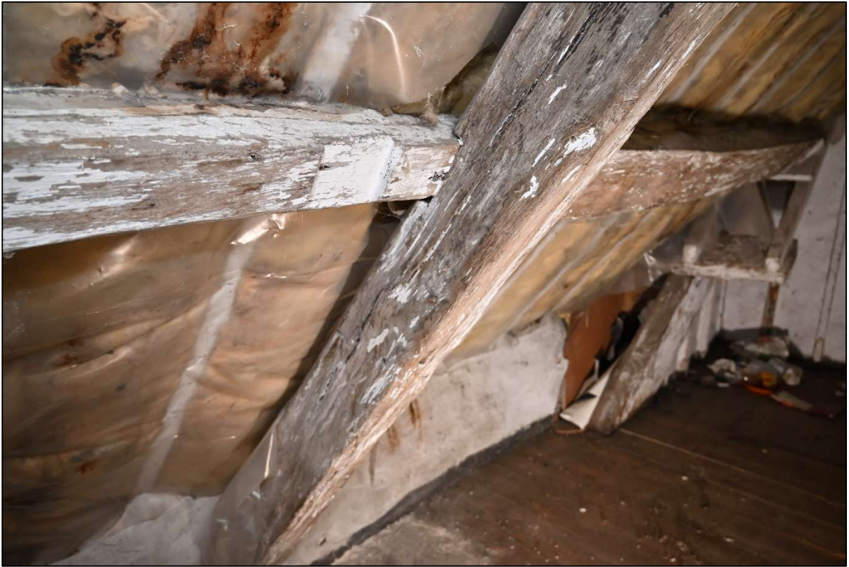
Plate 119: Relationship between the southern purlin and Truss 5
