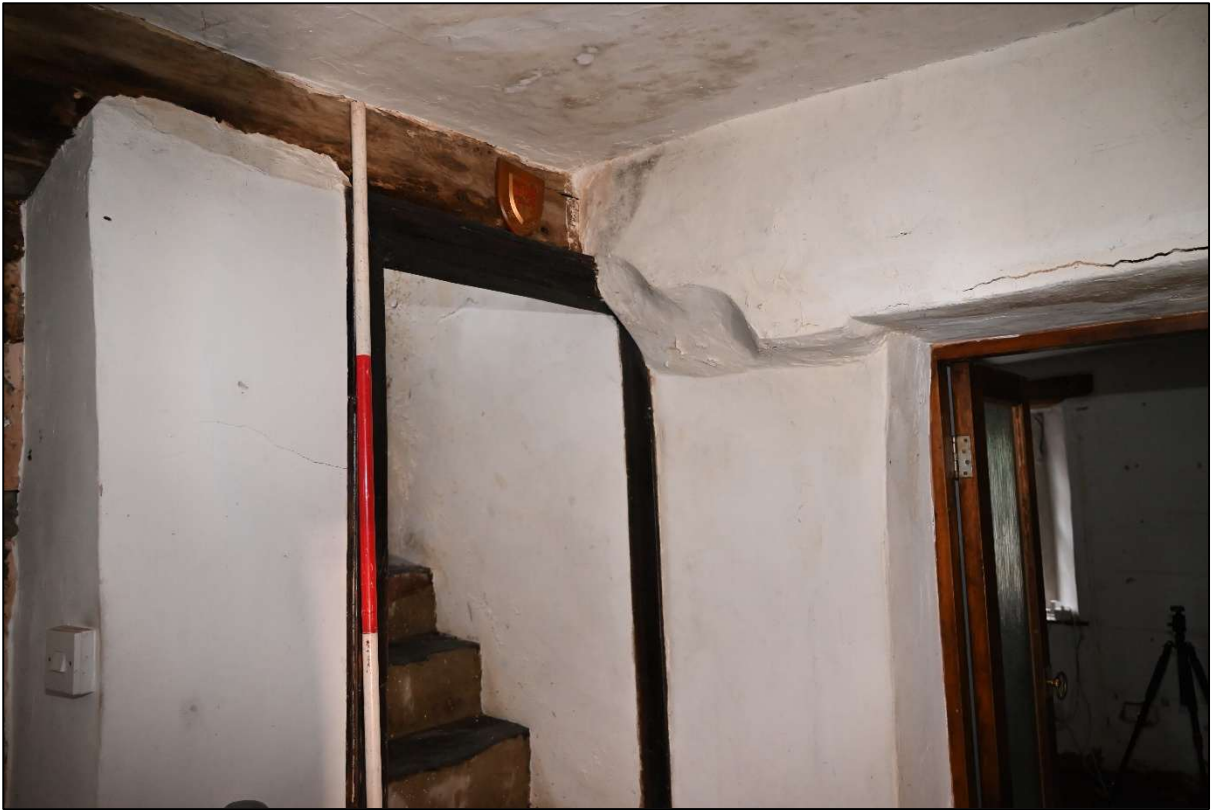
Plate 49: Lintel over the intramural stairs
