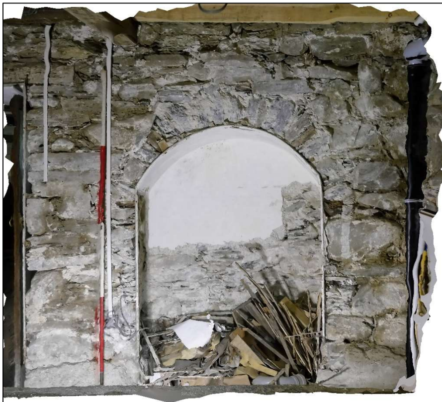
Plate 132: Recess in The Study after the removal of the plaster
