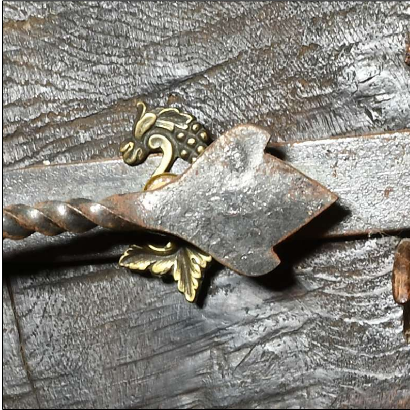
Plate 89: Detail of the latch handle on the western door of Bedroom 1
