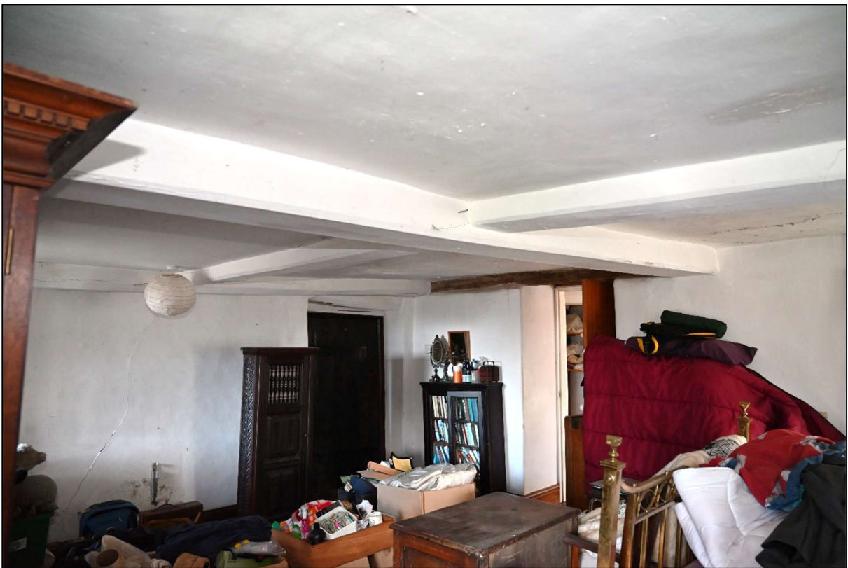
Plate 102: Ceiling beams in Bedroom 3
