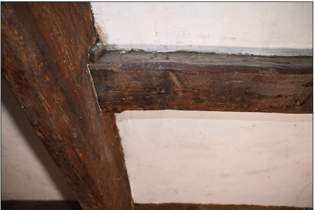
Plate 110: Detail of the relationship between Truss 4 and one of its purlins
