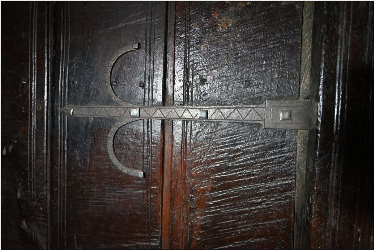
Plate 73: Hinge on the western door
