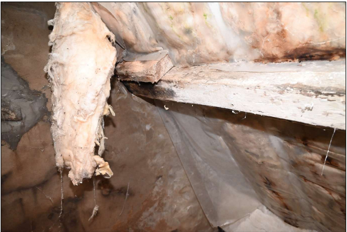
Plate 116: Overlap on the purlin for Truss 5
