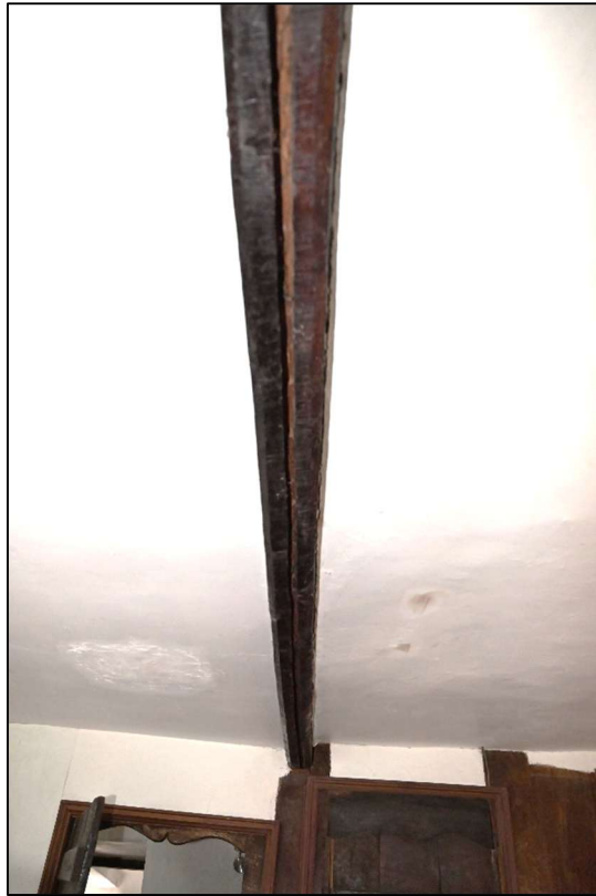
Plate 95: Slot for a partition crossing Bedroom 1
