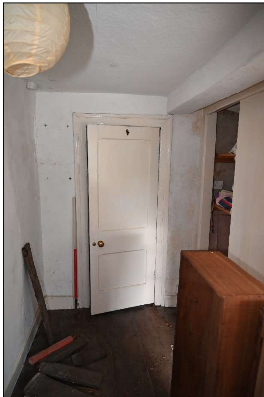
Plate 95: Slot for a partition crossing Bedroom 1
