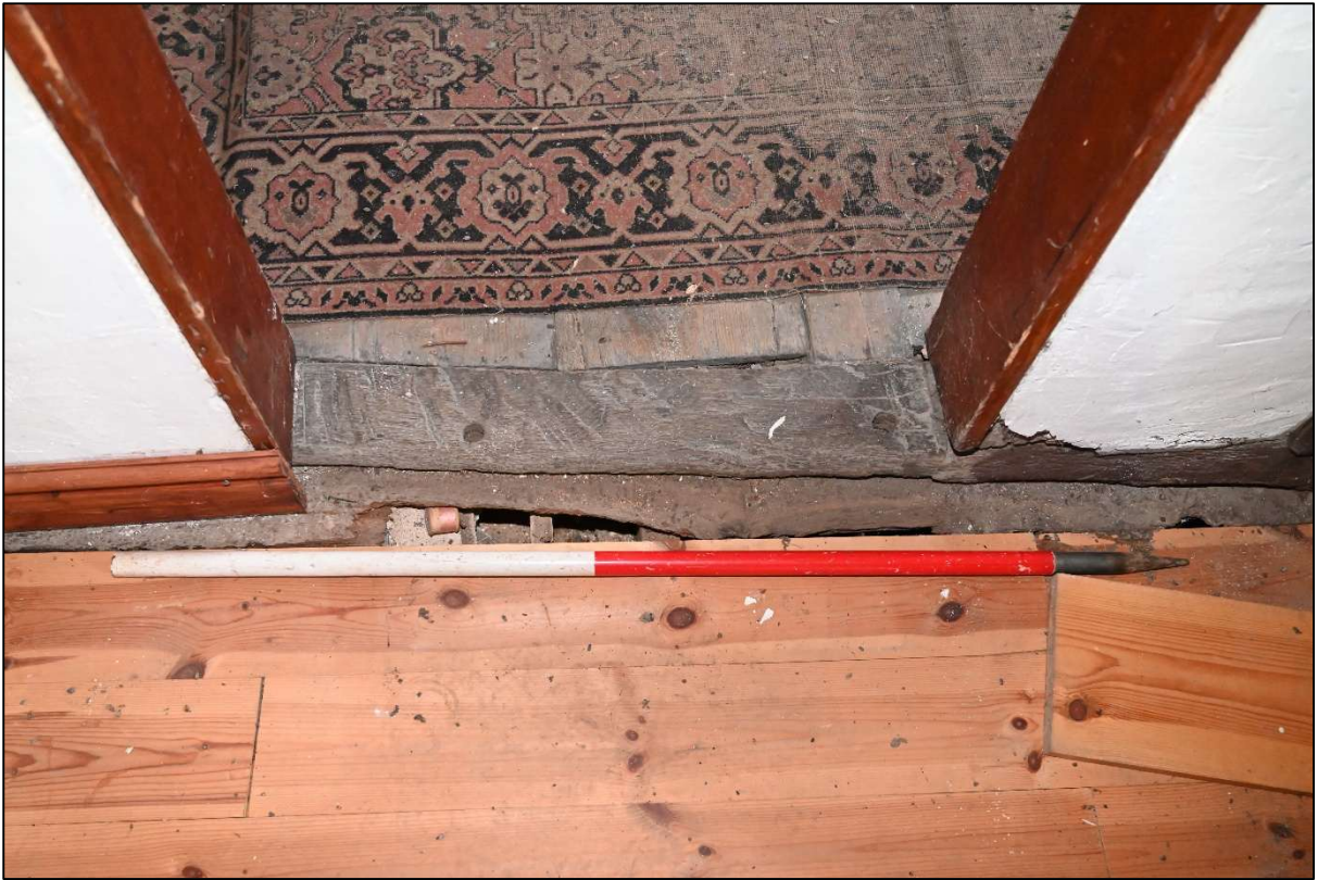
Plate 139: Tie-beam showing in the door between Attics 2 and 3
