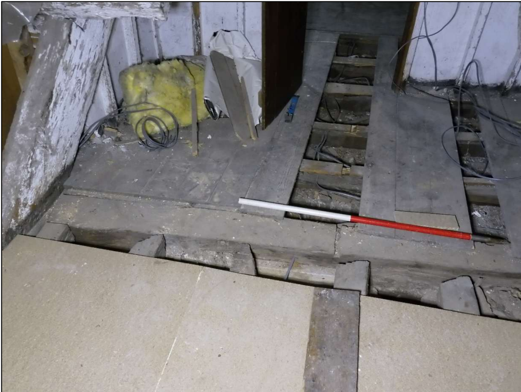
Plate 137: Beams below the floorboards of Attic 4
