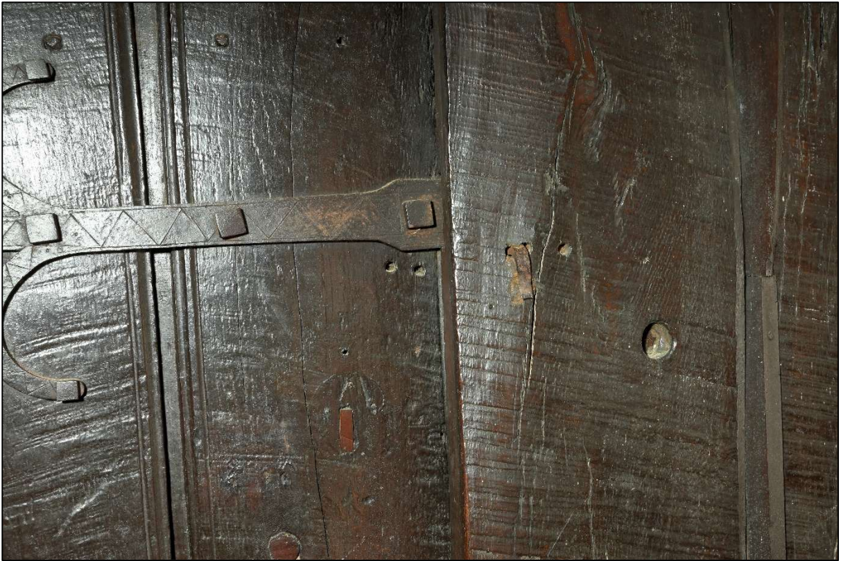
Plate 79: Blocked holes and metal fittings on the eastern door
