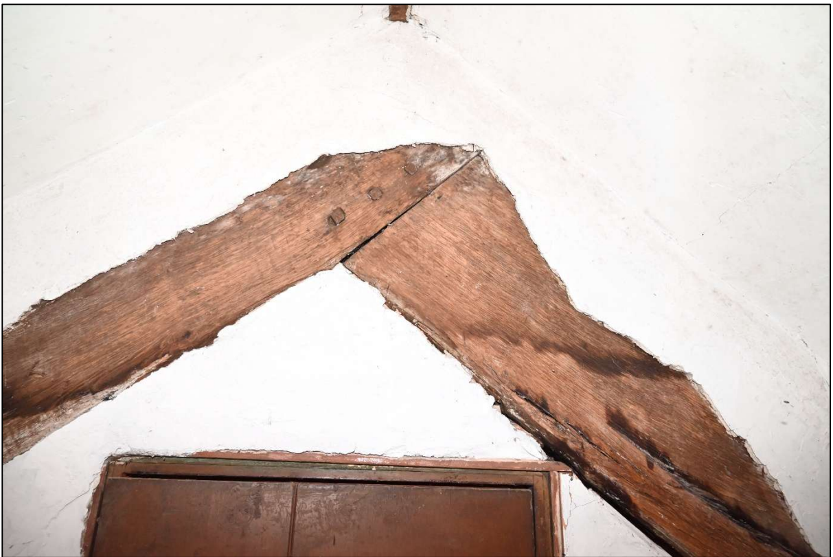
Plate 122: Joint at top of Truss 1
