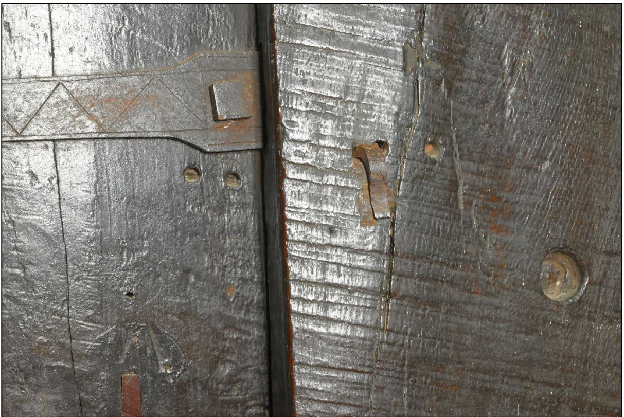
Plate 80: Metal fittings on the eastern door
