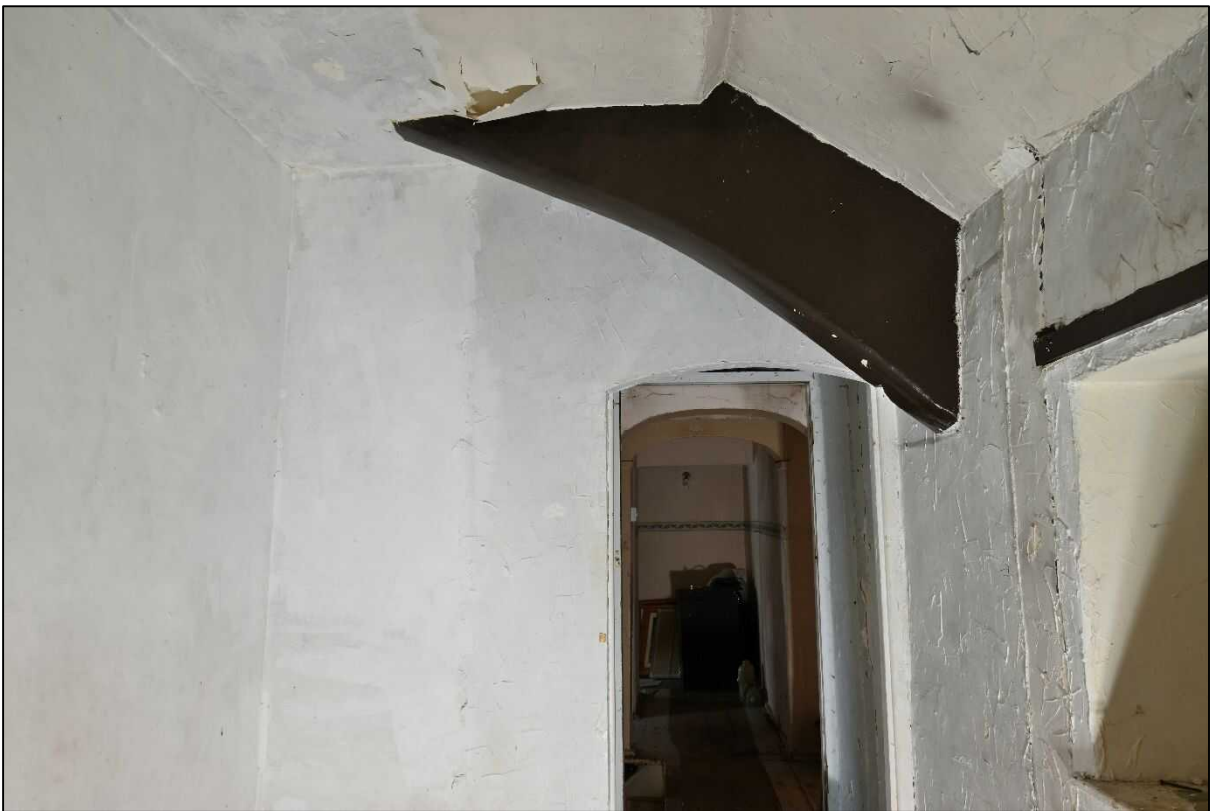
Plate 36: Exposed bas of Truss 3 in NW Bedroom
