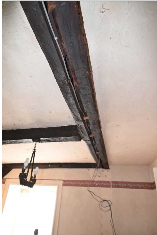
Plate 23: Ceiling beam showing the position of the cross-passage screen
