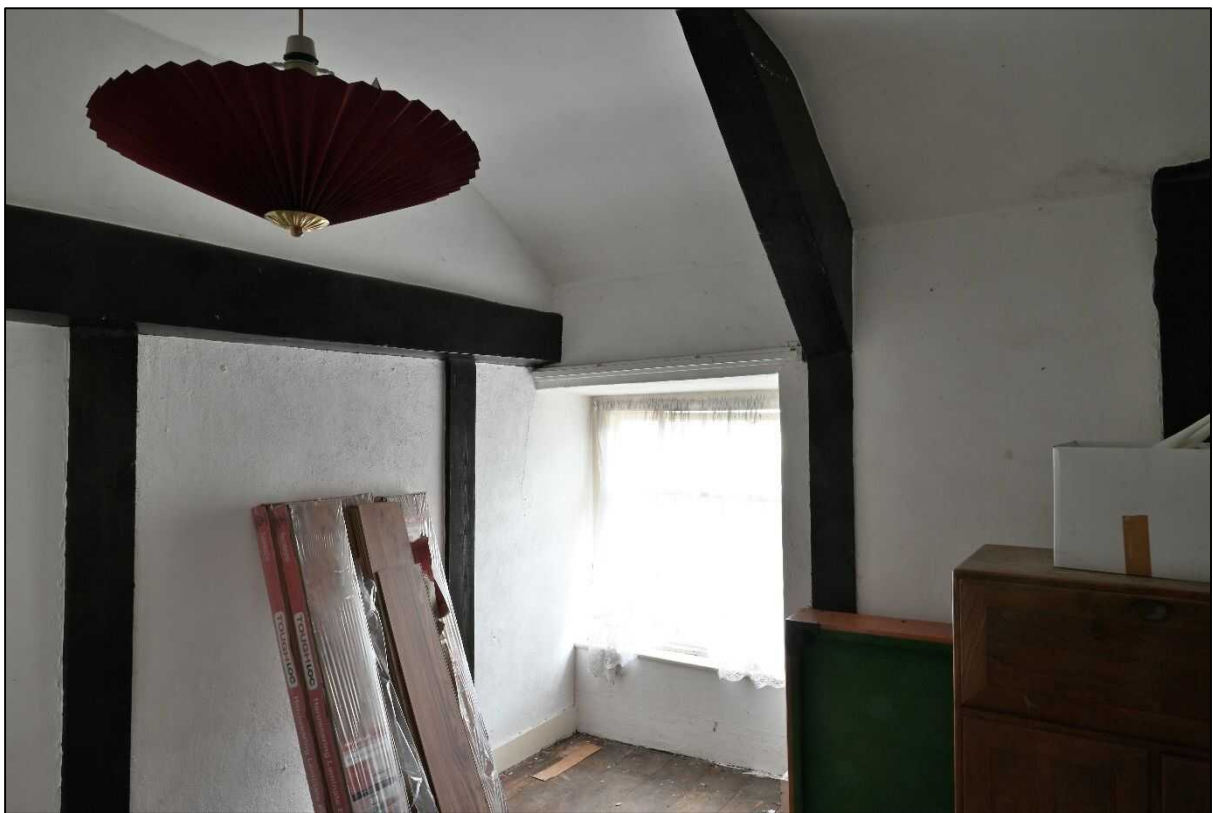
Plate 32: Central Bedroom with exposed base of the Truss 2
