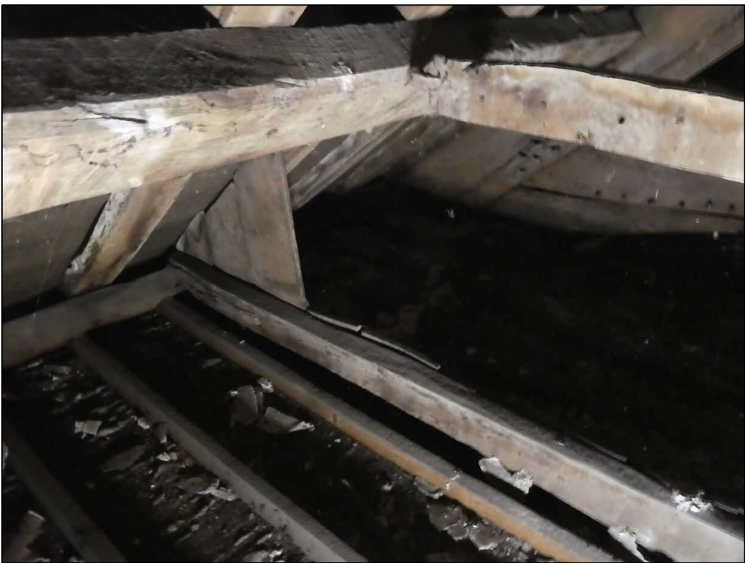
Plate 42: Possible top of a partition between Trusses 2 and 3
