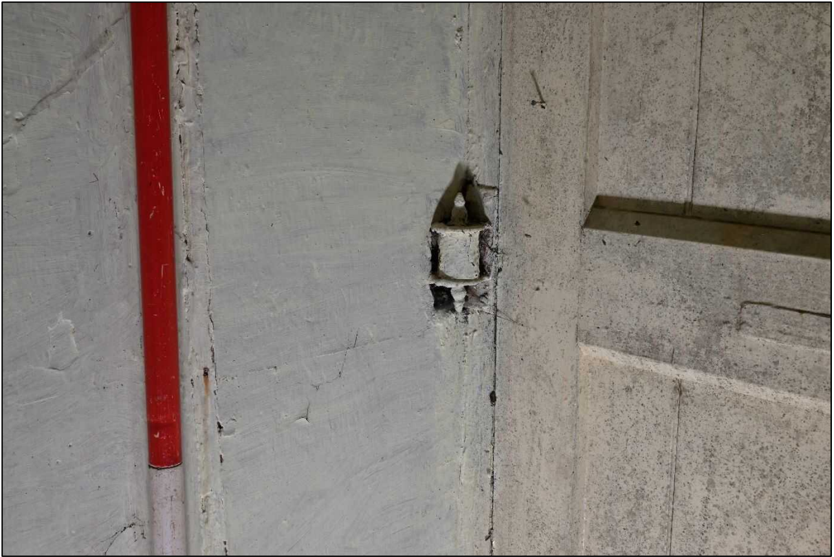
Plate 47: Remnant of door closer on the back door of the Service Range
