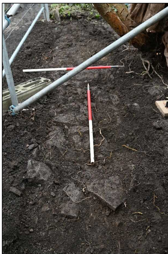
Plate 5: Wall (Context 5), looking north
