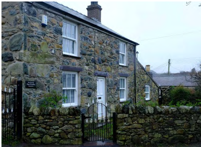
Fig 10 Pant-Ffrydlas farmhouse, built of rubble field stone but with quarried slate lintels, and replacement sash windows.
