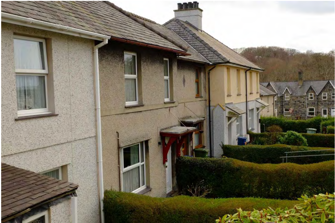
Fig 51 Adwy'r Nant, council houses dated 1934, of pebble-dashed walls, but retaining characteristic bracketed porch canopies.
