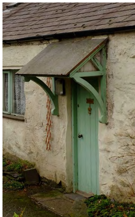
Fig 25 Slate-slab roof on a bracketed porch canopy.
