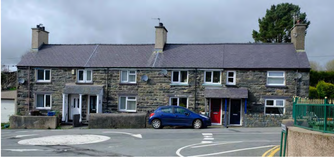
Fig 44 Houses in Penybryn Road are mostly of quarried stone in large blocks, and built either in pairs or rows of four.
