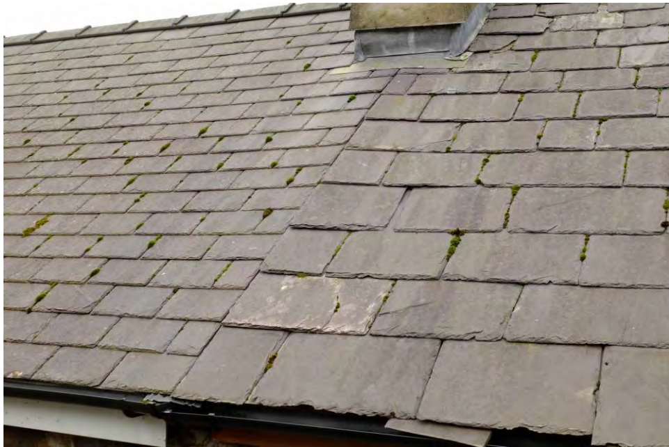
Fig 22 Roofs on Penybryn Terrace have slates of different sizes, the left side having been re-roofed.
