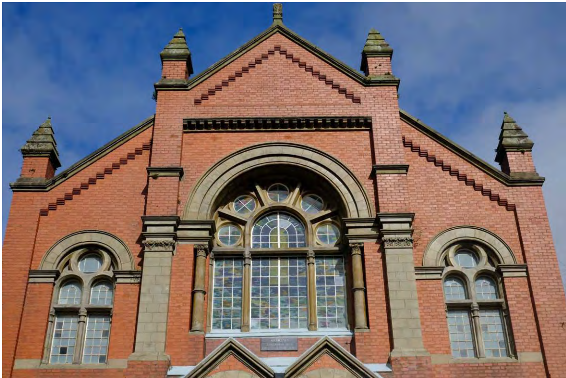
Fig 28 Capel Bethania was built of bright-red Ruabon brick, with sandstone dressings, and therefore of non-local materials.
