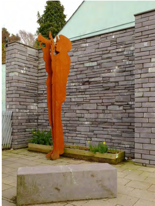
Fig 29 Slate remains an important local building material, used here for the retaining walls of Llys Dafydd in the centre of the town.
