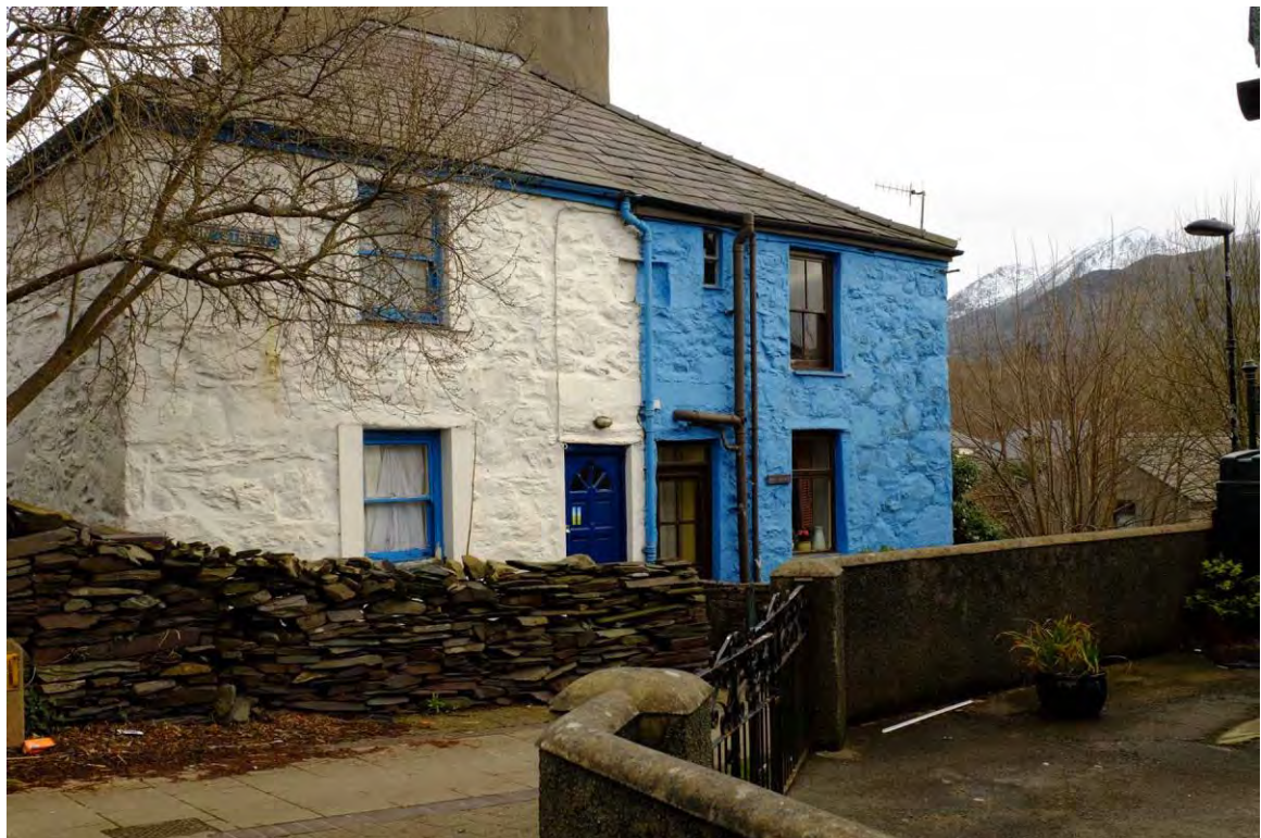
Fig 39 10-11 John Street, are unusual in sharing a hipped roof, and for retaining sash windows.
