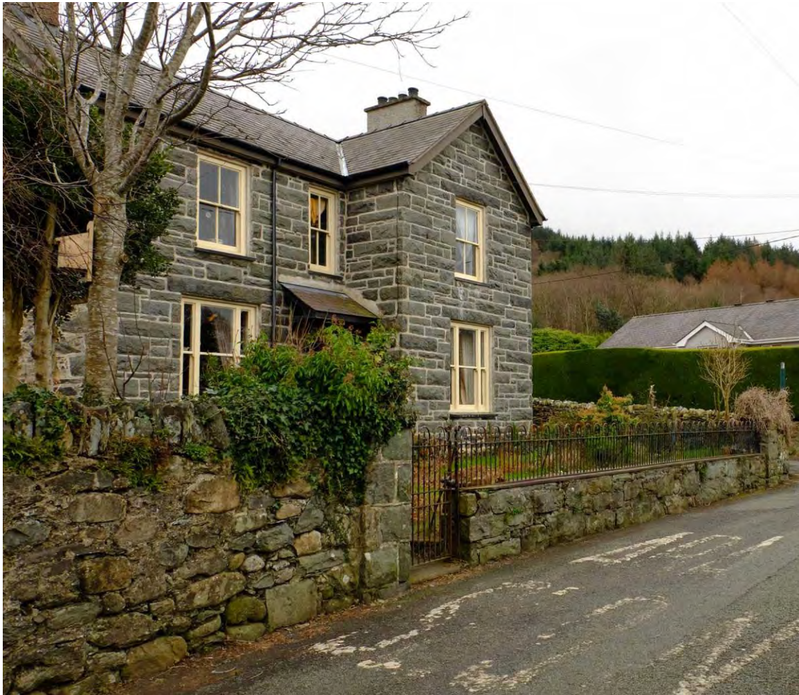
Fig 16 Llys Llewelyn, an individually built house in Braichmelyn, distinguished by being built of rock-faced quarried stone.
