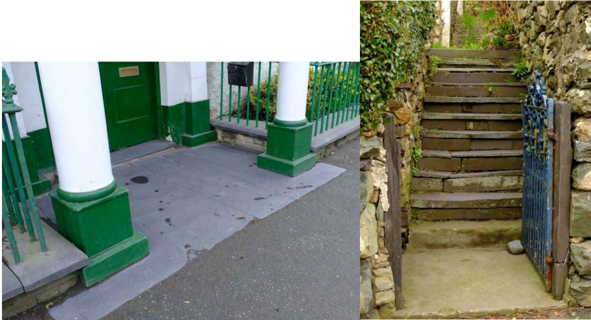
Fig 24 Slate paving slabs and gate piers.
