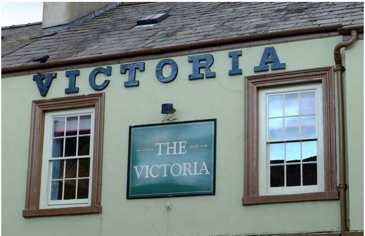
Fig 27 The roughcast front of the Victoria Hotel, with smooth-rendered architraves and raised letters.
