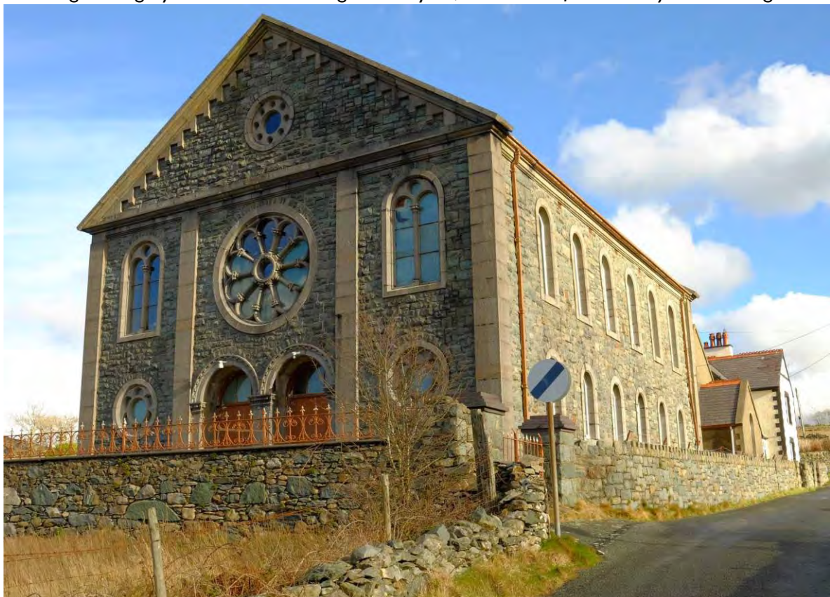
Fig 14 Cefn y Waen Chapel, 1868. Its gable-end front is built of snecked, rock-faced stones with freestone dressings.
