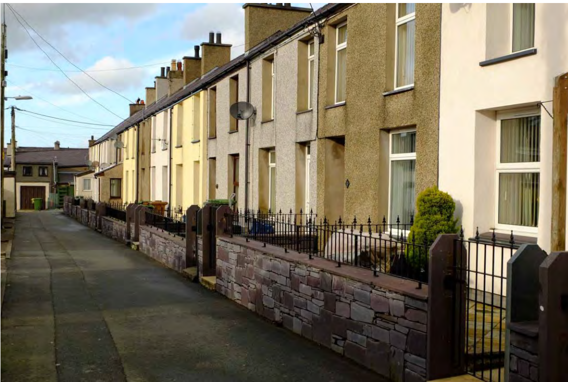
Fig 9 Rhes Marian, two-window houses built in the second half of the nineteenth century, setback from the street behind garden walls.
