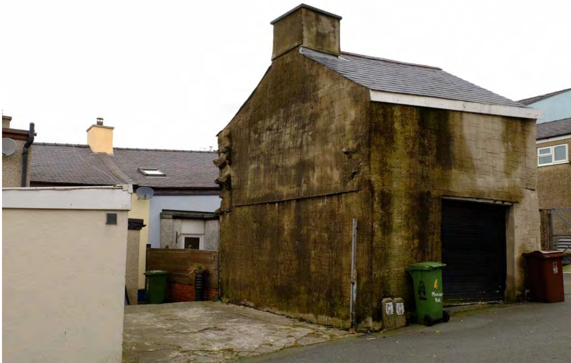
Fig 8 The shell survives on one of the houses that made up Back New Street.
