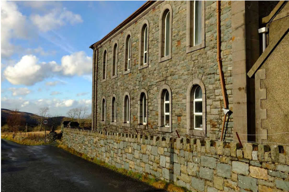
Fig 25 Cefn y Waen chapel. The boundary wall of snecked, quarried stone.
