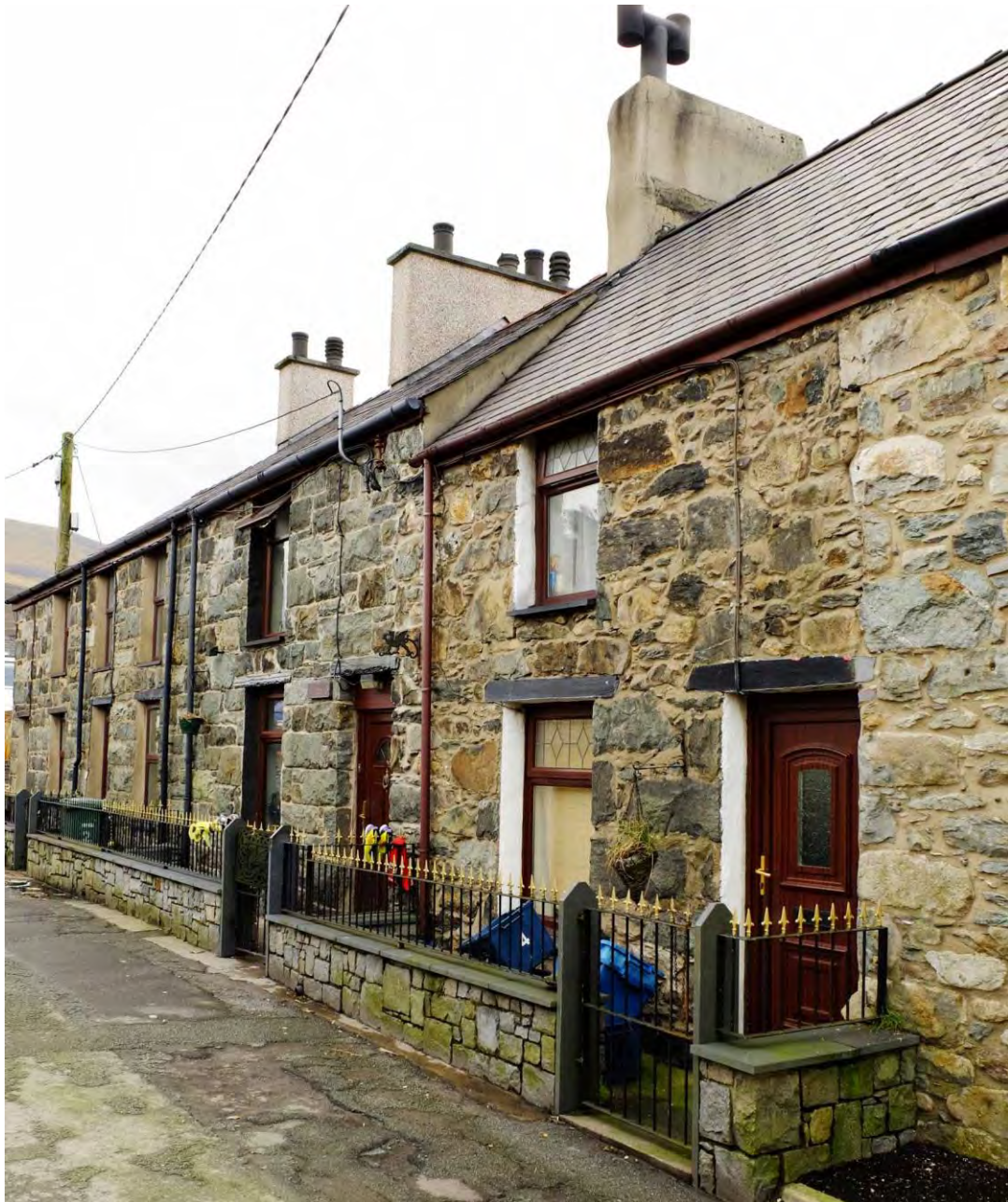
Fig 18 Houses in Tabernacle Street. The house on the right is built of random rubble stone, the later houses further left of quarried stone roughly shaped into blocks. All openings are under lintels of slate blocks. The snecked-stone garden walls are later. Originally the houses opened directly on to the street.
