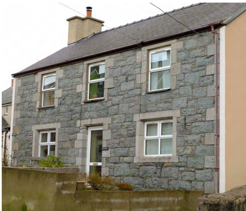
Fig 12 Bro Dawel, an individually built house in Ffordd Deiniol, of sneaked quarried stone, with light-grey granite dressings and quoins.
