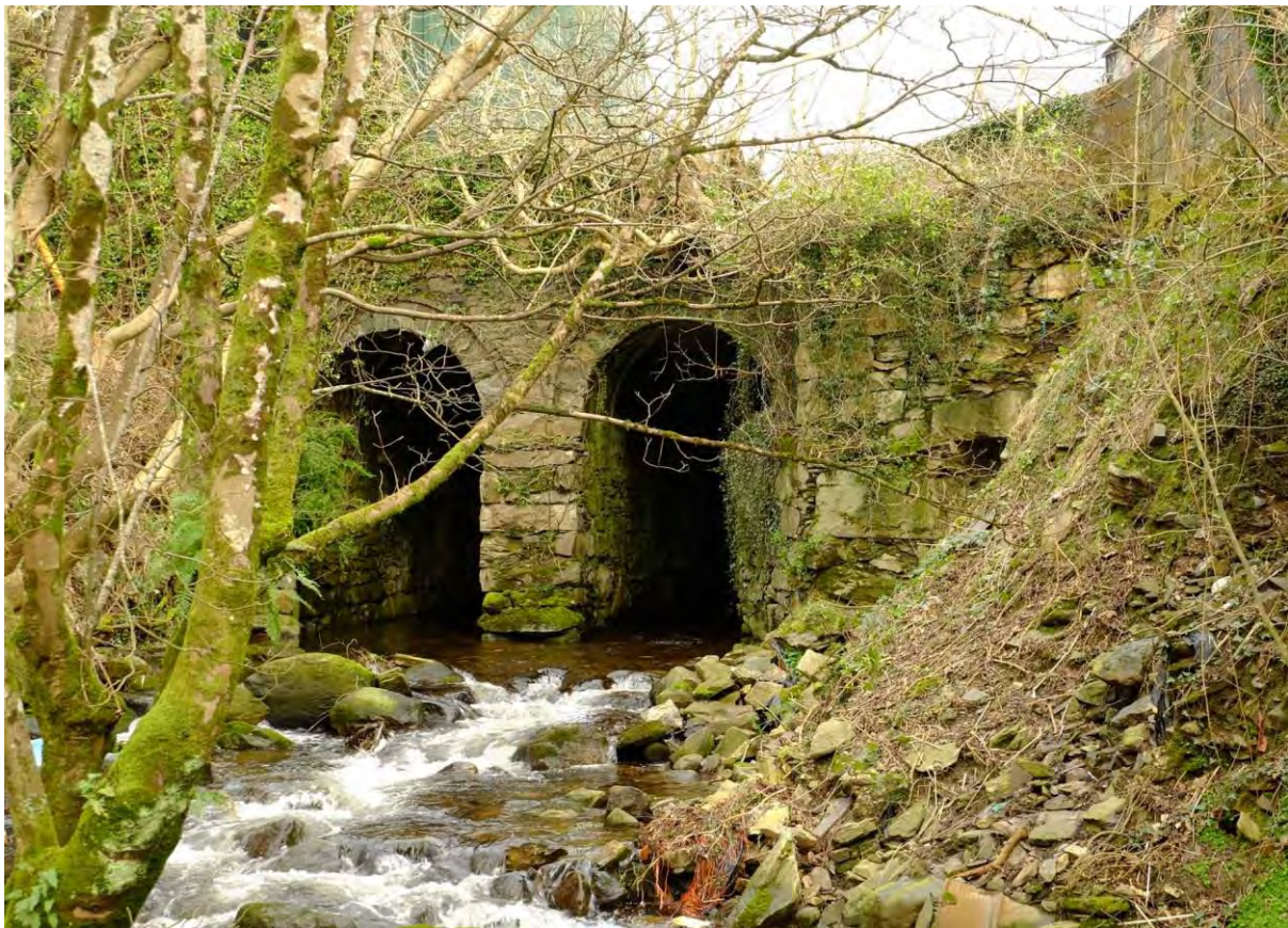
Fig 40 Stone-built culverts beneath the yard of Glandinorwig writing-slate mill.
