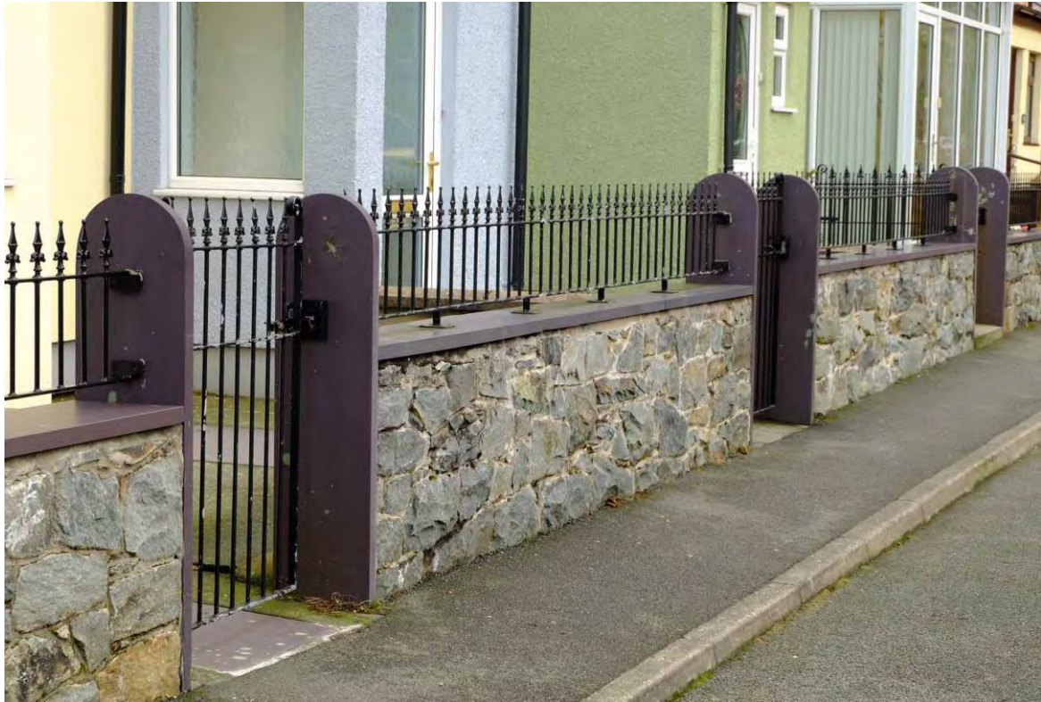
Fig 20 Rubble-stone garden walls with sawn slate used for gate piers and coping courses.
