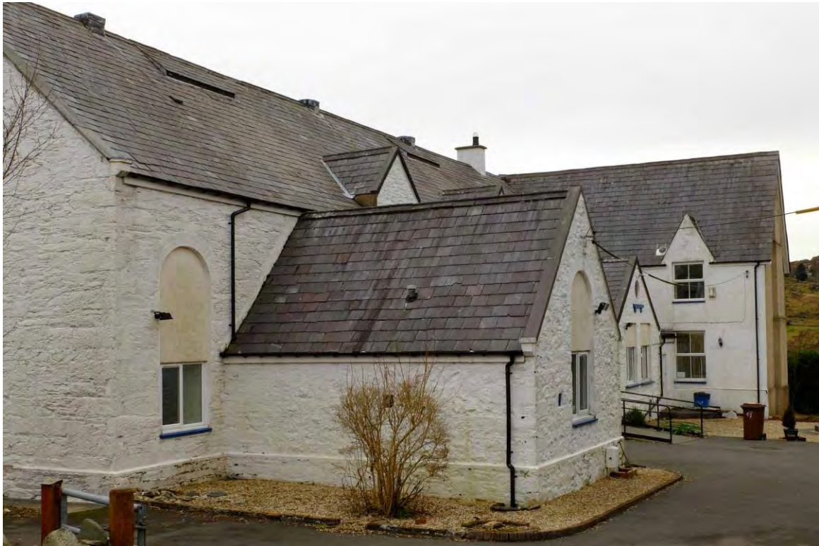
Fig 16 The former non-denominational school, with distinctive tall round-headed windows.
