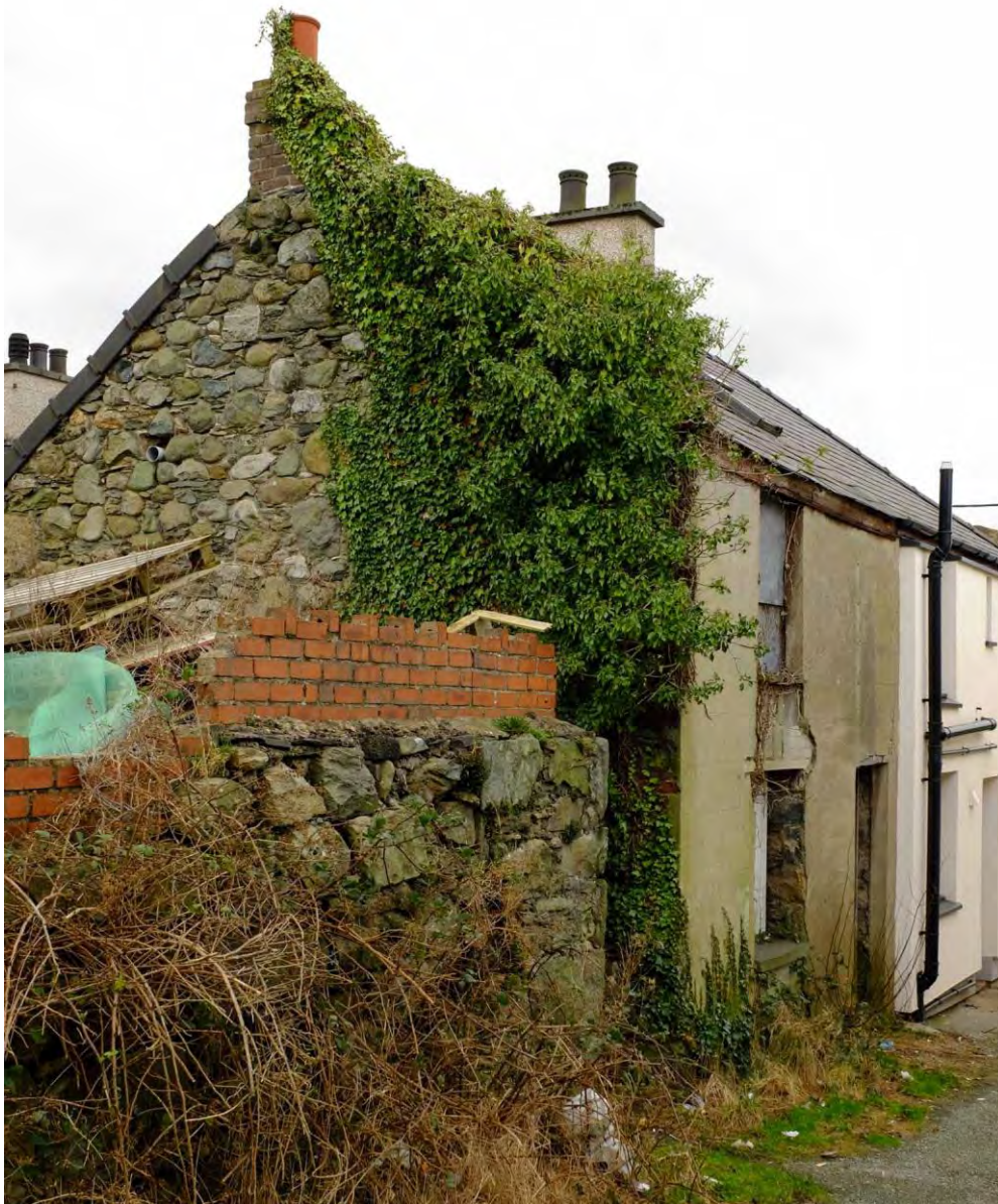
Fig 19 The poorest-quality materials are often to the side or rear, as seen here in a house behind Green Terrace, built of field stone.
