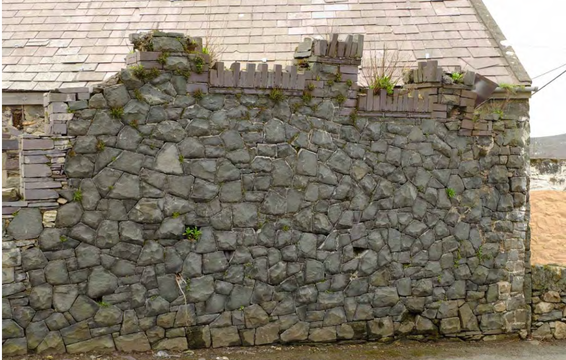
Fig 22 The boundary wall of Glandinorwig writing-slate mill has randomly shaped quarried stones pieced together in a crazed pattern, with slate blocks for the coping course.
