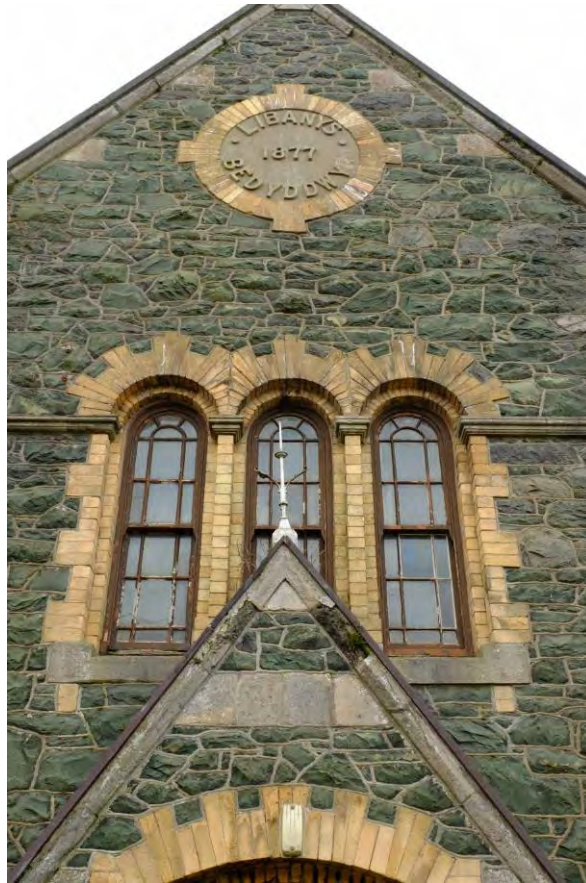
Fig 33 Detail of Capel Libanus, faced in random quarried blocks pieced together in a crazed style, and with brick window dressings.
