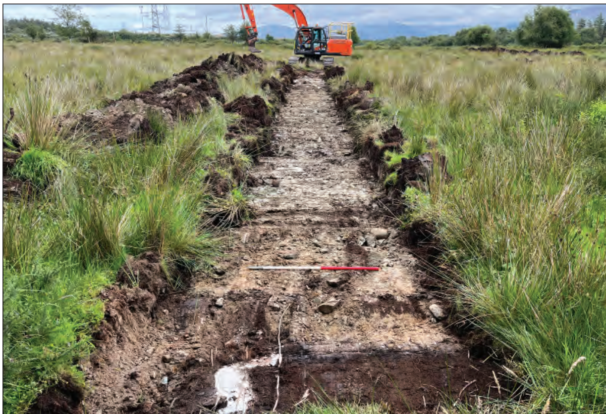
Plate 03 - Trench 18 overview facing east
