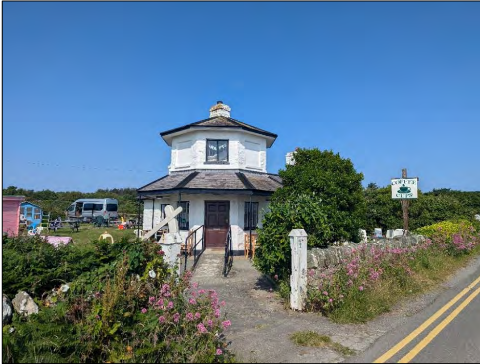
Figure 8 Stanley Toll House (LB2)
