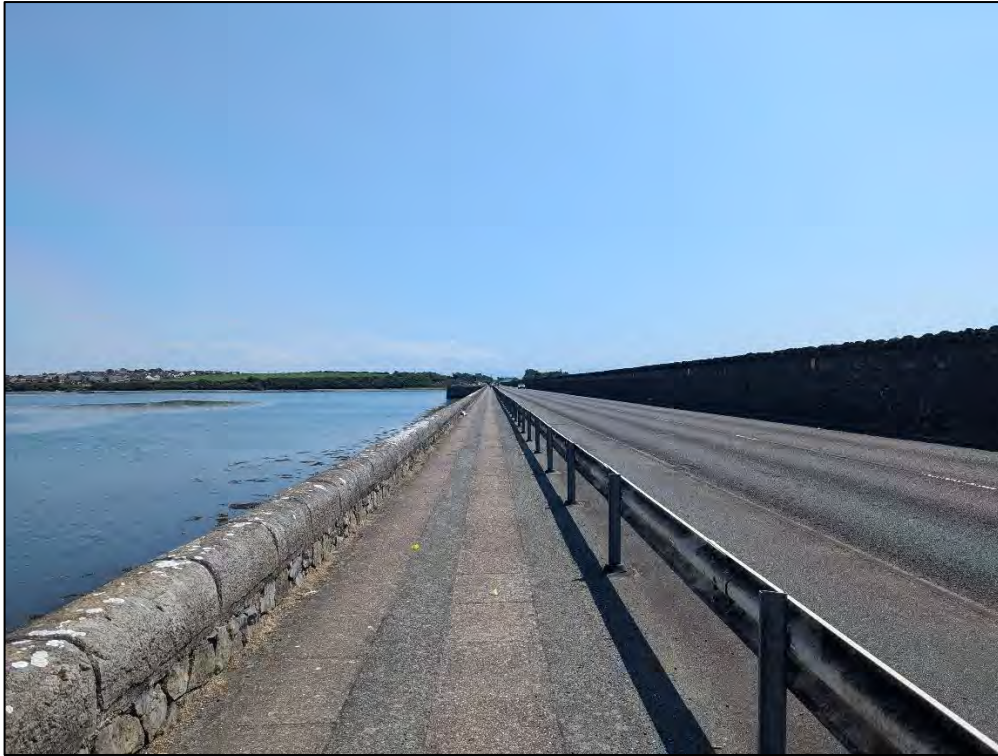
Figure 7 View south-east along Stanley Embankment (LB1)
