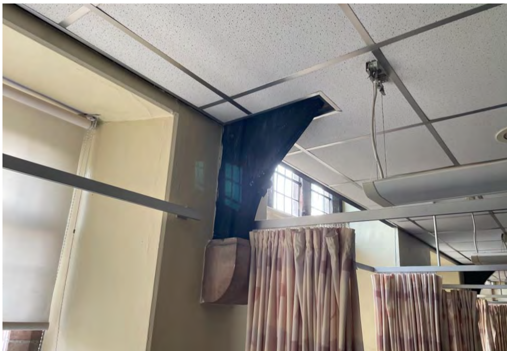
Figure 3.7: Concealed timber roof truss and modern suspended ceiling in the principal range
