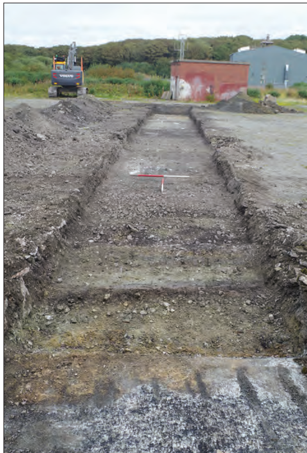
Figure 8: Trench 2 (prior to sondage excavation), tarmac 203 in foreground, view from south-west, 2 x 1 m scales
