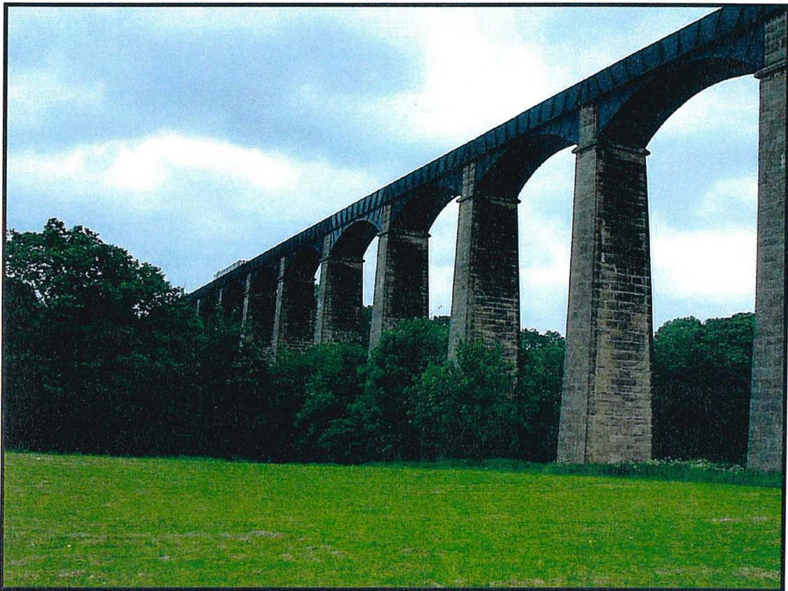
Figure 6.1 Vegetation near the Aqueduct
