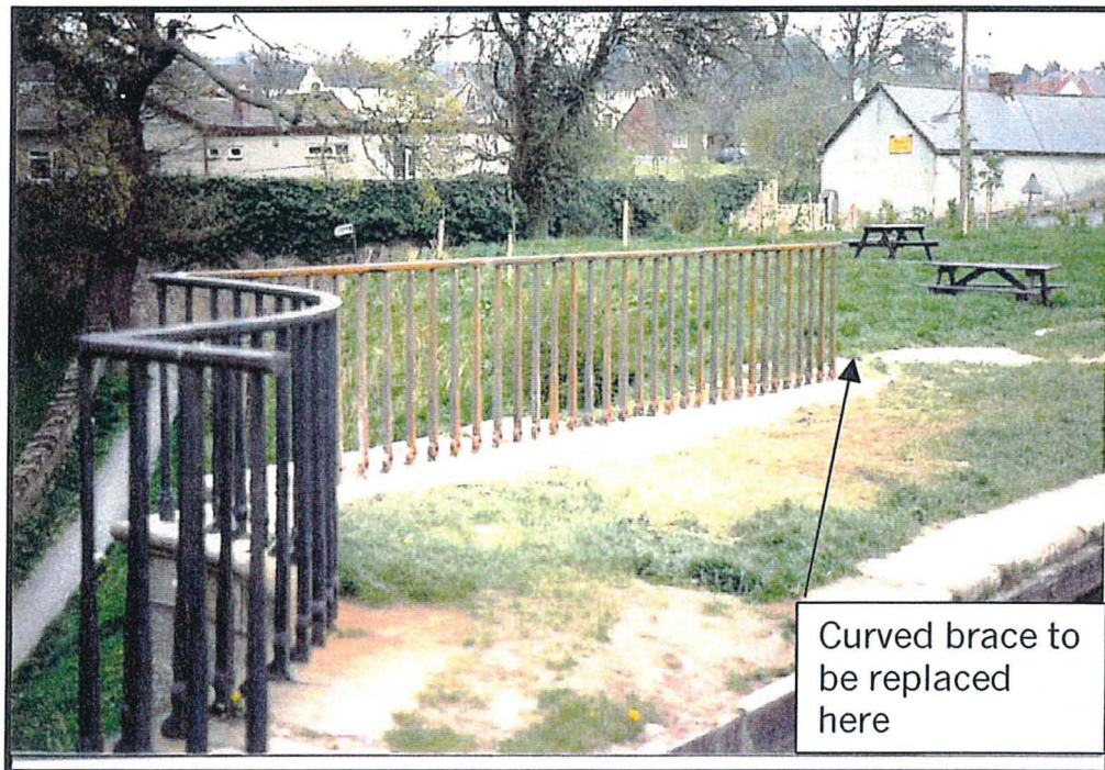
Figure 3.3 – Proposed location of curved braces (north west)
