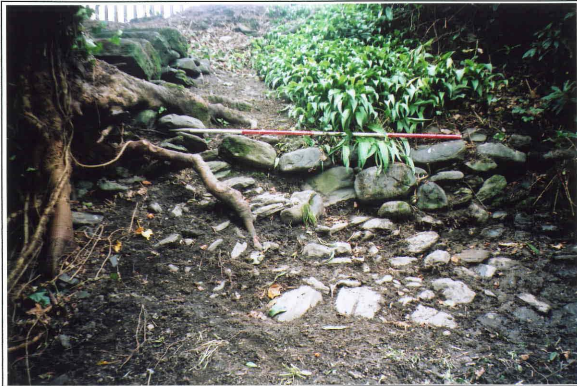
Plate 15 Path and retaining wall between upper and lower steps. Photo CPAT 1183.07
