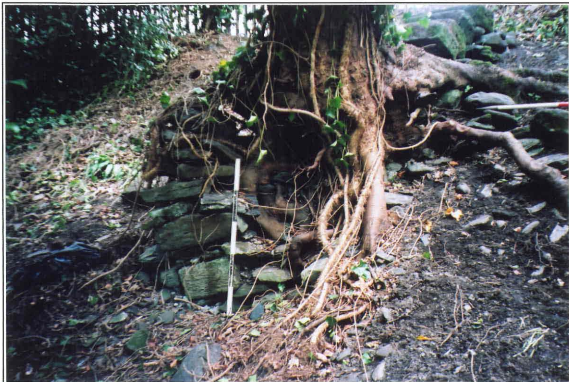
Plate 14 Retaining wall for upper steps. Photo CPAT 1183.08
