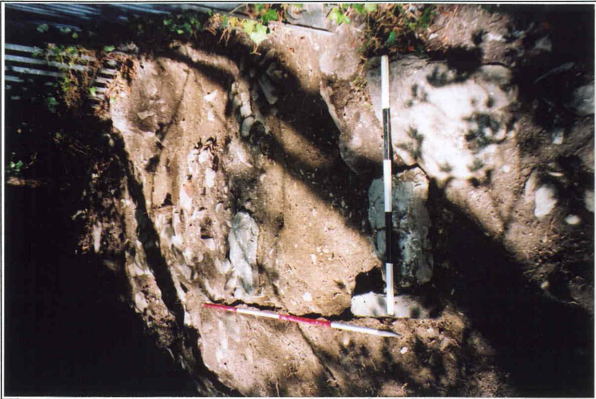
Plate 9 Summer-house foundations, west side. Photo CPAT 1183.09
