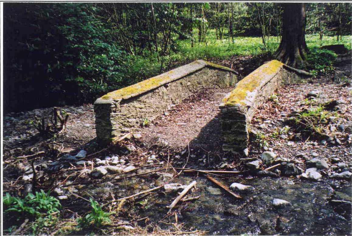
Plate 6 Bridge 5 and new stream channel. Photo 1178.13
