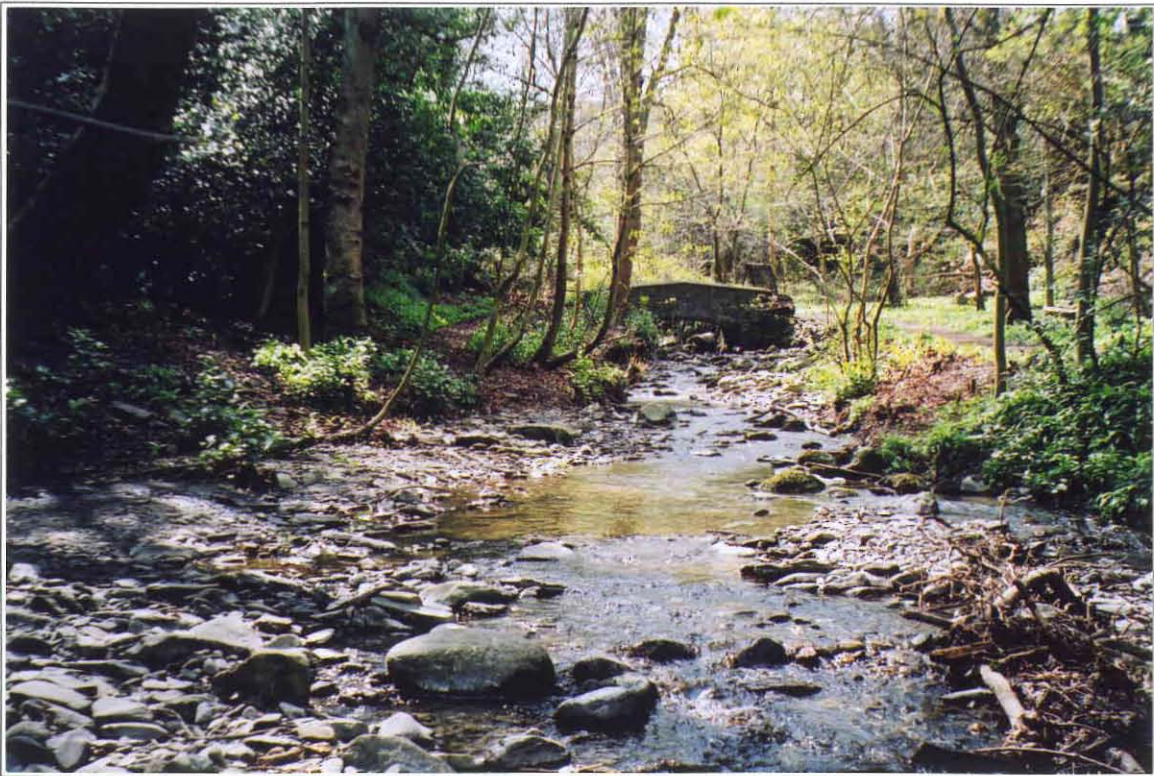
Plate 2 Bridge 3 and Afon Cyflymen. Photo CPAT 1178.09
