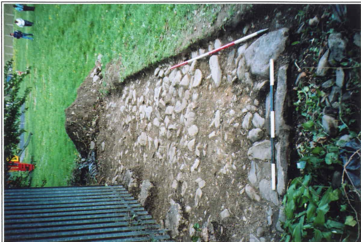
Plate 12 Summer-house foundations, east side. Photo CPAT 1183.18
