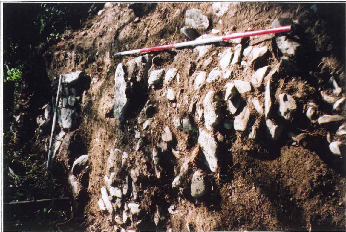
Plate 10 Summer-house foundations, west side. Photo CPAT 1183.13
