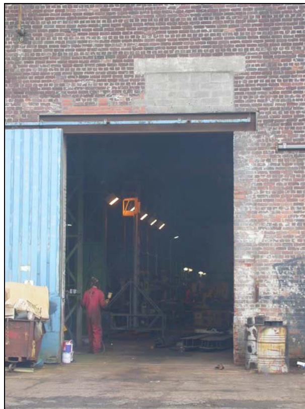
Plate 6. View of HMR3 showing various alterations to structures
