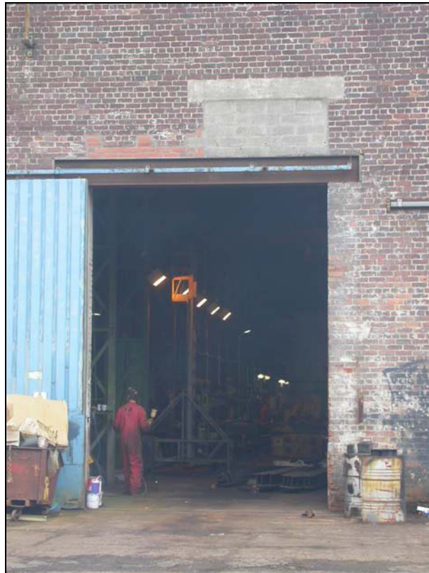
HMR 3 Showing various alterations to structures ©GGAT
