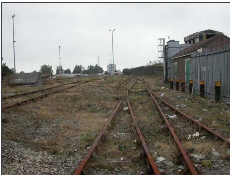
Plate 2. View of railway sidings HMR15, west of site to south
