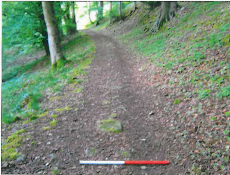
Plate 1: Part of Section IWT001(ii) Depicting a Surviving Stretch of Stone Blocks, View to Northeast
