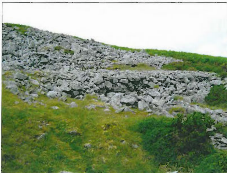
Plate 6: Revetted Causeway (IWT006/015) along Section IWT006(ix), View to North
