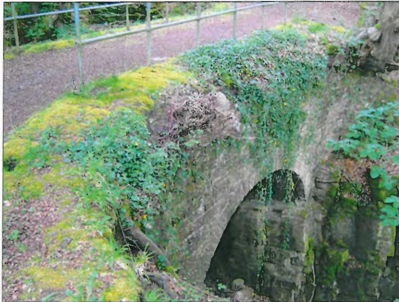
Plate 3: Listed Bridge (23814) Within Section IWT003(iii), View to Southeast
