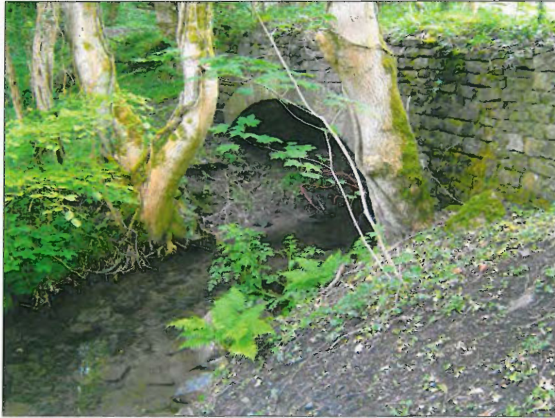
Plate 13: Single Arched Stone Bridge (IWT013/021) on Section IWT013(ix), View to Northwest
