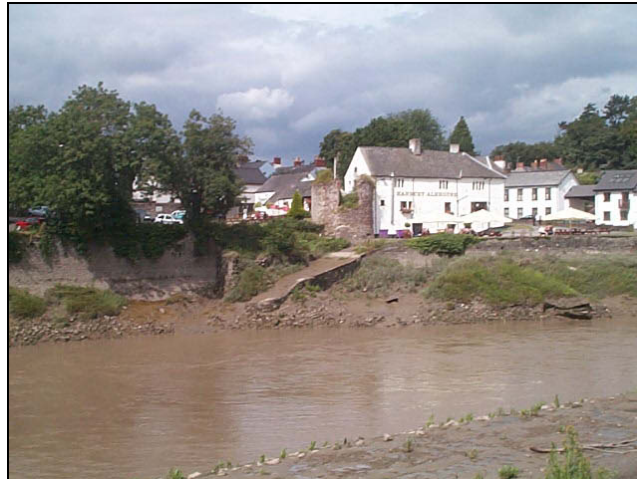
View of a Caerleon slipway with Hanbury Tower behind, looking north
