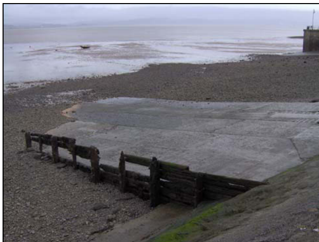
Plate 59 View of Slipway (05795w), looking southeast
