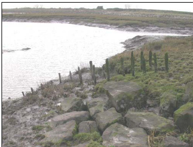
Plate 27 View of Stakes (08893g), looking west
