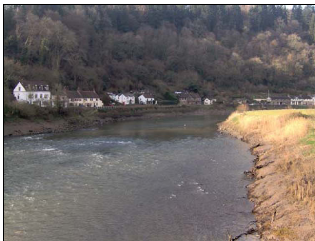
Plate 1 View of Ash Weir (00730g), looking northwest
