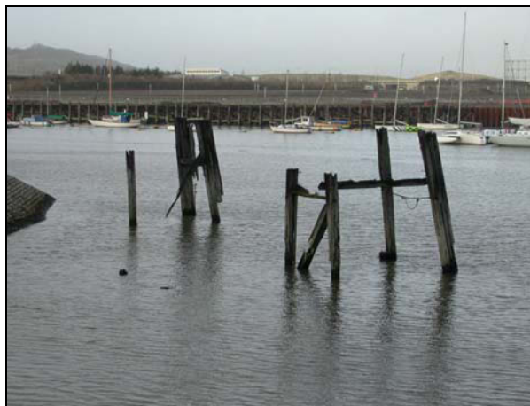
Plate 33 View of Jetty (03987s), looking northeast
