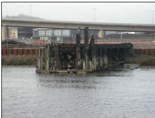
Plate 34 View of Coal staithe (03988s), looking north
