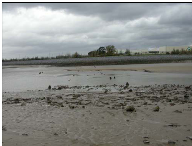
Plate 79 View of Old Loughor road bridge (01250w), looking northwest
