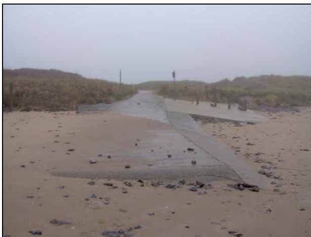
Plate 71 View of Slipway (05790w), looking northwest
