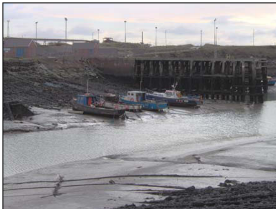
Plate 49 View of Port Talbot lock (03124w), looking northeast
