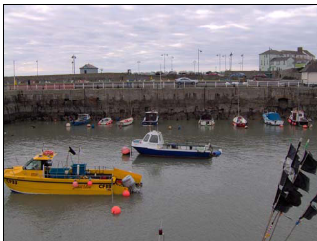
Plate 47 View of Porthcawl harbour (02537m/34275), looking west
