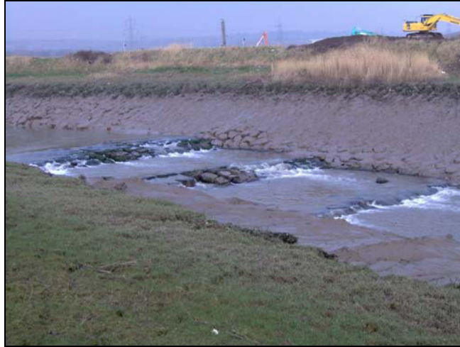
Plate 24 View of Weir (08891g), looking northeast
