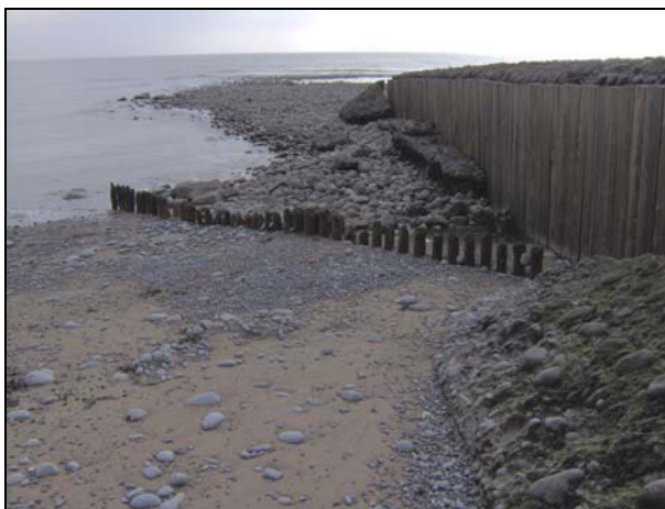
Plate 41 View of a stakes (03984s), looking south
