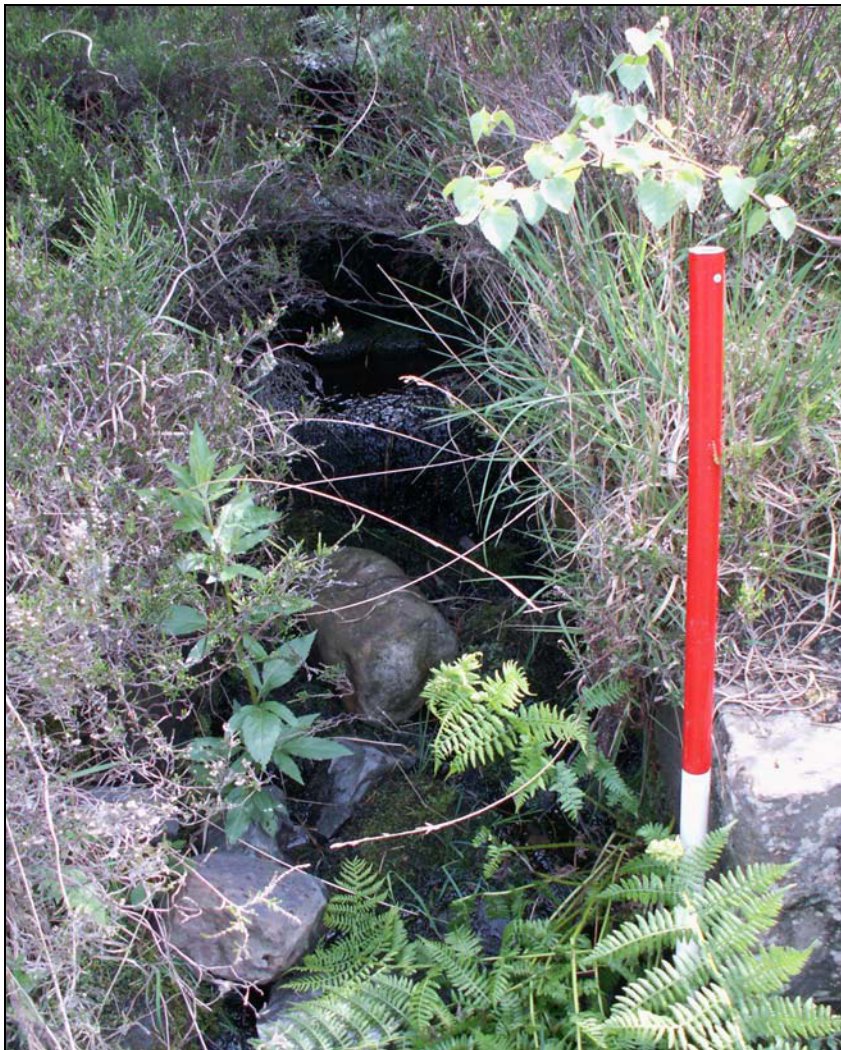
Plate 4: LSV005 Drainage System view to east
