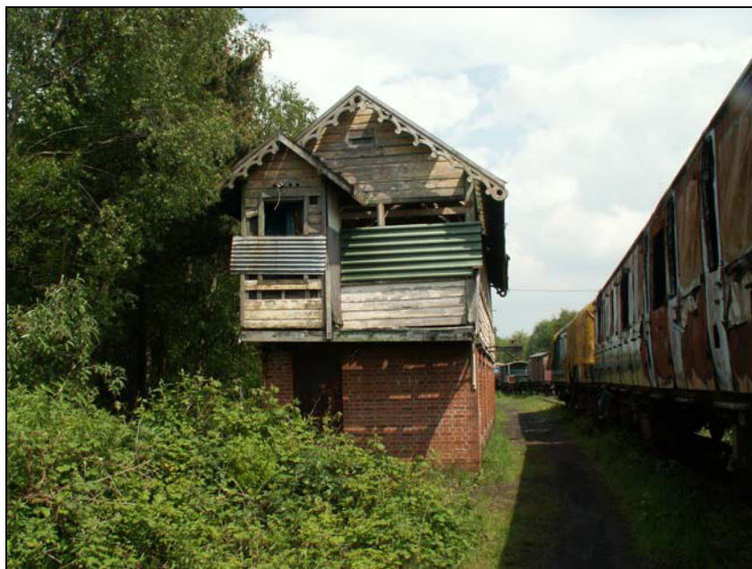
Plate 2: Signal box serving Swansea Vale Railway
