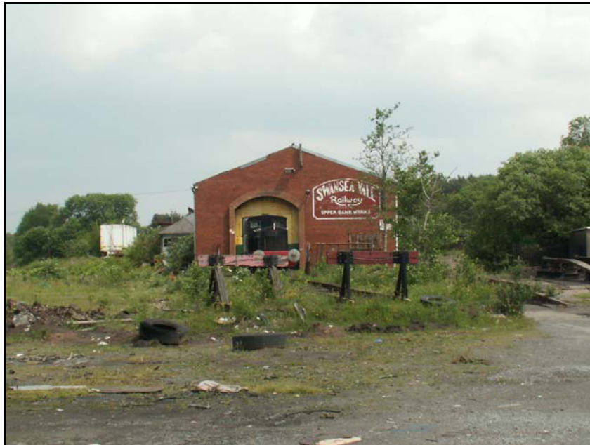
Plate 1: Swansea Vale Railway Engine Shed
