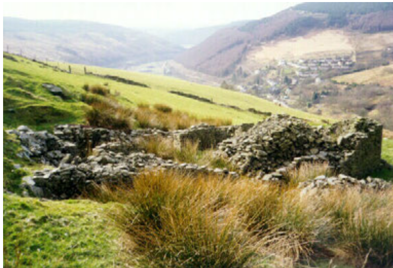
Site 2048m, Glyncorrgw, Neath and Port Talbot, looking southwest. The interior is filled with rubble from demolition.
