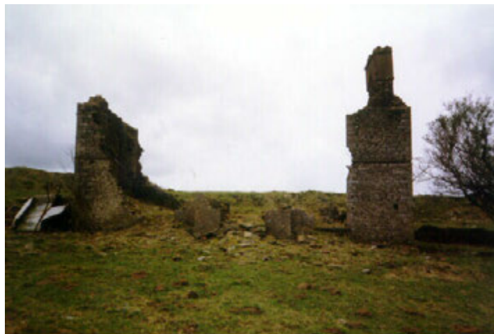
Plate 4: Site 5657w, Pen-y-Lan farmhouse, built of stone, with a central porch and stairway. The farm may be a post-medieval successor to a grange of Neath Abbey.
