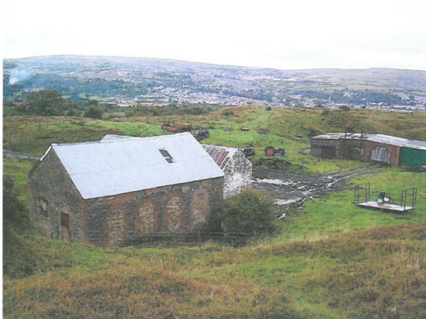
Cwm-du Drift (Cwm Glo), engine house and stables, looking northeast
