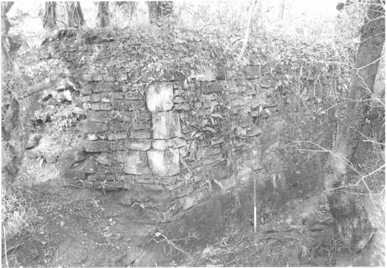
Plate 3: Abutment of tramway bridge
