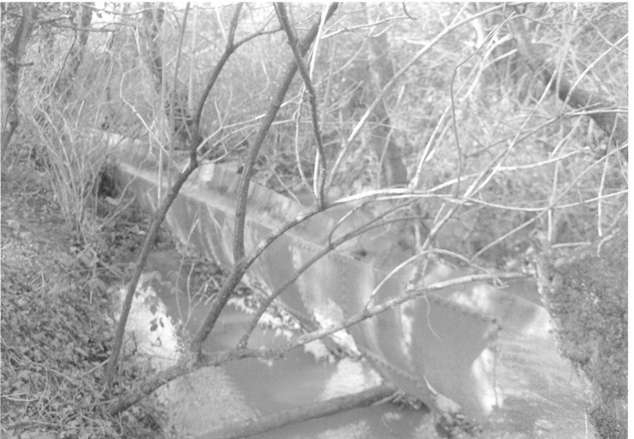
Plate 2: Iron water channel
