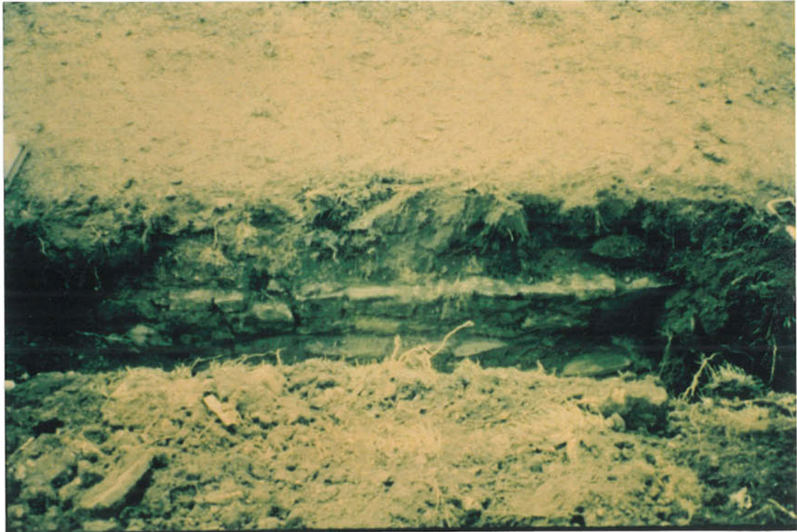
Plate 1: Section of wall located in Area 2.
