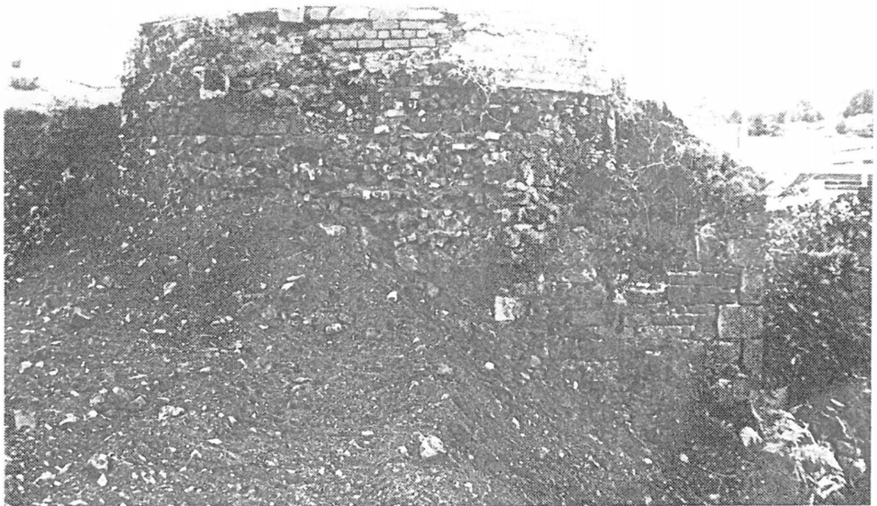
fig 9 Pit Head Shaft
