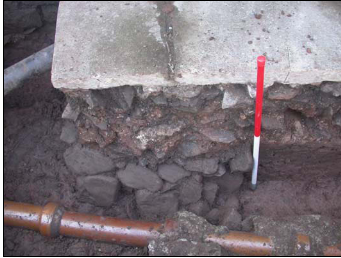
Plate 1. Showing stone foundation 017 cut (019) through natural deposit (015)
