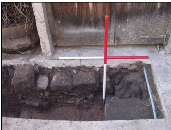
Plate 2. View to the west of re-used dressed stone laid floor of outside toilet.
