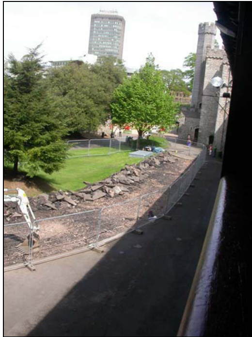
Plate 11: Overview of excavated area, looking east
