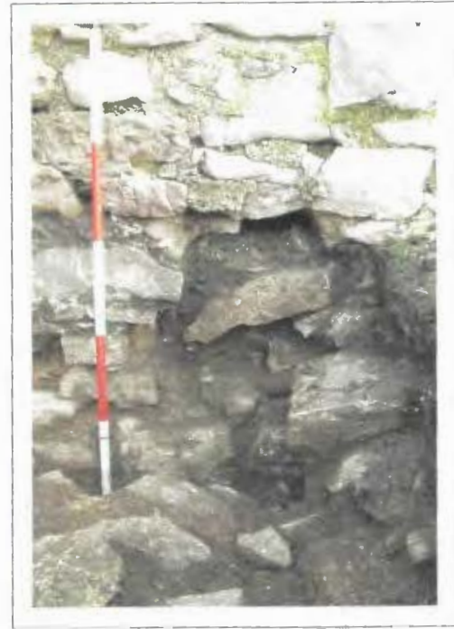
Plate 04: drain [6], void in curtain wall, looking east. Scale 1m
