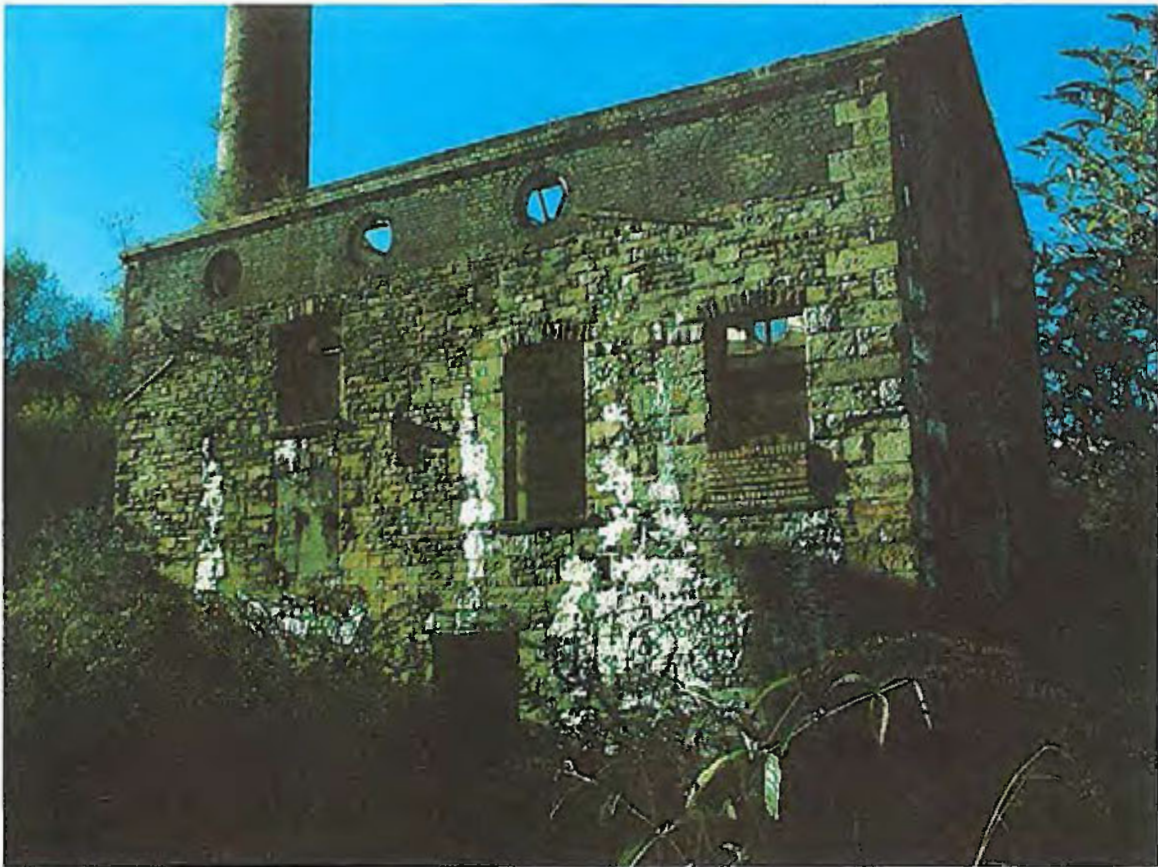
Photo 9 - Building 8.0 (Hafod Vivian engine house) from the south
