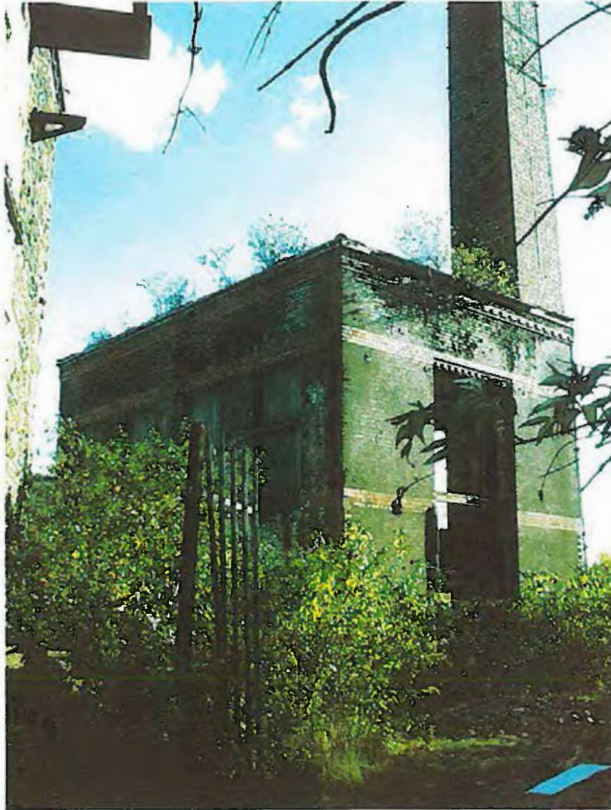
Photo 10 - Building 9.0 (Hafod Musgrave engine house) from the north
