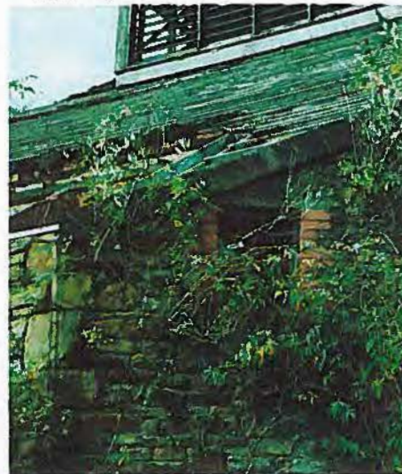
Below centre: vegetation growth on the north east corner of the building; intrusive root growth has resulted in the dislodging of masonry.
