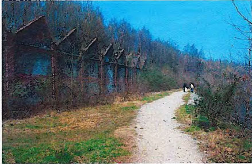
P41: Close proximity of footpath to Locomotive Shed
