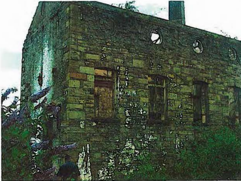
Left upper: north elevation of the Vivian engine house, the upper portion is built in copper slag bricks.
