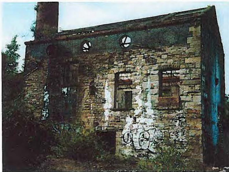
Left lower: south elevation of the engine house.
