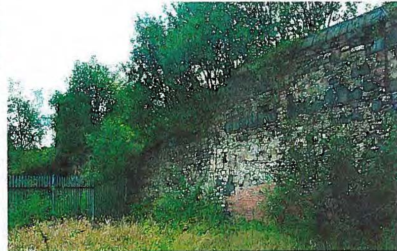
Above: east face of the boundary wall at its northern end near the Laboratory building; the wall is constructed of copper slag and rubble stone capped with pointed copper slag coping blocks. Below: west / canal face of the boundary wall; a wide brick arch near the base of the wall formerly acted as an entrance to one of the canal dock basins.
