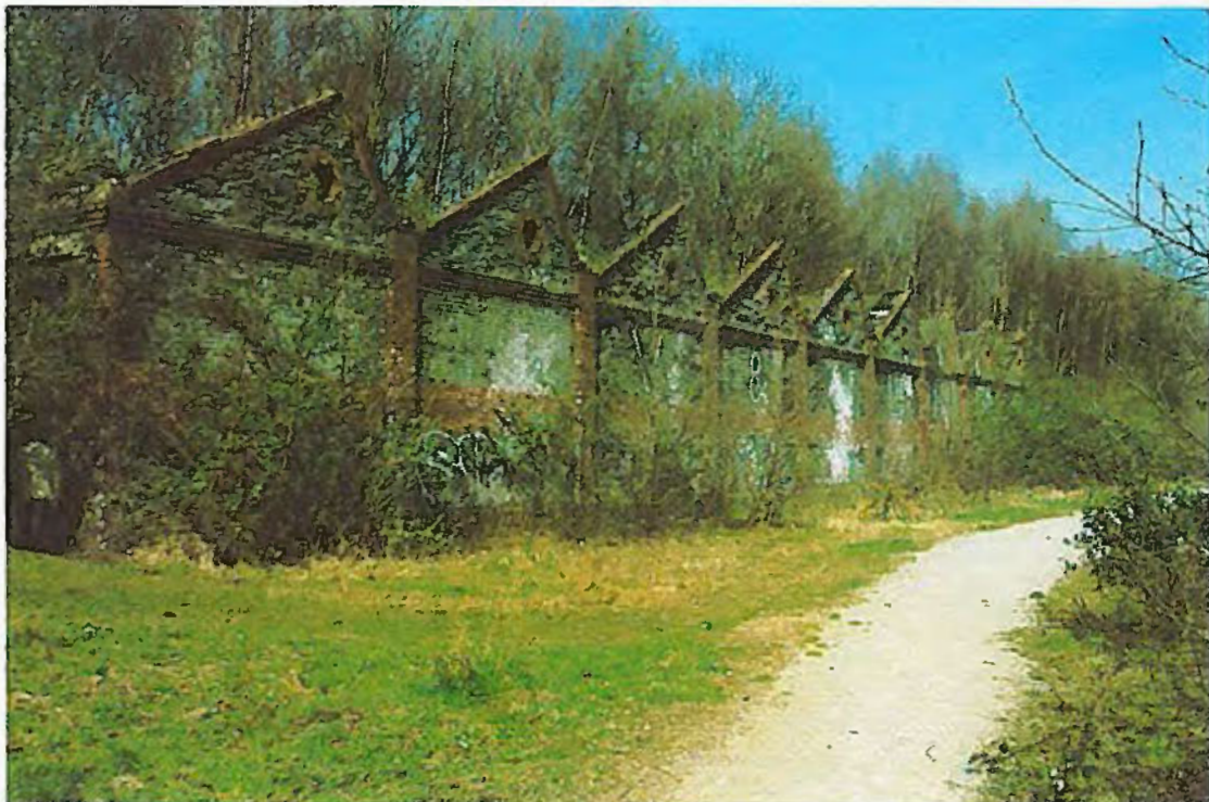
Photo 11a - Building 11.0 (Vivian Locomotive Shed) from the southeast
