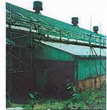
Right lower: modern steel framed profiled metal clad extension at the north end of the museum stores.
