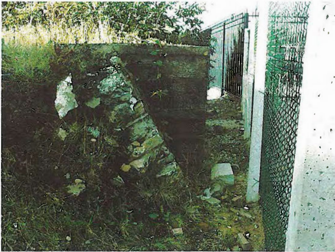
Photo 14c - Area 4, the remains of revetment wall YIM 42 from the south
