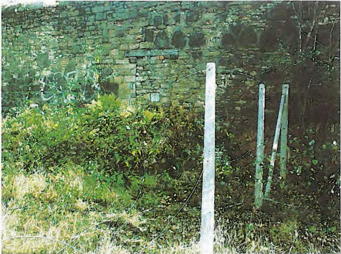
Photo 4b - Building 3.0 (canal wall) from the west showing blocked archway and doorway to canal basin YIM 12, and towpath YIM 33
