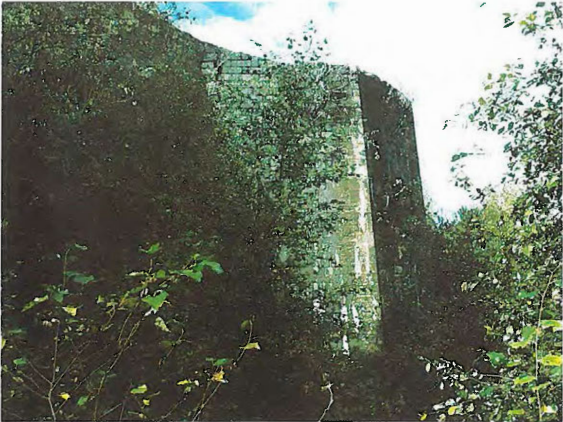
Photo 5 - Building 4.0 (Hafod copper slag abutment) from the SE
