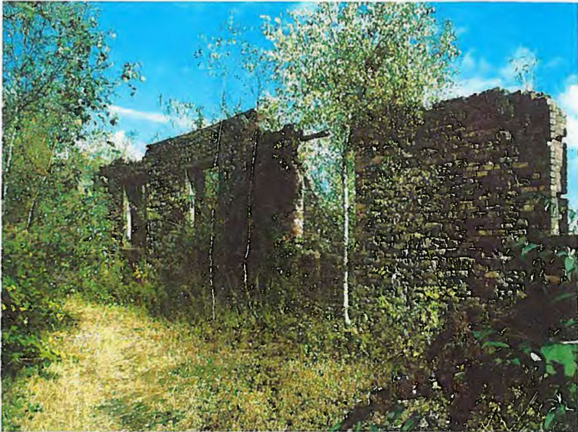
Photo 14a - Area 4A, part of building YIM 40 from the southwest (exterior)
