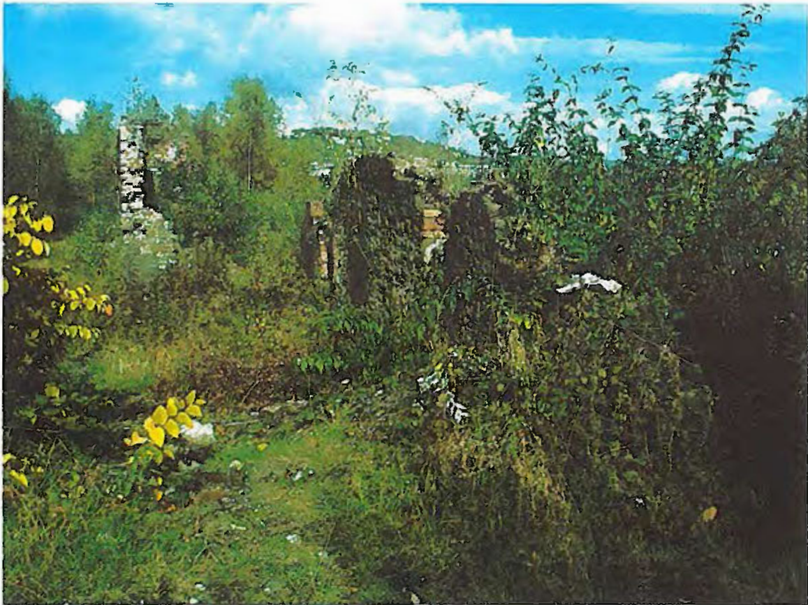
Photo 14b - Area 4A, part of building YIM 41 from the southwest (exterior)
