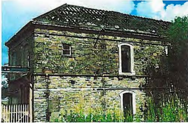
Left upper: west elevation backing on to the Swansea canal.
