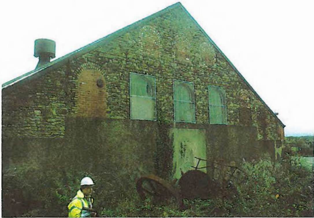
Photo 1b - Building 10.0, Museum Stores/rolling mill, from the NE showing primary arch (c.1830), later blocked
