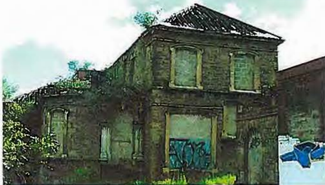
Left centre: north elevation.
