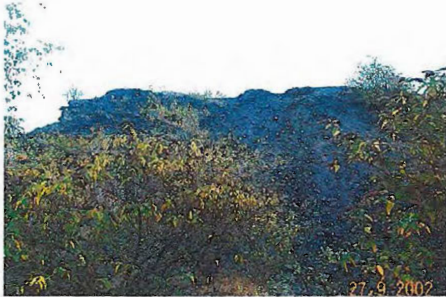
P19: Rear of structure 4 (access to unprotected drop).
