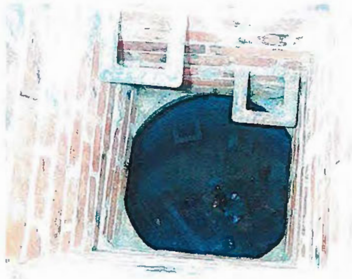
P11: Uncovered culvert chamber.
