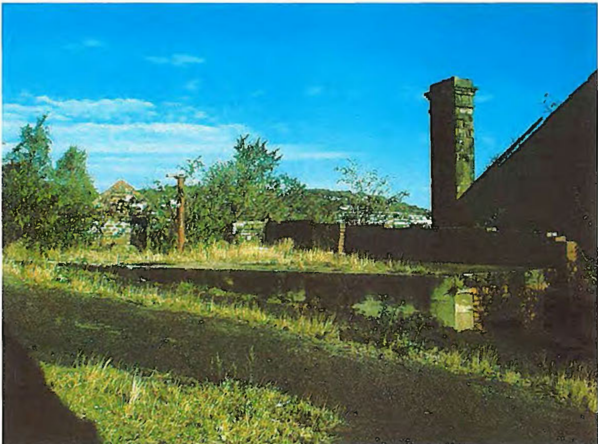
Photo 12 - Area 2, later 20th century tank YIM 37 from the south
