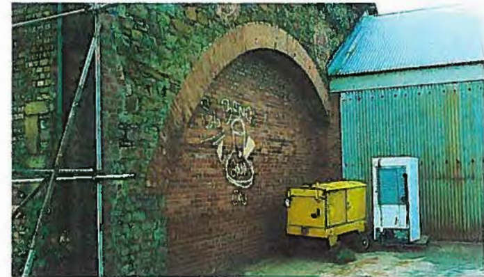
Right upper: north gable with wide infilled brick arched opening.
