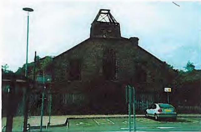
Left top : east gable elevation and clock tower frame of the former Canteen Building.
