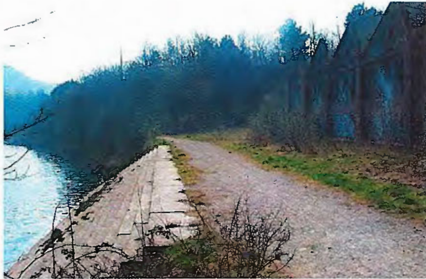
P31: Unprotected edge to River Tawe
