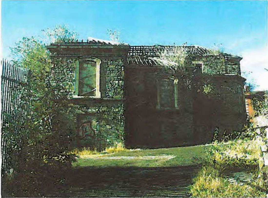
Photo 3a - Building 2.0 (Laboratory) from the east showing main facade (1880s)
