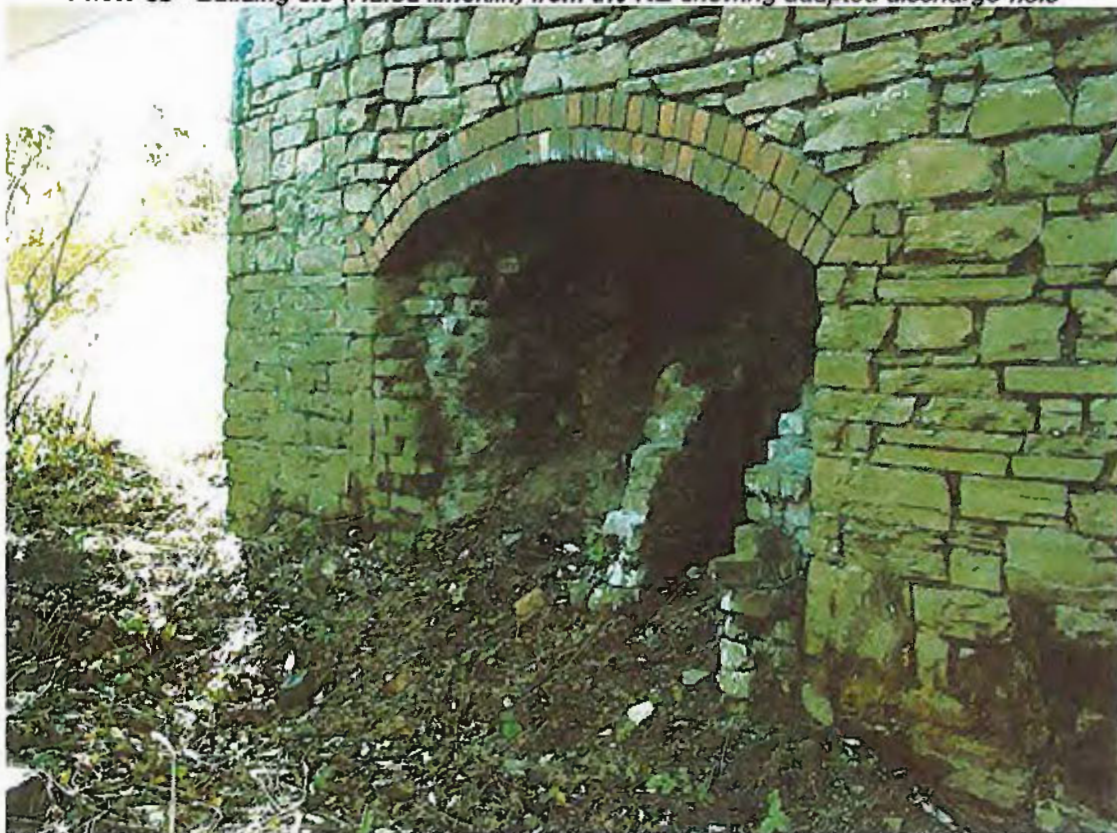
Photo 6b - Building 5.0 (Hafod limekiln) from the NE showing adapted discharge-hole
