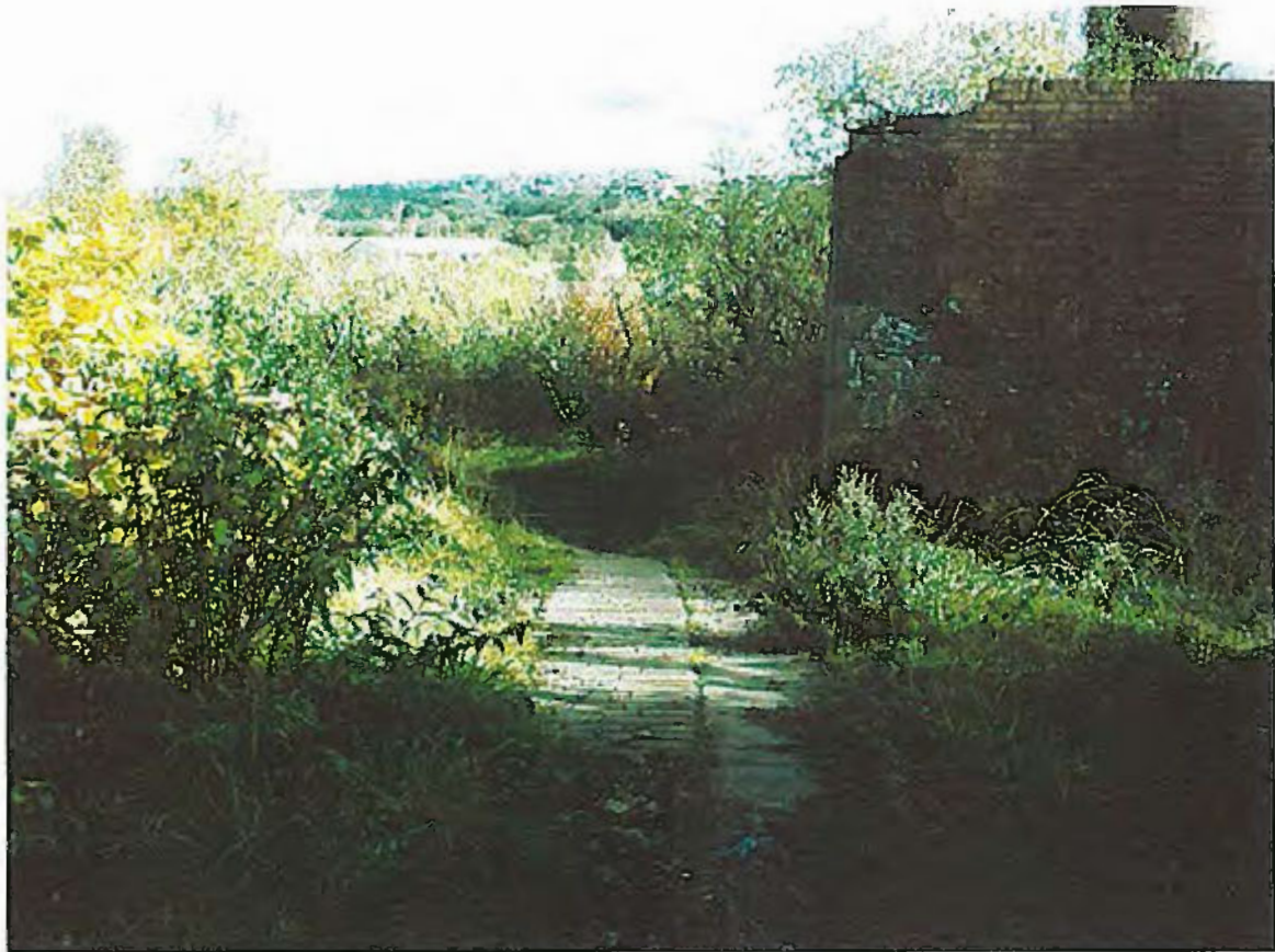
Photo 13 - Area 3A, YIM 38, showing the surviving sett surface from the west
