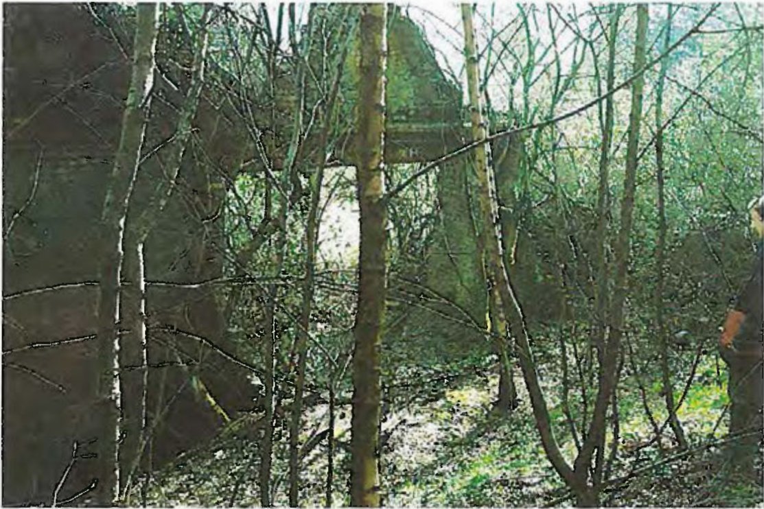
Photo 11b — The south end of Building 11.0 (Vivian Locomotive Shed) from the northwest, showing annexe
