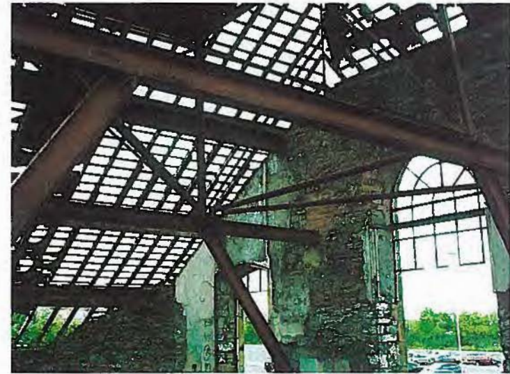
Below right: due to the extensive fire damage to the roof timbers over the western portion of the building, temporary ties are required to give restraint to the iron arch braces and supporting columns.
