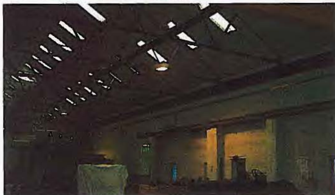
Left lower: internal view of stores, steel angle roof trusses bear onto an eaves beam; brick piers have been built at intervals along the external walls to carry an overhead travelling crane.
