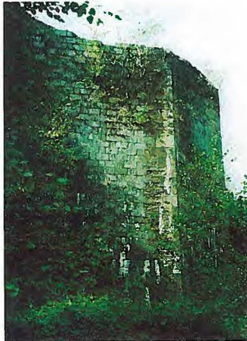
Above: view from south looking up the bed of the former Swansea Canal. The tall, substantial projecting abutment, trapezoidal in plan, is flanked either side by battered walls. Constructed in large copper slag blocks with dressed stone quoins. The abutment formed the western support of the tramroad over the canal.
