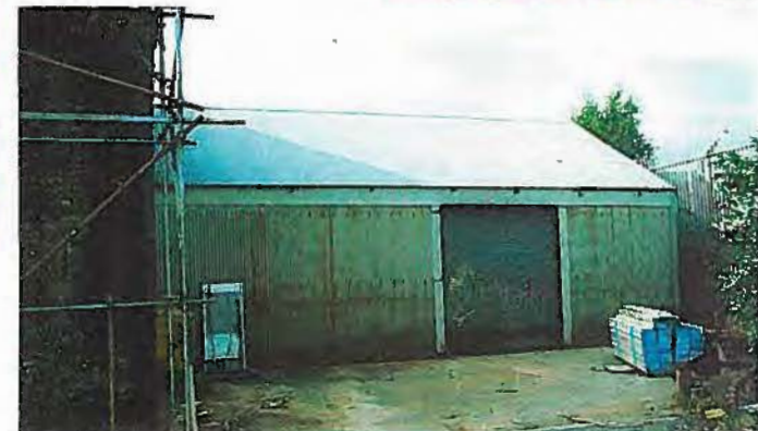
Right lower: modern steel framed profiled metal clad extension at the north end of the museum stores.
