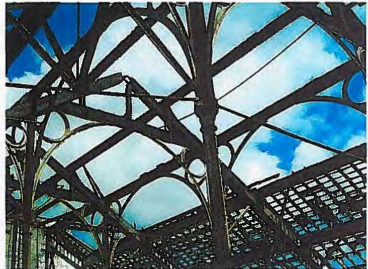
Below right: due to the extensive fire damage to the roof timbers over the western portion of the building, temporary ties are required to give restraint to the iron arch braces and supporting columns.
