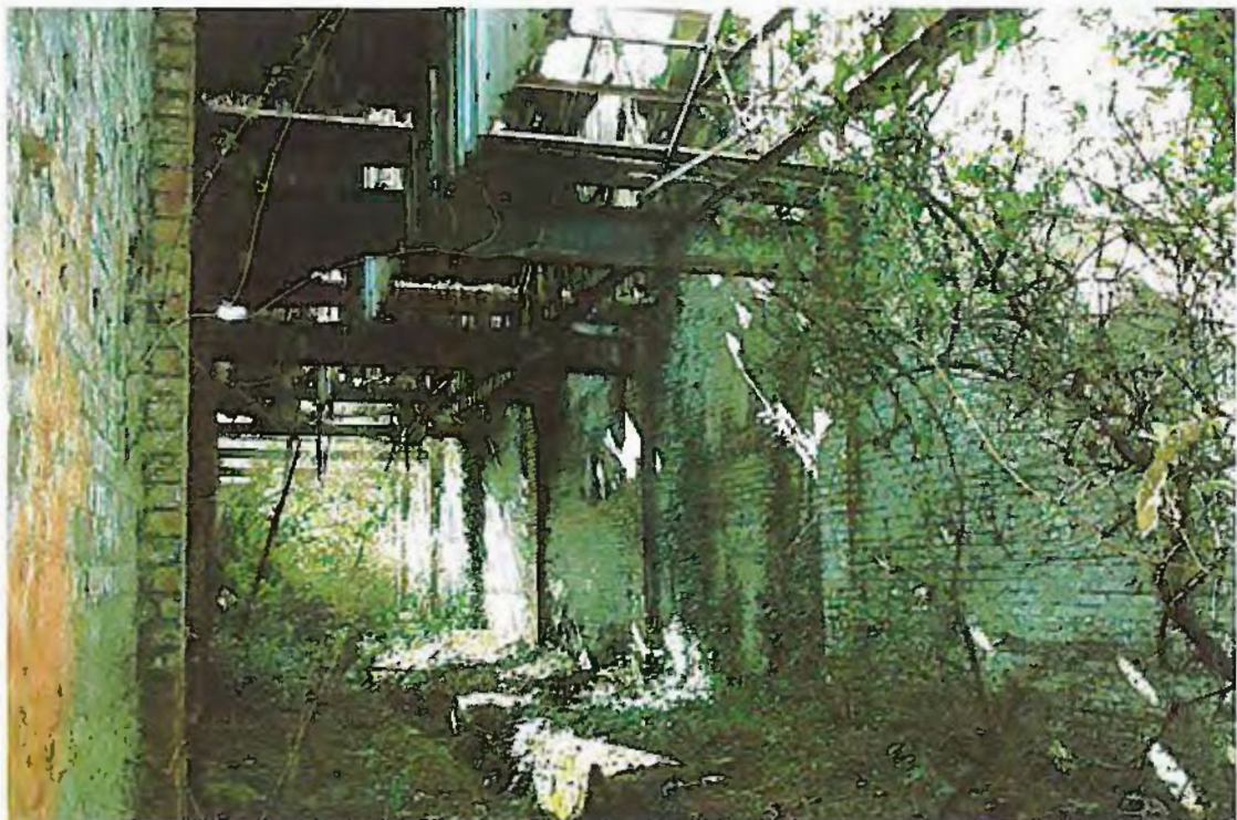
Photo 11c — The interior of Building 11.0 (Vivian Locomotive Shed) from the northeast
