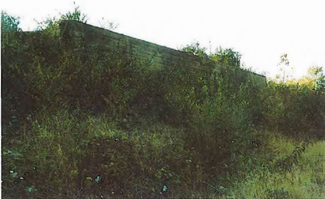
Photo 14d - Area 4, revetment wall YIM 44 from the south
