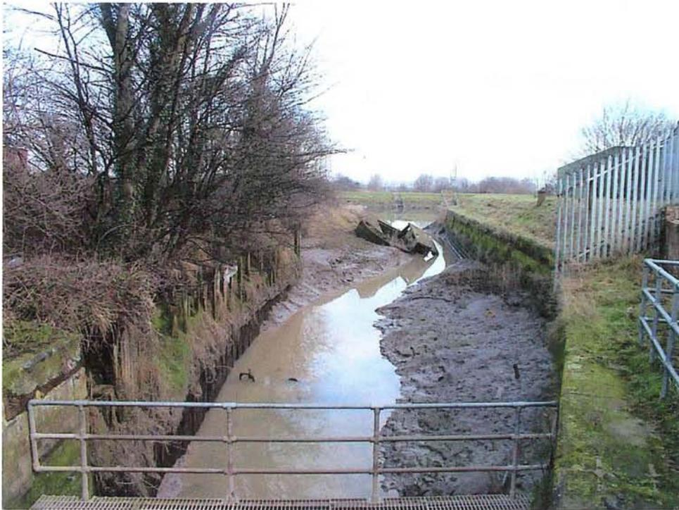
Fig. 52 Sandycroft Quay showing timber revetment on the left and stone revetment on the right.
