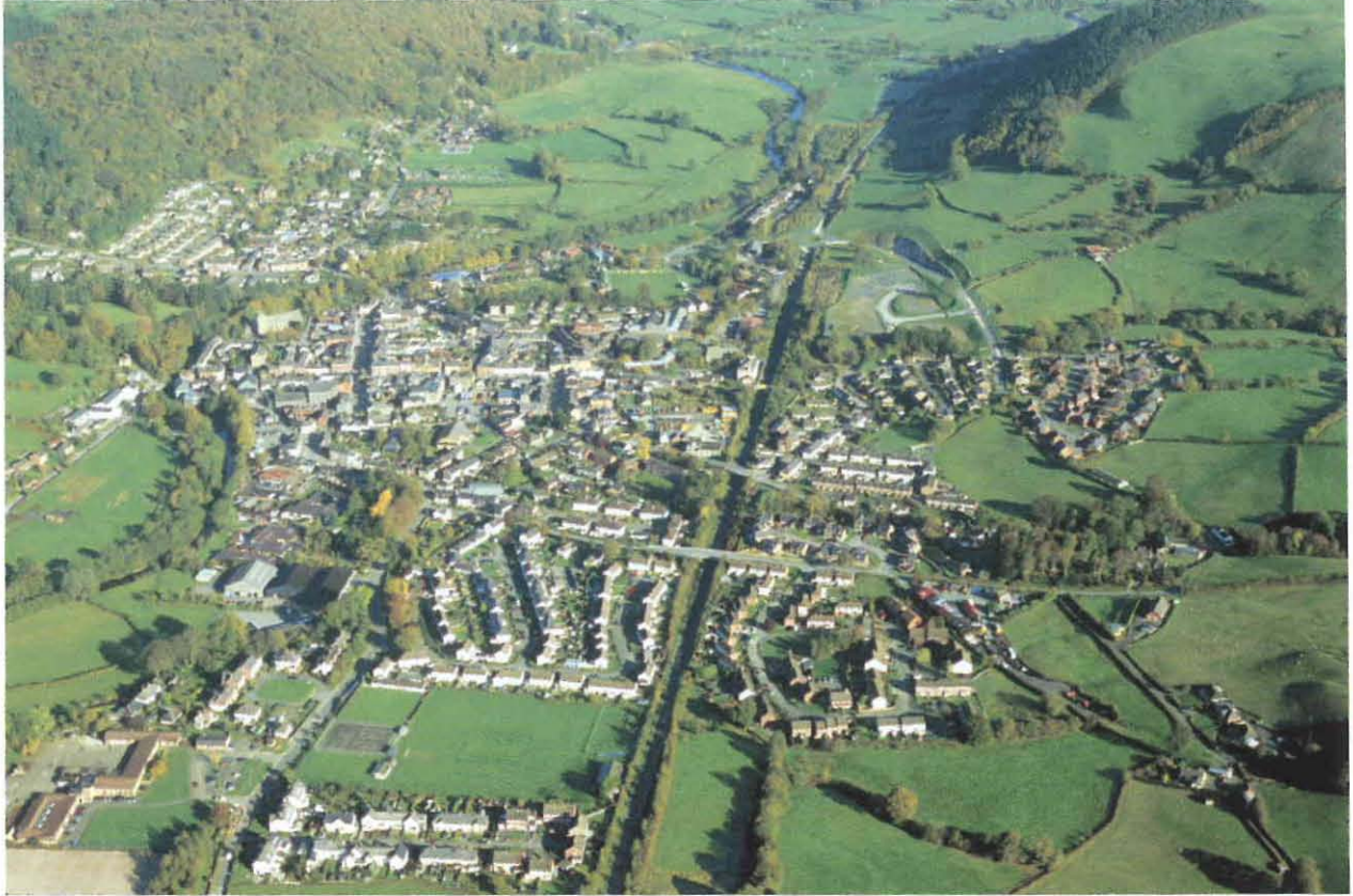
Aerial view of Llanidloes from the south-east with the wooded slopes of Allt Goch to the back left and Gorn Hill to the back right and the Llanidloes bypass, on the course of the former railway down the middle. Photo: CPAT 06-C-131
