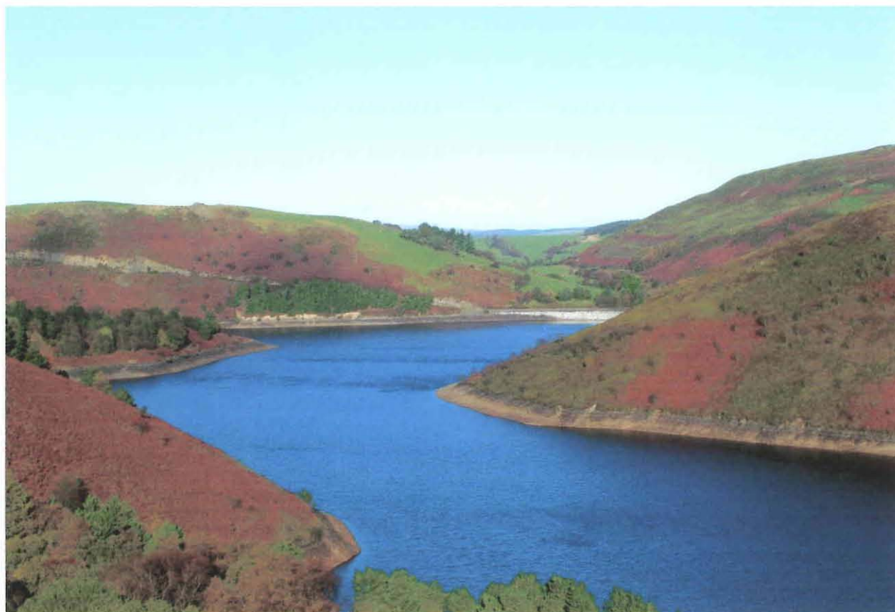
The Clywedog reservoir viewed from near Pen-y-gaer, looking towards the Bwlch-y-gle bridging dam towards the right middle distance. Photo: CPAT 2273-062
