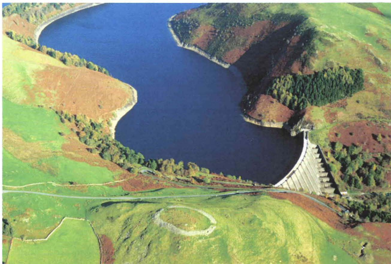
The Clywedog dam and reservoir from the west with the Iron Age defended enclosure of Pen-y-gaer in the foreground. Photo: CPAT 06-C-243
