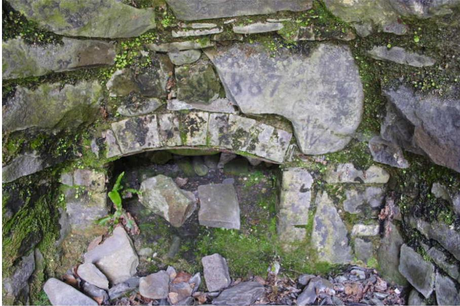
**Photo 53:** Partial dated lintel within southwest draw hole of Llangranog beach limekiln.
