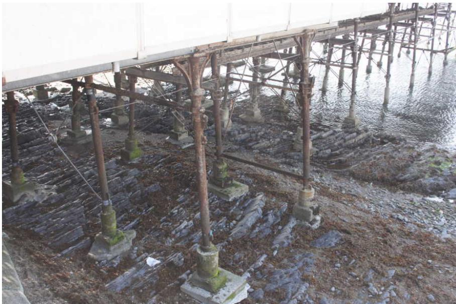
**Photo 19:** Cast iron support pillars of pier with cross tie supports visible to left.
