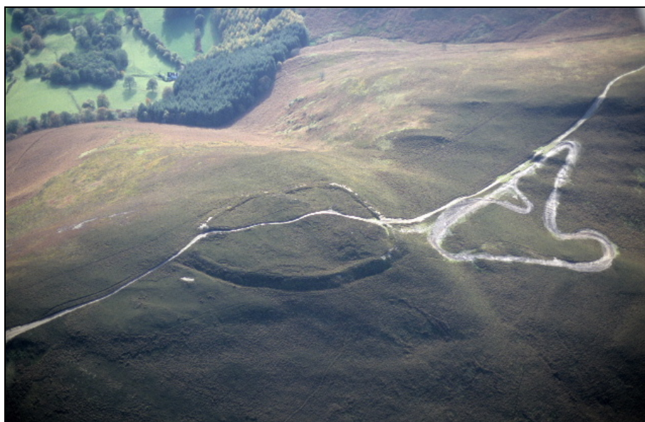
Fig. 1. View of Moel y Gaer from the north-west showing the threat posed by the use of off-road vehicles. Photo CPAT 06-c-0373
