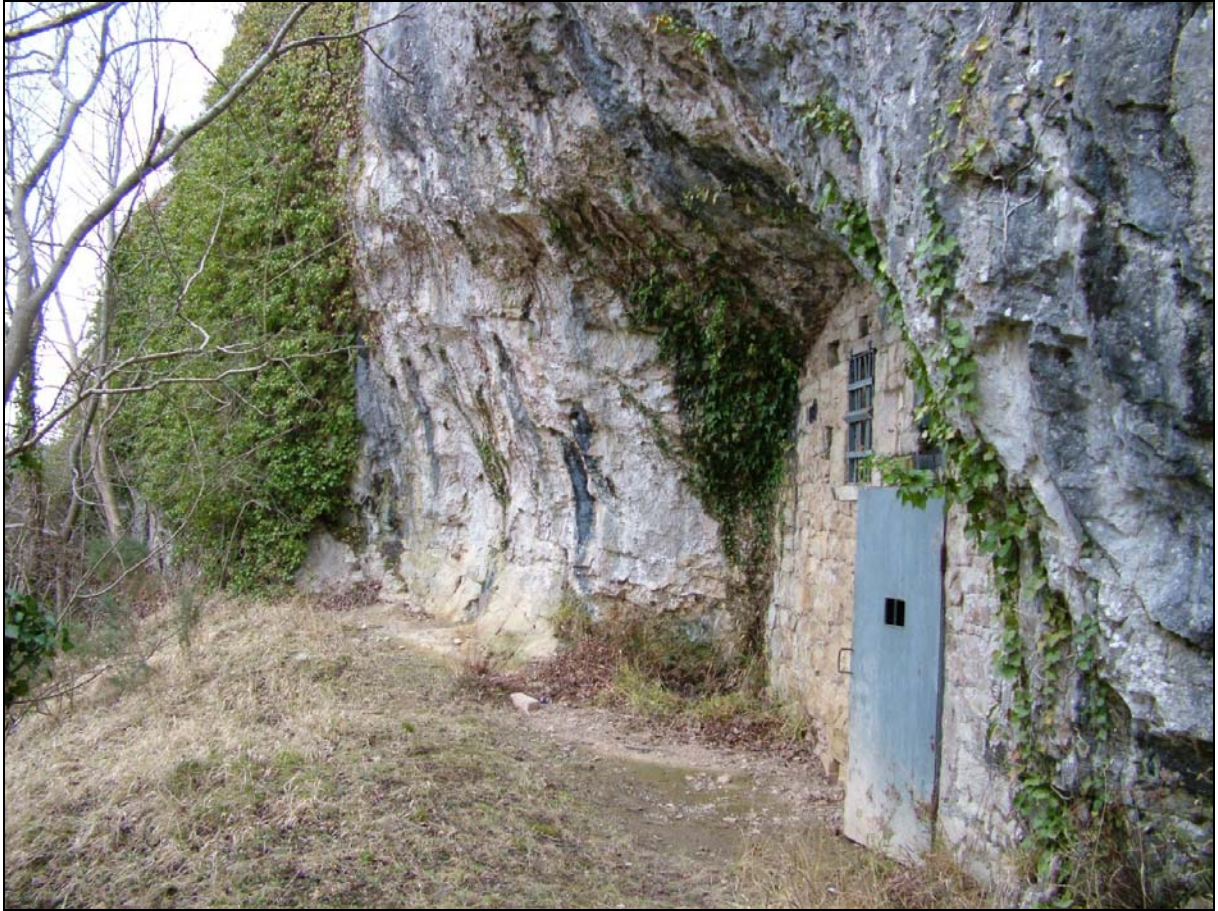
The entrance to Bontnewydd Cave (PRN 102132) showing the walling created when the site was used as an ammunition store in WW2 (Photo CPAT 2784-007)
