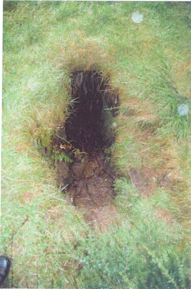
ABOVE: ENTRANCE TO SUBTERRANEAN PASSAGE FROM N
