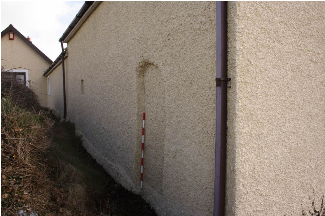
Photo 58: The north wall of Cliff Cottage, showing the blocked arched doorway and small window which may support the idea that the building was formerly a 'fishermen's chapel'.
