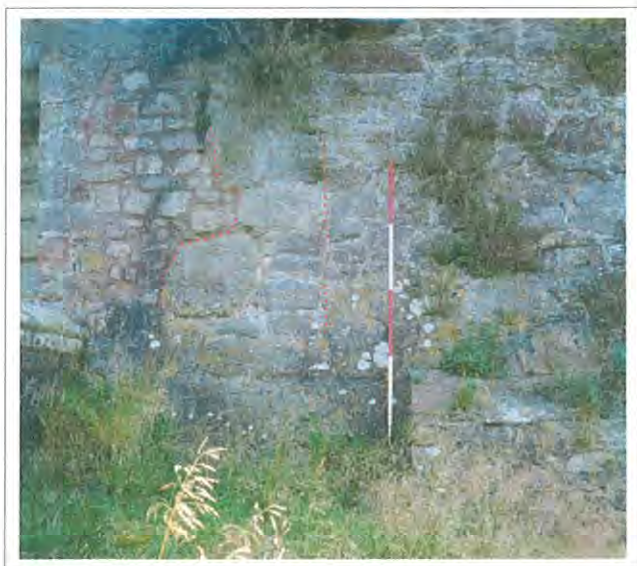
Figure 12 The principal joints in the bowling green wall. Left is the edge of modern disturbance while right is the concealed butt joint
