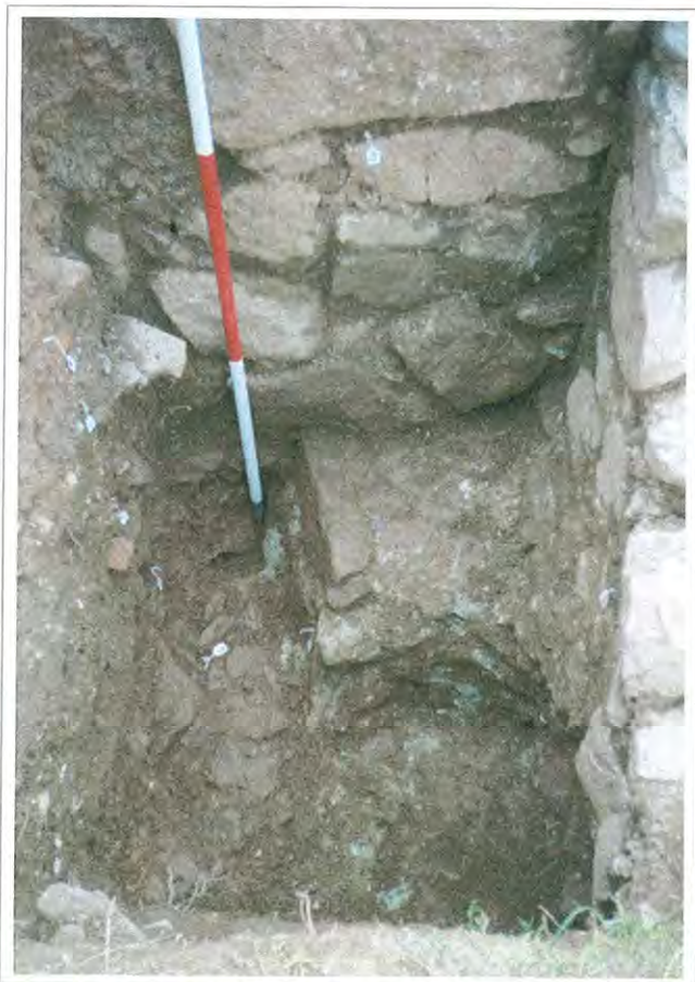
Figure 18 At the top is terrace wall [32] seated on masonry [31] below wall [33] to the right. Rubble [30] is just appearing in the base of the trench
