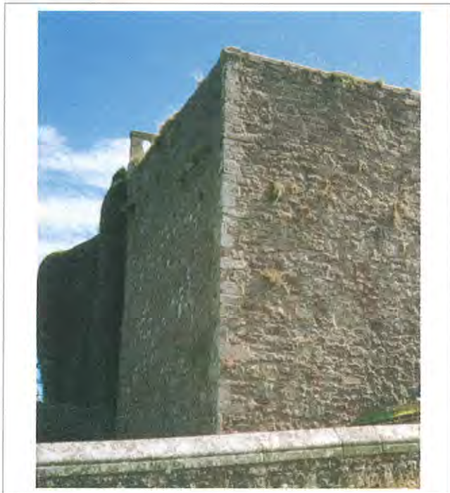
Figure 13 The rubble masonry and quoins of the extended High Terrace
