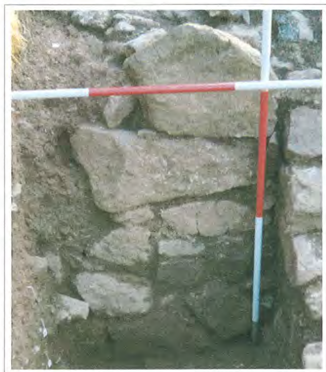
Figure 20 The full surviving height of terrace wall [32], showing the coarse masonry, damaged to the left during demolition. The butt joint against the stair wall [33] to the right is clear. The wall was probably only a little higher when built
