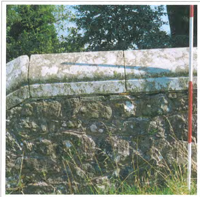
Figure 14 The masonry of the North wall of the stairs. Note that the coping has hardly eroded
